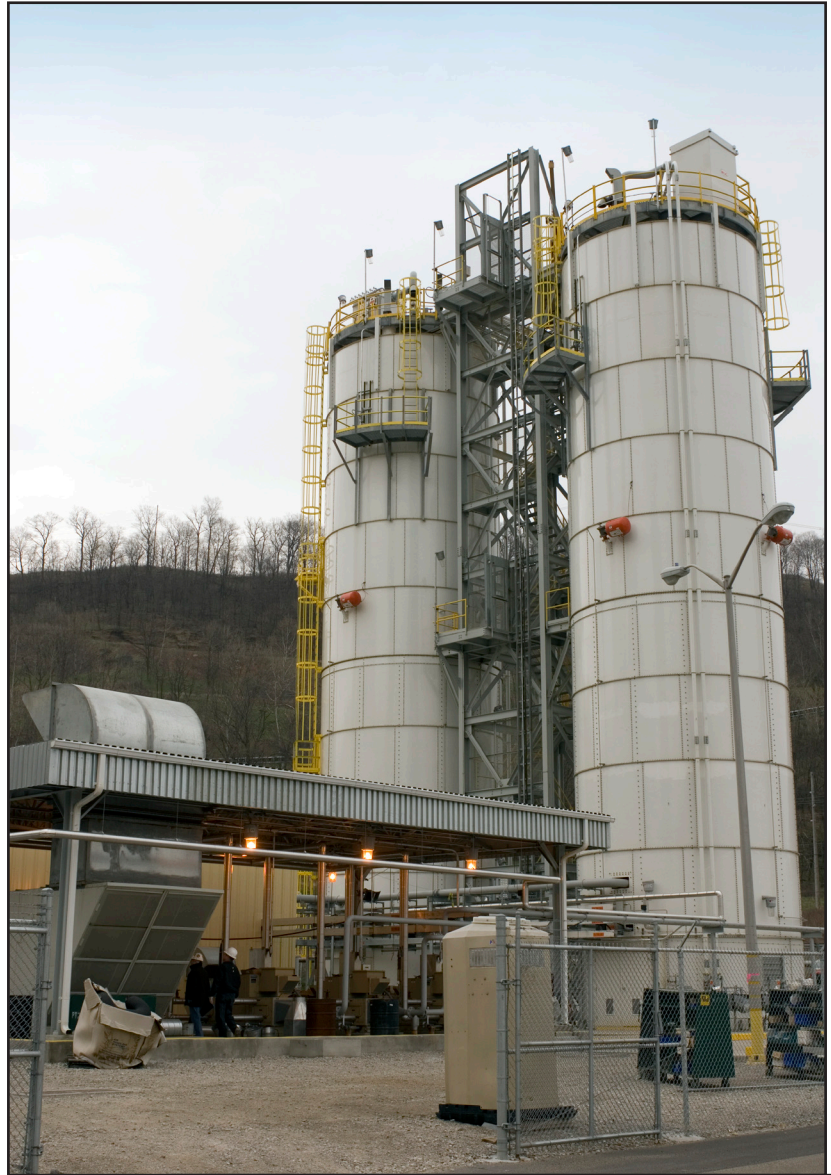
Truck unloading and conditioning station for trona system.
