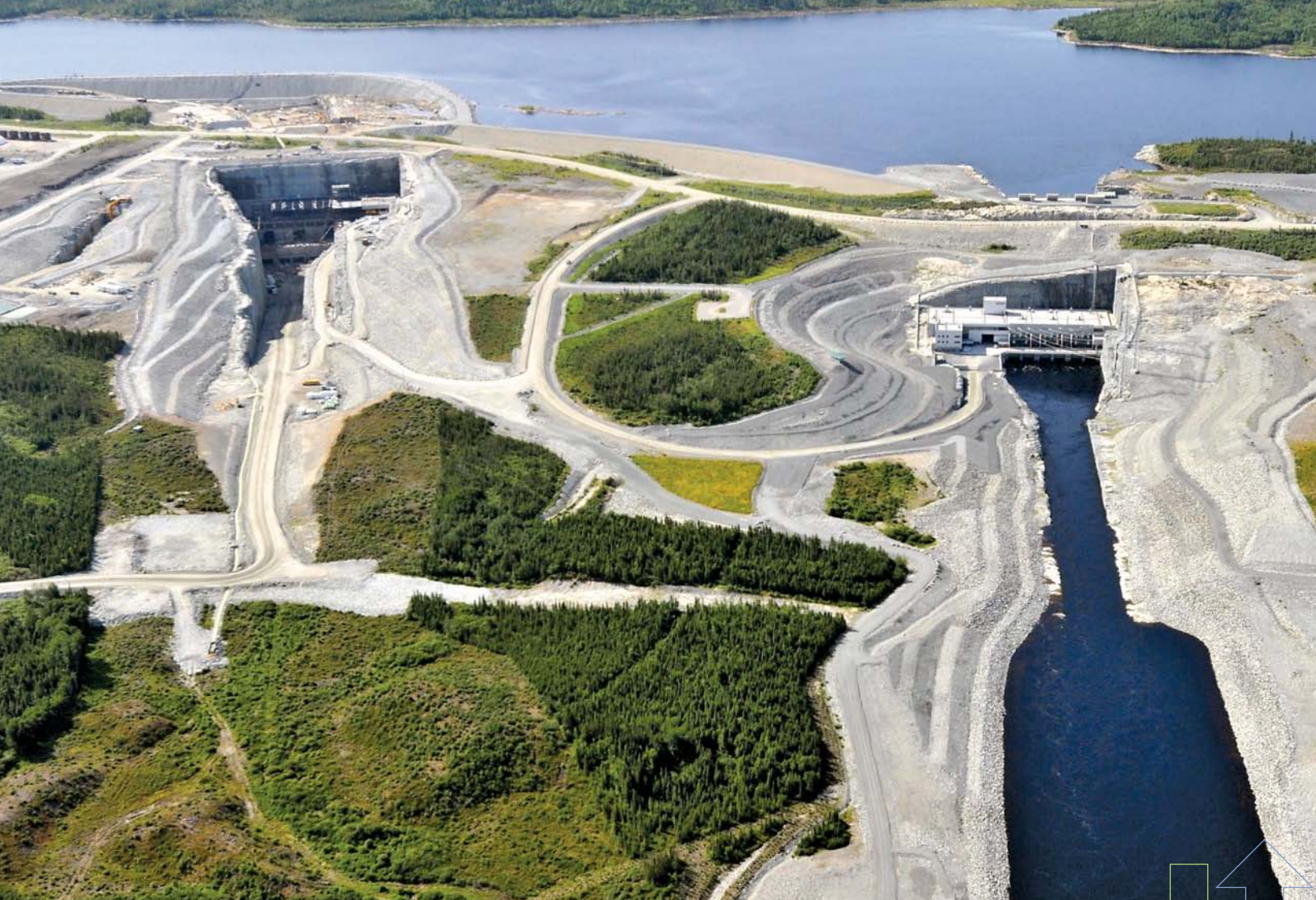
Eastmain-1 powerhouse and Eastmain-1-A construction site
