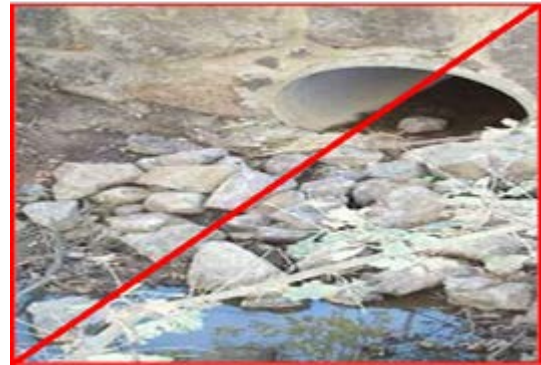
Figure 12-35 – Incorrect Construction of Rock Energy Dissipaters
