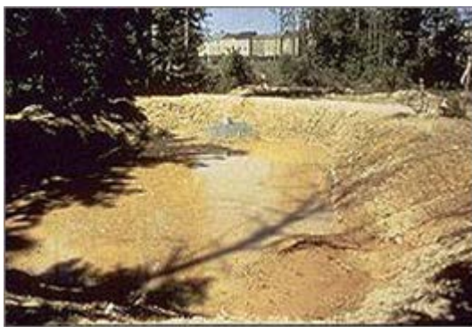
Figure 12-41 – Sediment Basin
