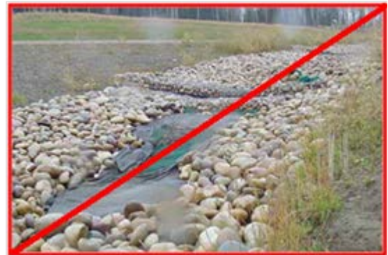
Figure 12-31 – Photograph of Failed Rip Rap Protection
