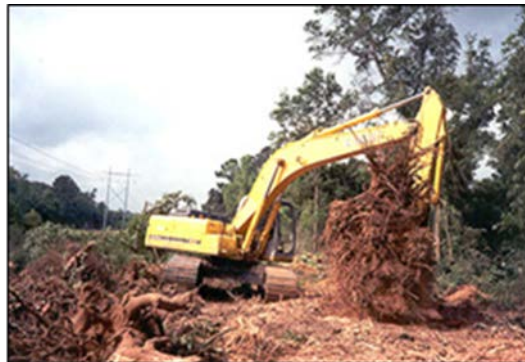
Figure 12-18 – Example of a Grubbed and Cleared Path
