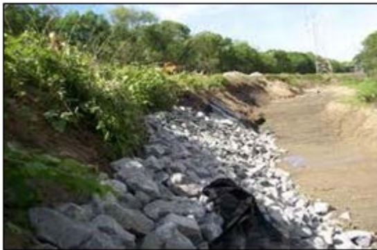
Figure 12-30 – Photograph of Rip Rap Placed Along a Slope
