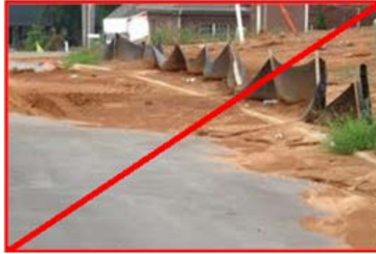
Figure 12-40 – Example of Poorly Installed Silt Fences
