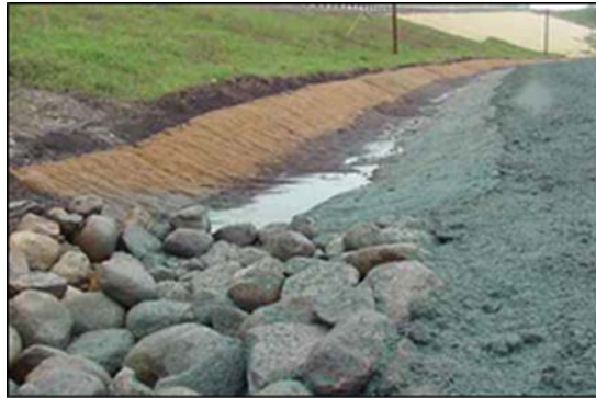
Figure 12-29 - Photograph Shows Erosion Control Blanket on Slope and Erosion Control Mat in Channel
