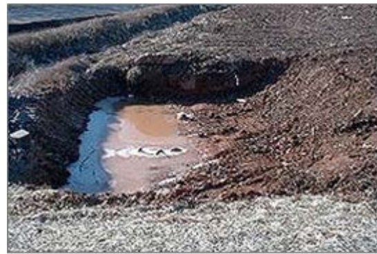
Figure 12-42 – Sediment Trap
