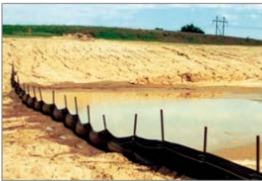
Figure 12-36 – Well Constructed Silt Fence
