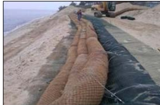
Figure 12-28 – Photograph of Fibre Rolls Used to
