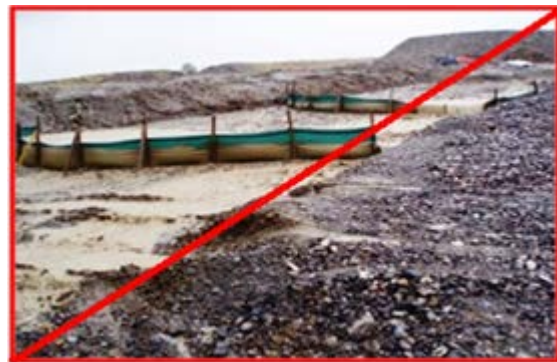
Figure 12-39 – Example of Poorly Installed Silt Fences
