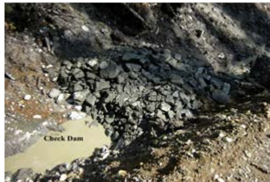
Figure 12-33 – Photograph of a Rock Constructed Check Dam
