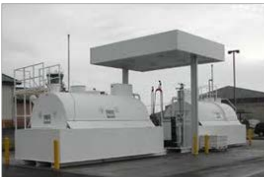
Figure 12-10 – Acceptable Fuel Storage with Dykes
