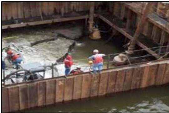
Figure 12-15 – Cofferdams Surrounding Work Area
