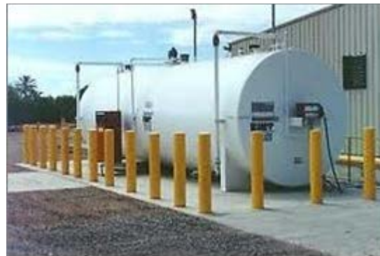
Figure 12-11 – Fuel Storage on Concrete pad
