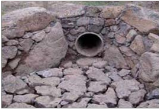
Figure 12-34 – Correct Construction of Rock Energy Dissipaters
