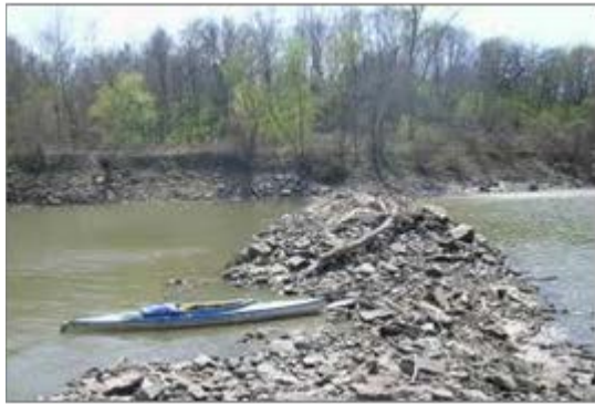
Figure 12-32 – Photograph of a Rock Constructed Dyke
