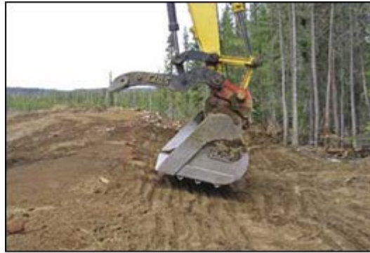
Figure 12-24 - Photograph of Grooving Slope Treatment Method
