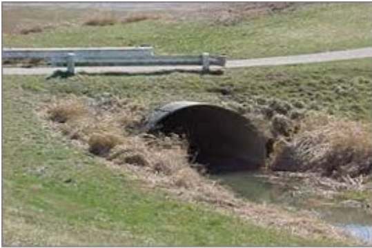
Figure 12-12 – Example of a Well Installed Culvert
