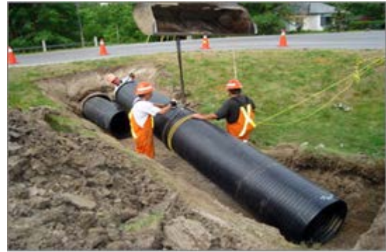
Figure 12-13 – Example of Culvert Installation
