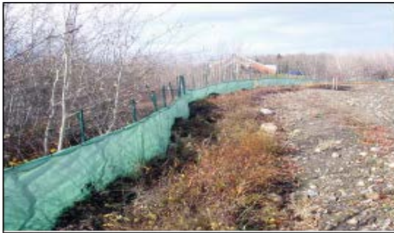
Figure 12-14– Tarp Fence Outlining a Vegetation Buffer Zone
