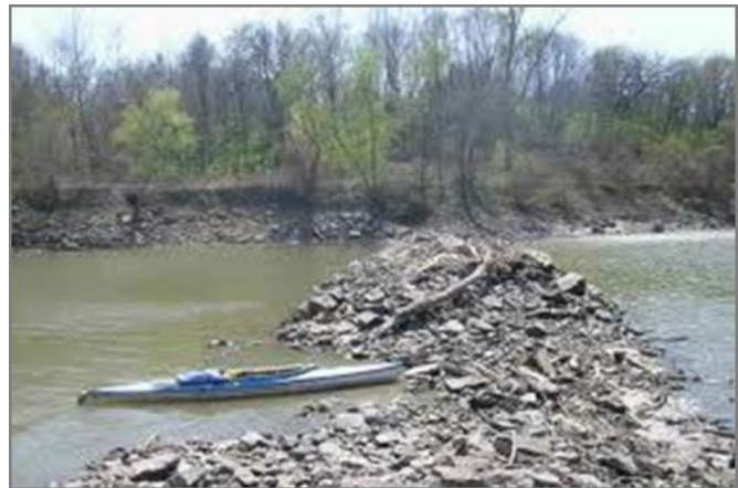
Figure 11-30 - Photograph of a Rock Constructed Dike
