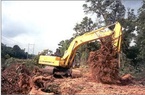
Figure 11-13 - Example of Grubbing Activities
