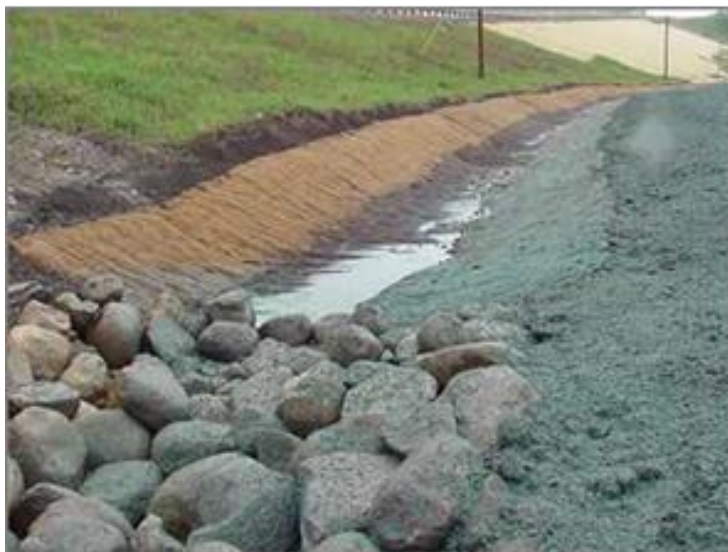
Figure 11-25 - Photograph of Fibre Rolls used to Stabilize
