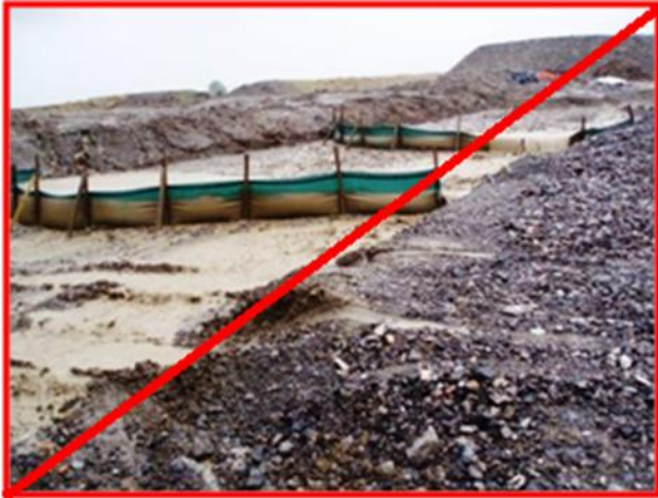
Figure 11-36 - Examples of Poorly Installed Silt Fences
