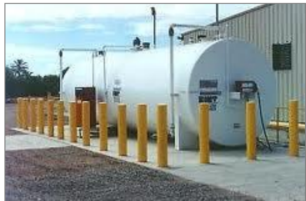
Figure 11-7 - Fuel Storage on Concrete Pad
