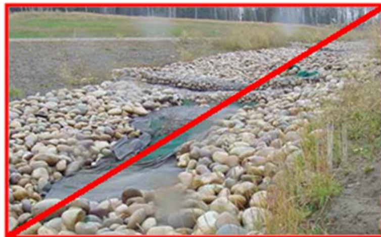
Figure 11-28 - Photograph of failed Rip Rap Protection a Slope
