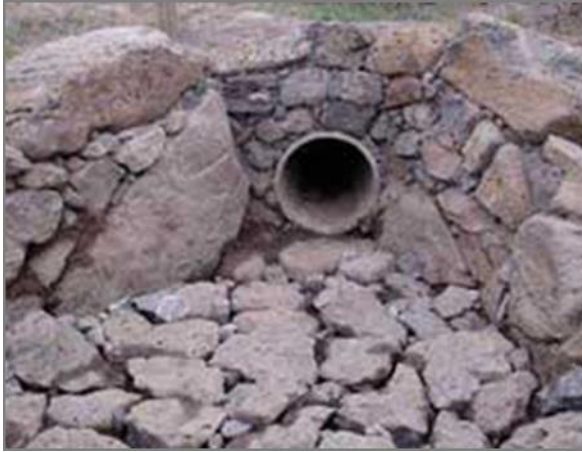
Figure 11-31 - Correct Construction of Rock Energy Dissipaters
