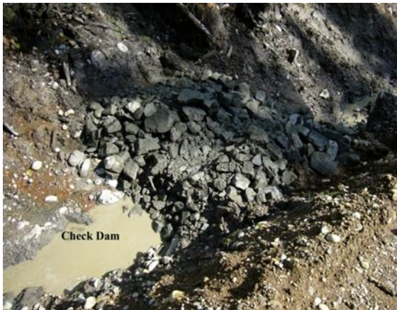
Figure 11-29 - Photograph of Rock Constructed Check Dam
