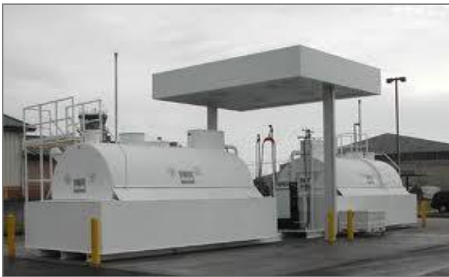
Figure 11-6 - Acceptable Fuel Storage with Dykes
