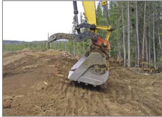
Figure 11-21 - Photograph of Grooving Slope Treatment Method
