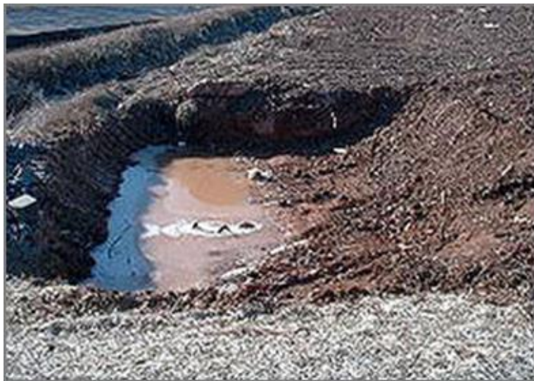
Figure 11-39 - Sediment Trap
