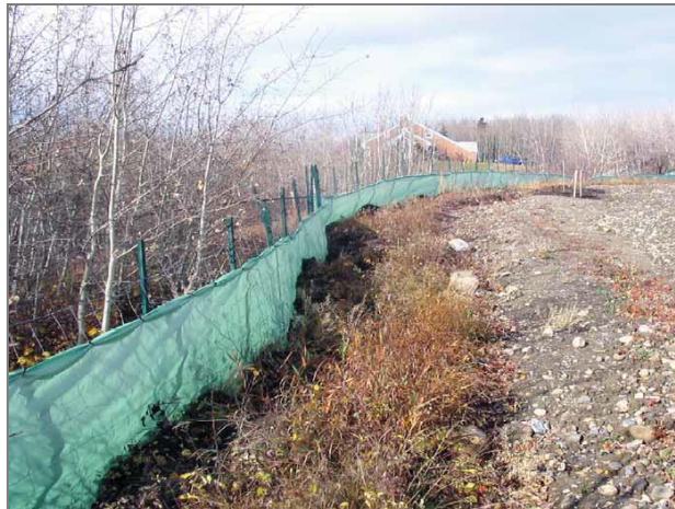
Figure 11-10 - Tarp Fence Outlining a Vegetation Buffer Zone
