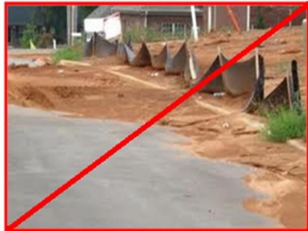
Figure 11-37 - Examples of Poorly Installed Silt Fences
