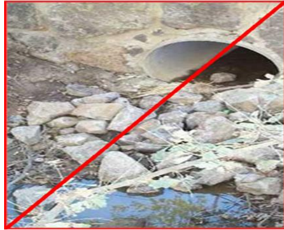
Figure 11-32 - Incorrect Construction of Rock Energy Dissipaters
