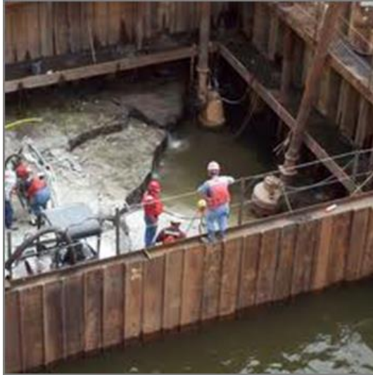
Figure 11-11 - Cofferdams Surrounding Work Area
