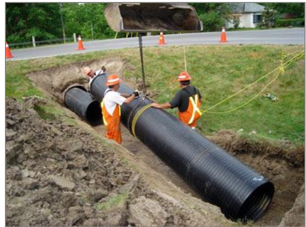
Figure 11-9 - Example of Culvert Installation
