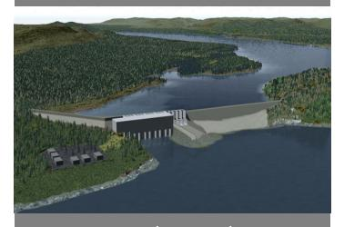
824 MW/ 5 TW-h/yr Reservoir length - 60 km Flood area – 41 sq km
