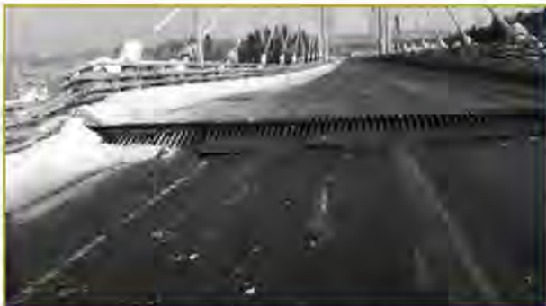
Figure 10: Nipigon River Bridge After It Malfunctioned
