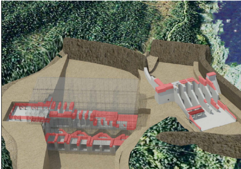
Figure 8: Astaldi as-planned status of the civil structures by October 2014 – CH0007 Construction visualization with Astaldi bid (downstream view). Note the intended concrete placement in the various structures, but in particular Intake unit 1 located towards the left background in the above photo.
