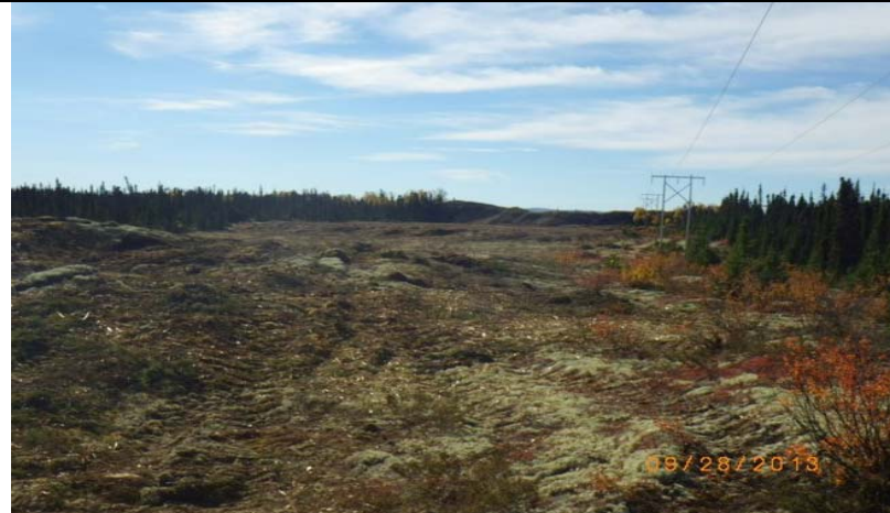
CT0341: RoW Clearing HVac 315kV TL – Clearing works.
