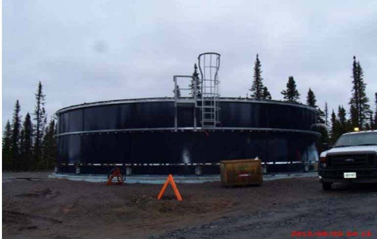
CH0002: Accommodation complex – Water Treatment Plant - installation works
