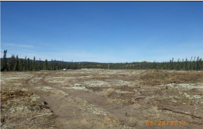
CT0341: RoW Clearing HVac 315kV TL – Clearing works.
