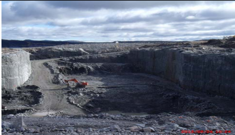
CH0006: Bulk Excavation – Powerhouse excavation works
