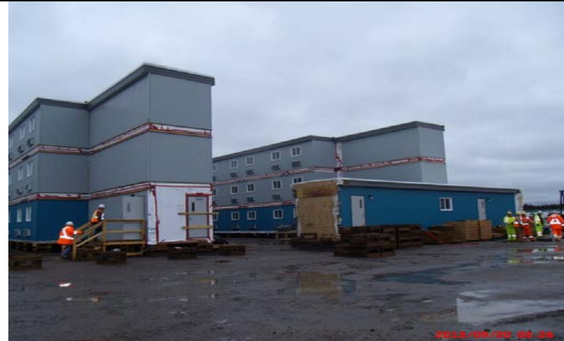
CH0002: Accommodation complex – Dorms - Installation works.
