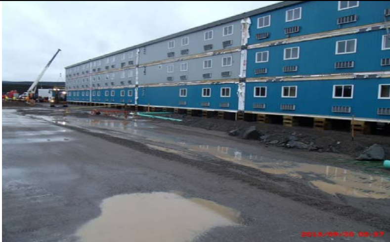
CH0002: Accommodation complex – Dorms - installation works
