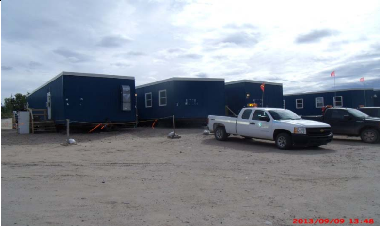
CH0024: Reservoir Clearing – Camp installation works.
