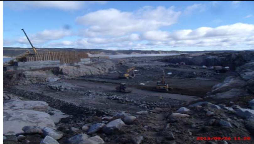
CH0006: Bulk Excavation – Spillway excavation works
