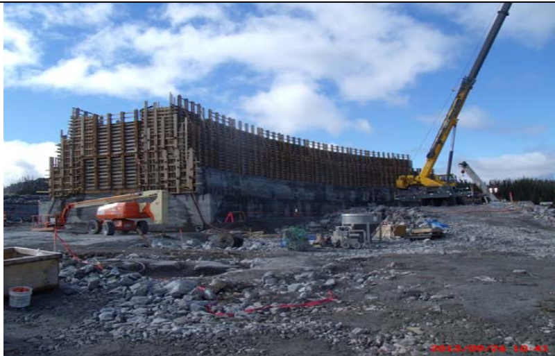
CH0006: Bulk Excavation – River side RCC Cofferdam construction works
