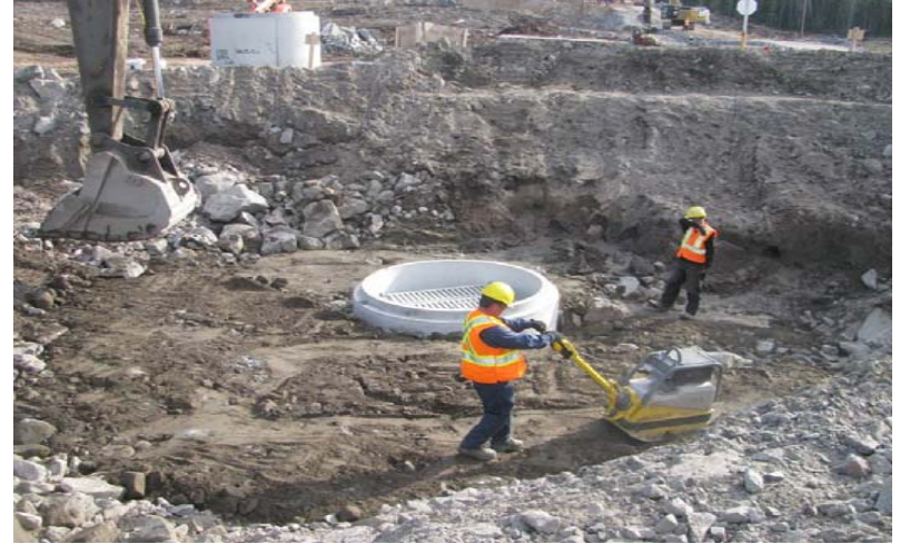
CH0002: Accommodation complex – Sewage Plant - Construction works.
