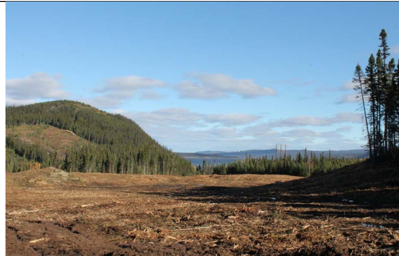
CH0024: Reservoir Clearing – South side clearing works.
