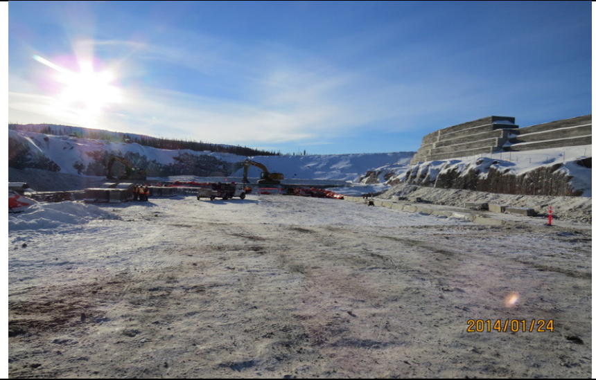
CH0007: Spillway concrete foundation base temporary structure
