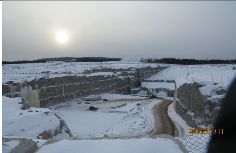
CH0007: Powerhouse-mobilization and dewatering activities
