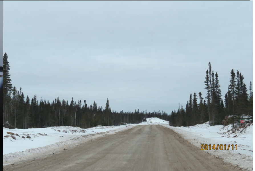
CH0004-1: Caroline Brook Resource Road Upgrade-complete at KM1
