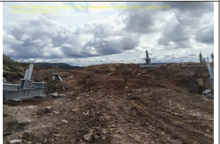
CT0319: Construction of HVac Transmission Line-Self-supporting structure foundations ready for concrete
