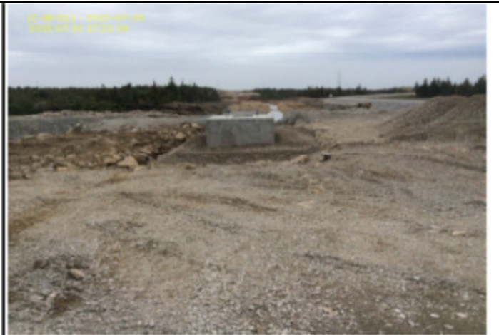
SOBI: Cable vault foundations completed with backfill at Shoal Cove
