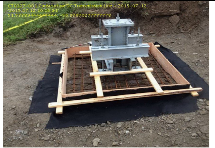
CT0327-001: HVdc Transmission Line—Rock foundation formwork ready for concrete placement
