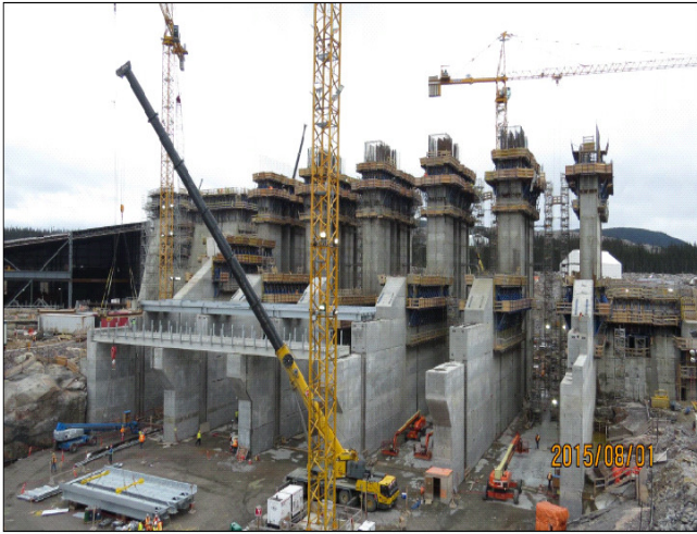
CH0007: Spillway-as seen from Cofferdam 2
