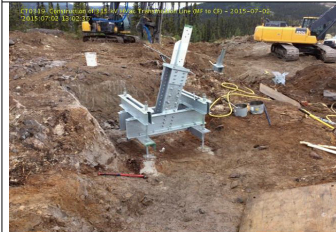
CT0319: Construction of HVac Transmission Line-Formwork construction of concrete installation
