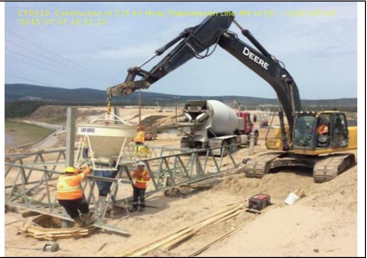
CT0319: Construction of HVac Transmission Line-Placing concrete at structure L1-10
