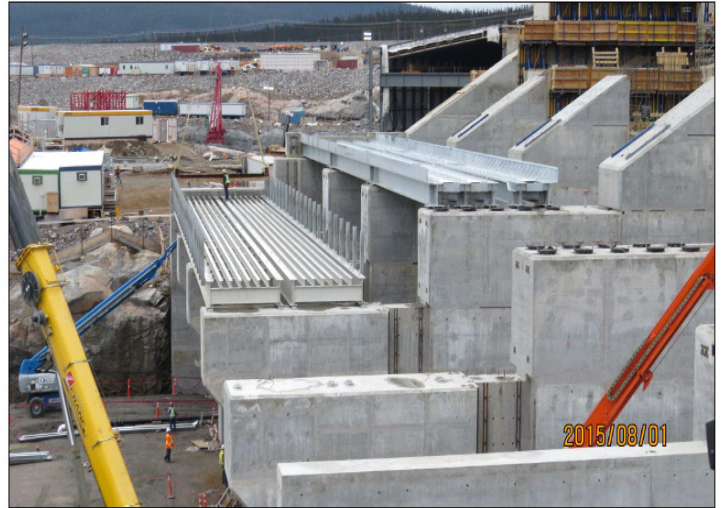
CH0007: Downstream temporary/permanent spillway bridges
