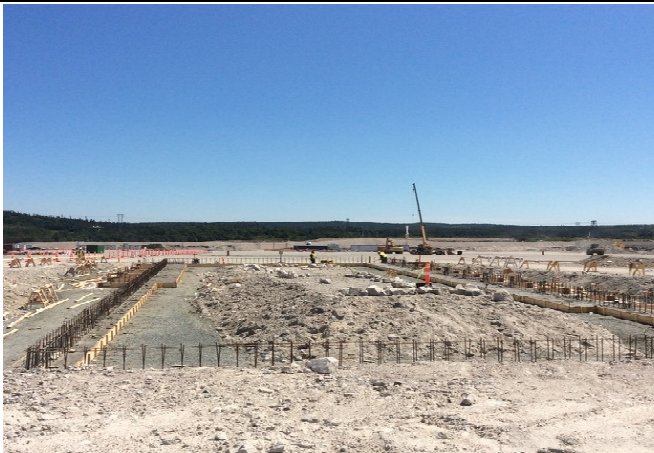
CD0504: HVdc Specialties Civil Works and Building Services-Control Building foundations
