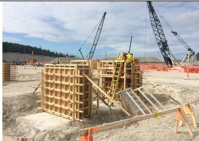
CD0534: Supply and Install Soldiers Pond Synchronous-Formwork
