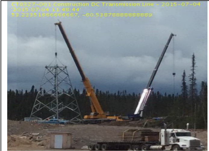
CT0327-001: HVdc Transmission Line—Erecting of self-supporting structure of tower S1-45
