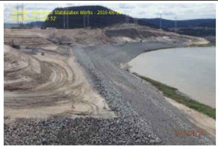
CH0008: North Spur Stabilization Works
