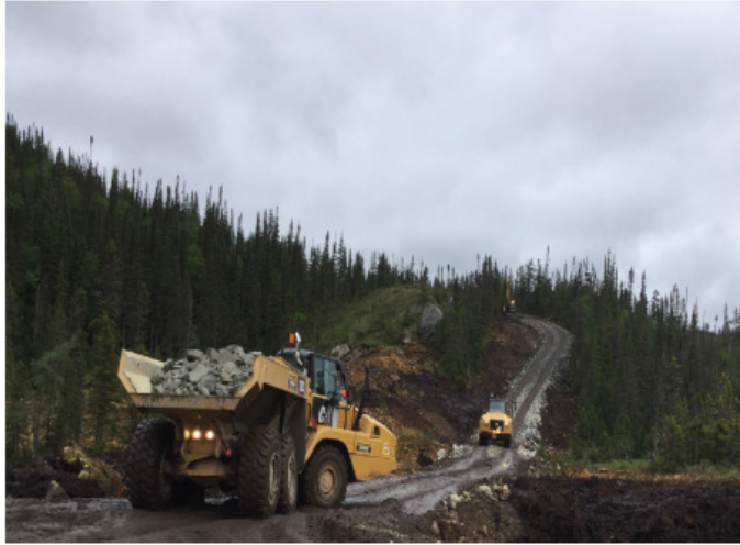
CT0327-001: HVdc Transmission Line-Clearing/Access-LRM
