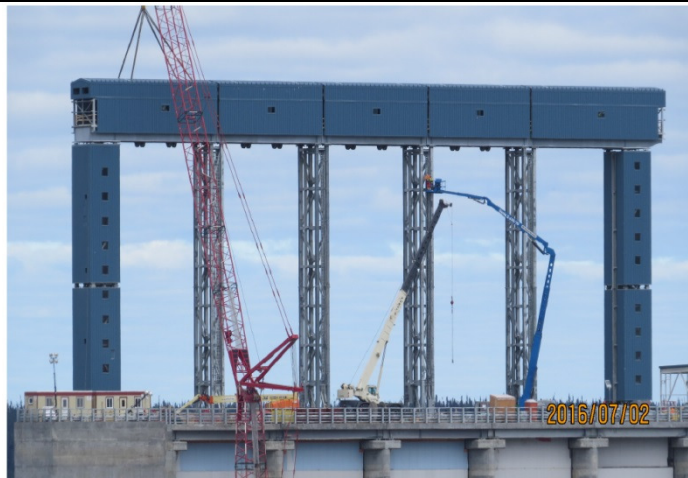
CH0007: Completing spillway structure
