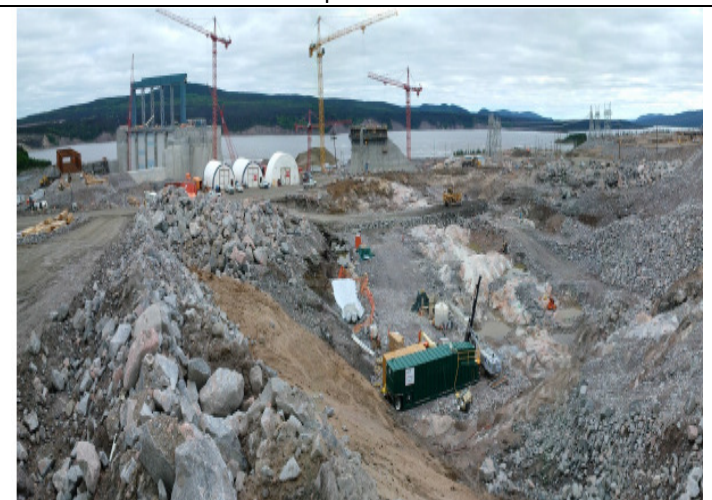
CH0009: South Dam Construction
