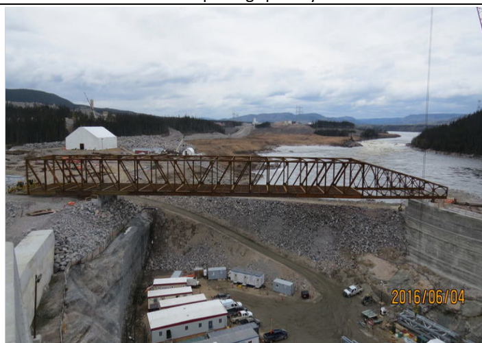
CH0009: Temporary Spillway Bridge
