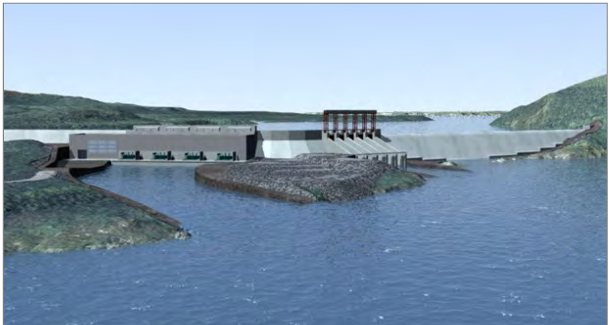
Figure 2-1: Muskrat Falls Generating Facility (Component 1)
