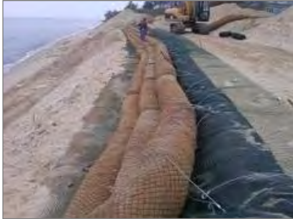
Figure 5-25: Photograph of Fibre Rolls used to stabilize
