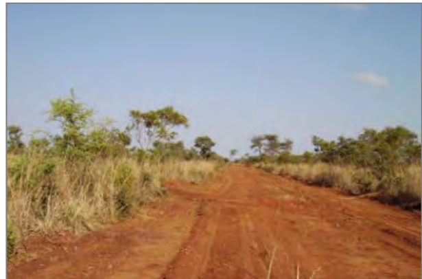
Figure 5-14: Example of grubbed and cleared path
