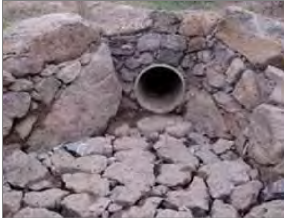
Figure 5-31: Correct Construction of Rock Energy Dissipaters
