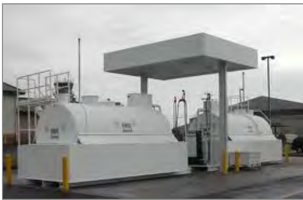
Figure 5-5: Acceptable fuel storage with dykes
