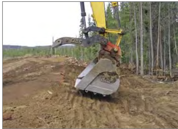
Figure 5-21: Photograph of grooving slope treatment method
