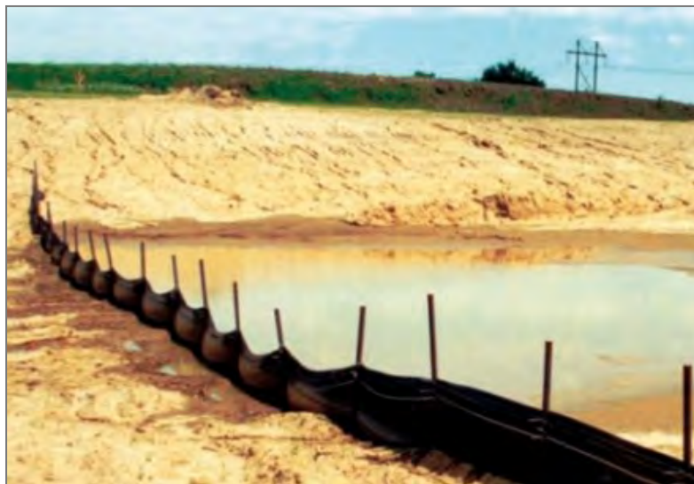
Figure 5-33: A well constructed silt fence
