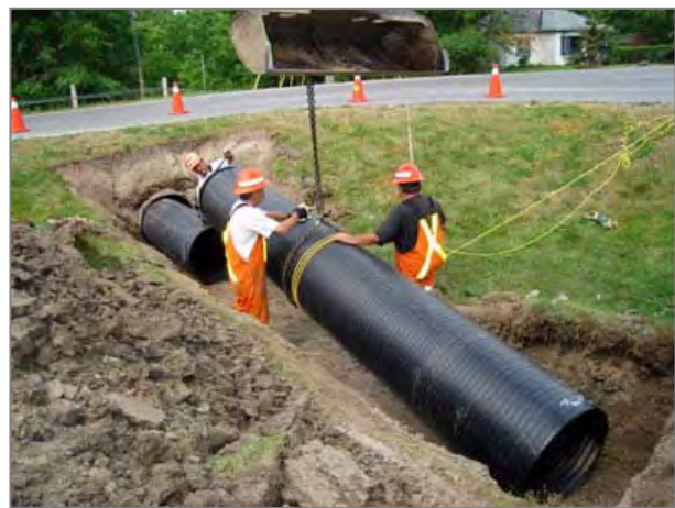
Figure 5-8: Example of culvert installation
