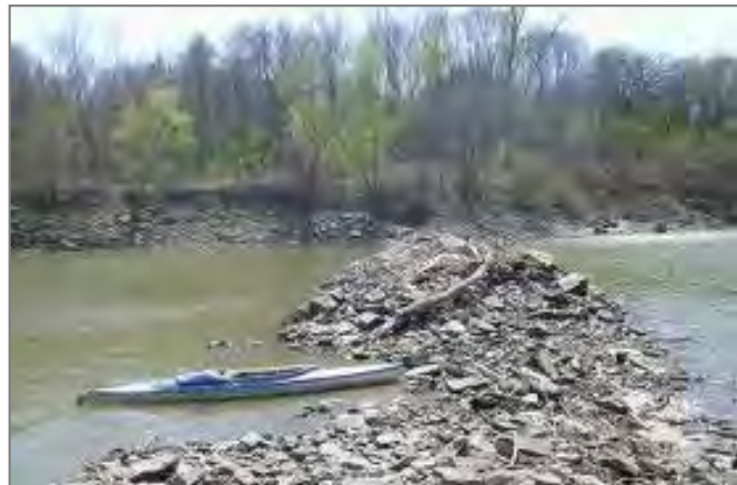
Figure 5-30: Photograph of a Rock Constructed Dike
