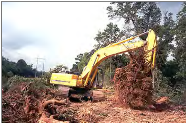
Figure 5-13: Example of grubbing activities
