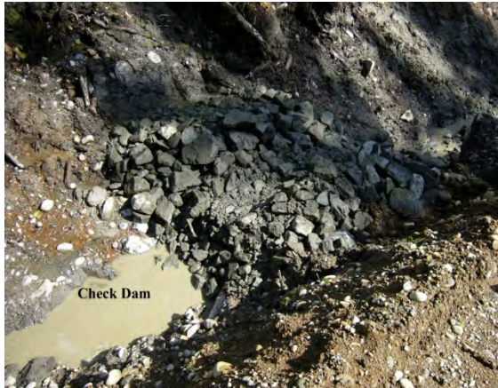
Figure 5-29: Photograph of Rock Constructed Check Dam
