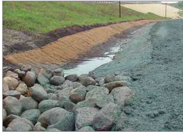
Figure 5-26: Photograph shows erosion control blanket on slope and erosion control mat in channel
