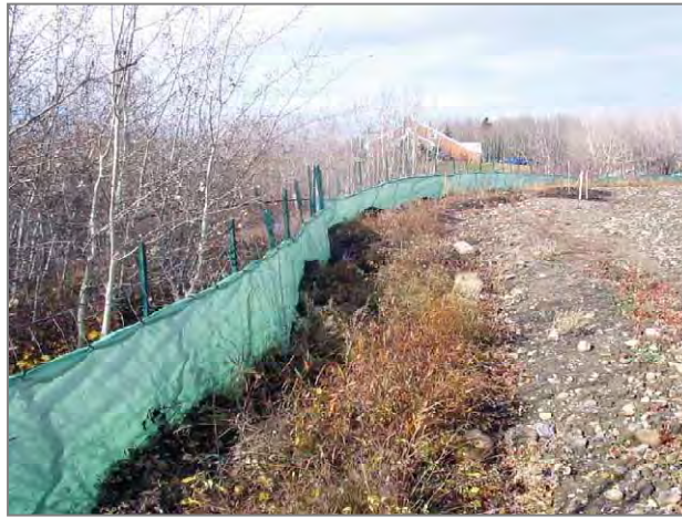
Figure 5-9: Tarp fence outlining a vegetation buffer zone
