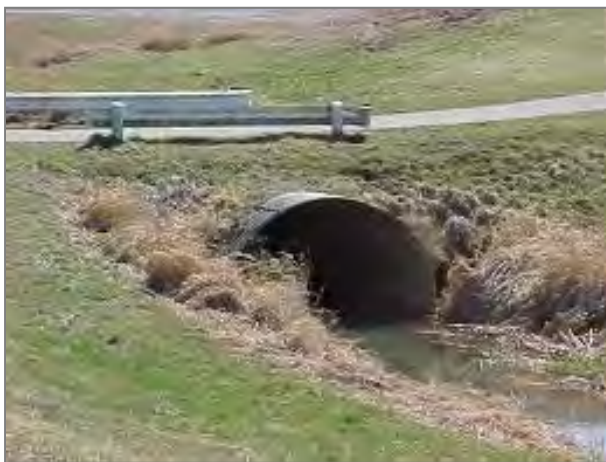
Figure 5-7: Example of well installed culvert
