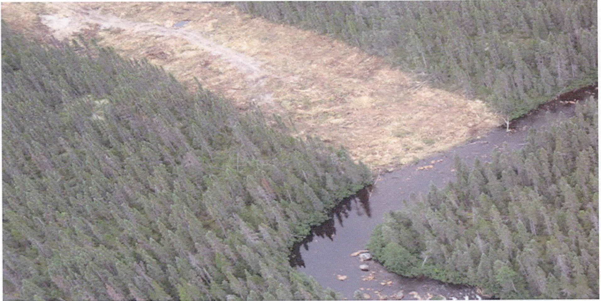
Station 14+100_ C13 Crossing_23-Aug-12
