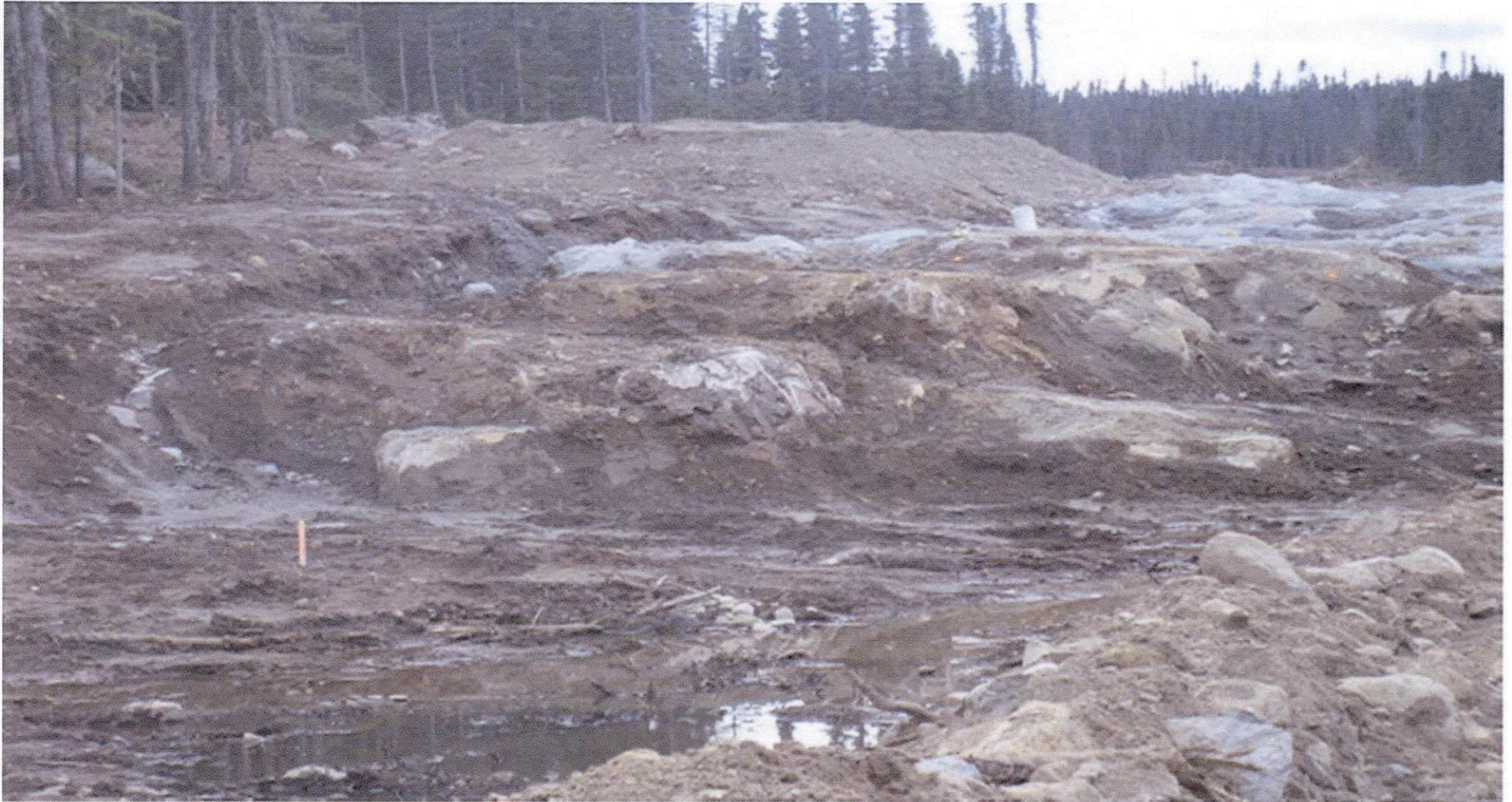
SSAR_ Preparation for Blasting on ROW_ 24-Aug-1
