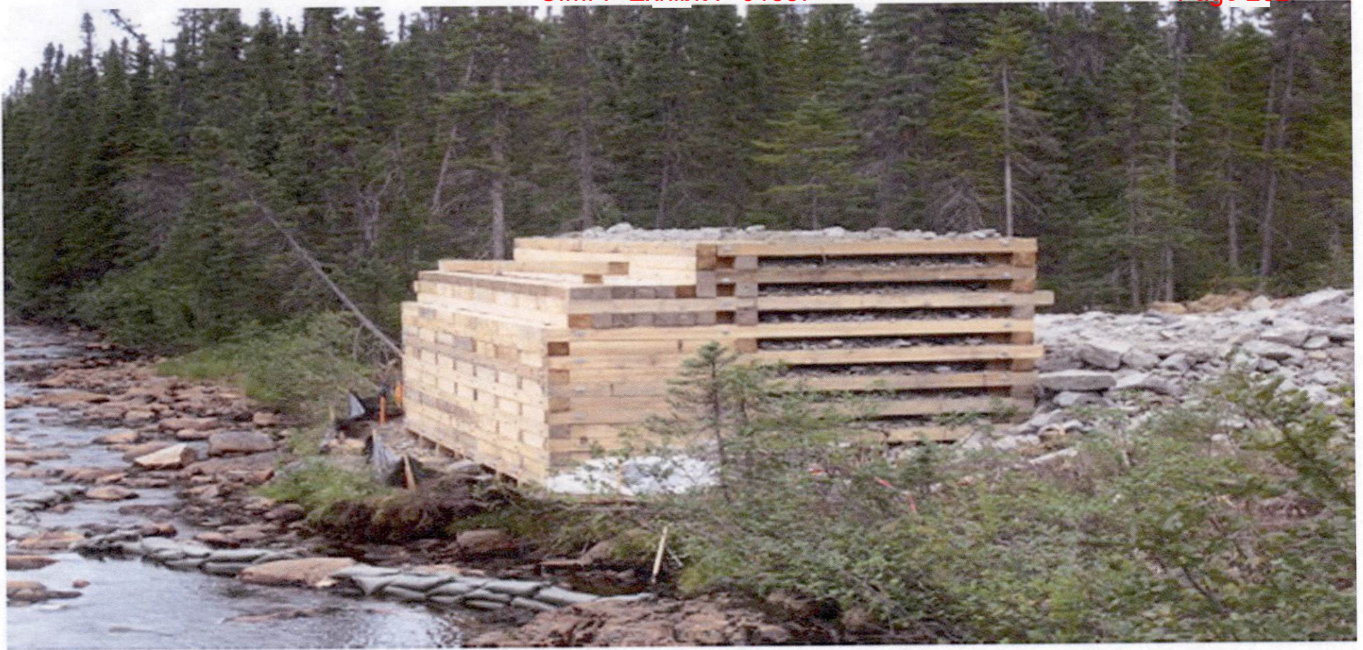
C7 Caroline Brook East side Abutment Completed 26-Aug-12
