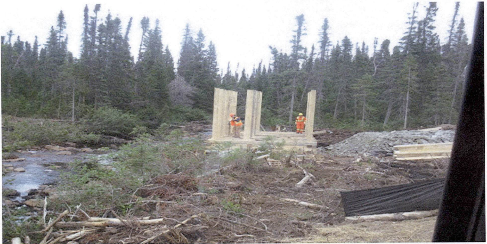
SSAR_ Preparation of Cribbing at C7 Caroline Brook_ 24-Aug-12
