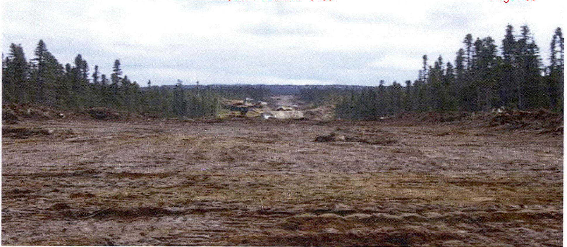
Road Construction Activity Looking East From 13+800
