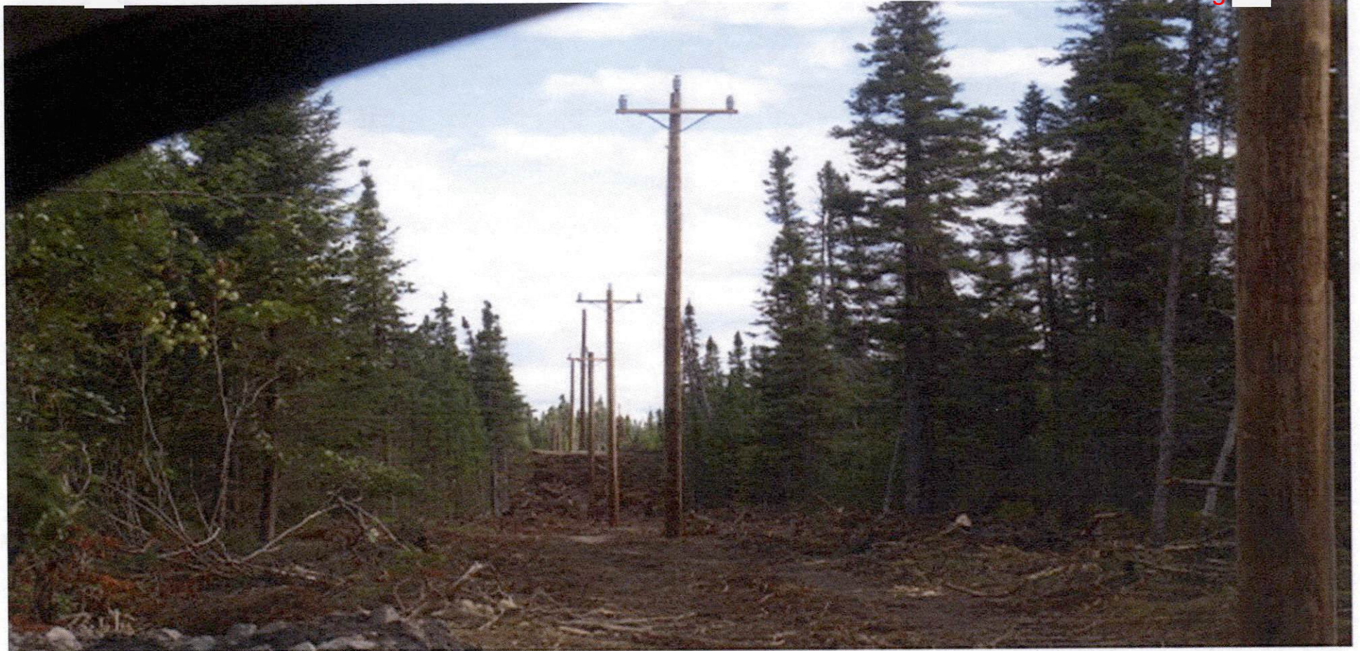
Construction Power_ Pole line Southside of Public Access Road_24-Aug-12
