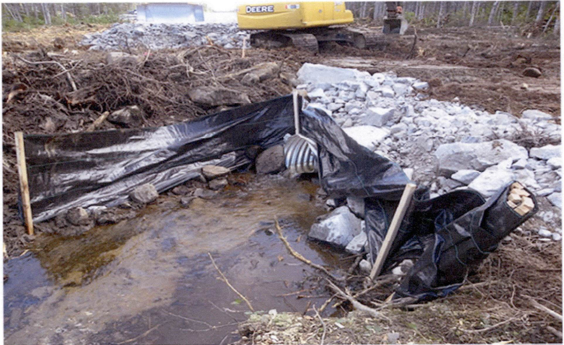
Installed Temporary Culvert At C10 (10+572)
