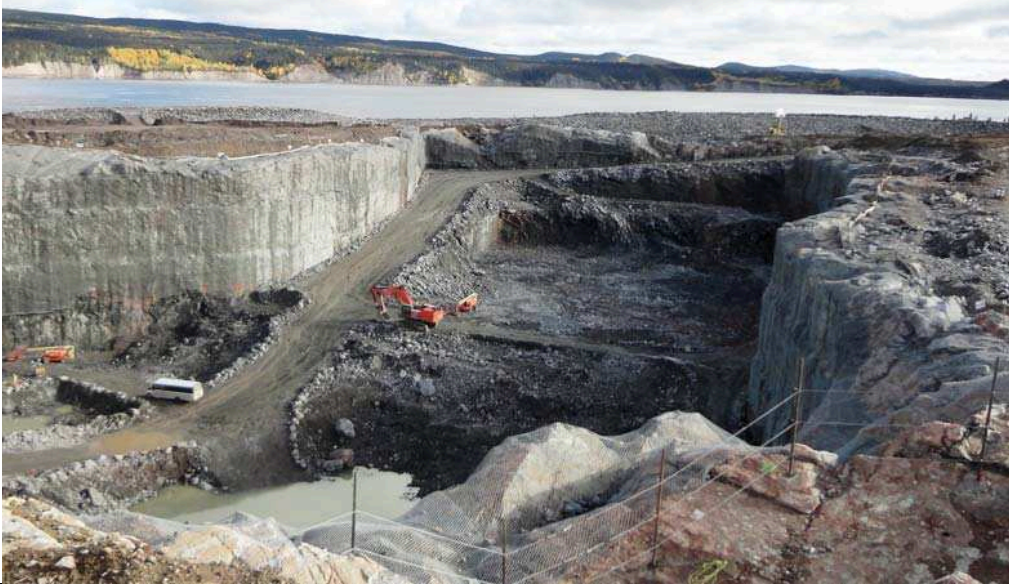
Photo 12: Powerhouse/tailrace excavation looking downstream (09/26/2013)
