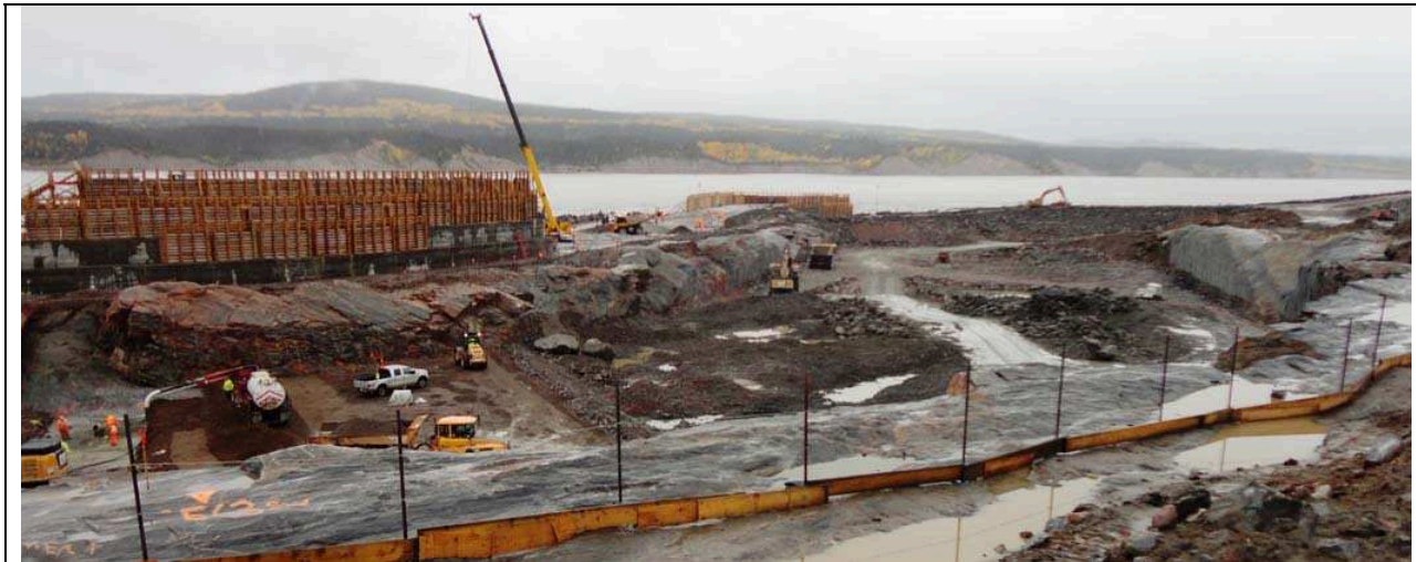
Photo 22: Spillway, downstream area (09/25/2013)
