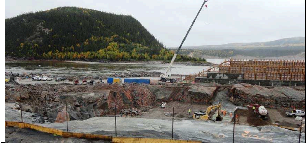
Photo 23: Spillway. Upstream end of north wall (09/25/2013)
