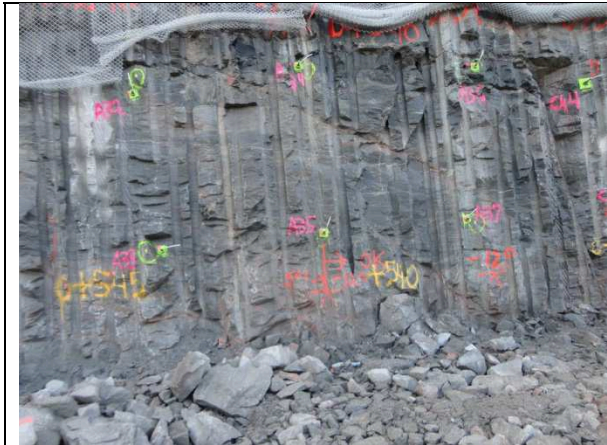
18a: Line drilling results in powerhouse wall
