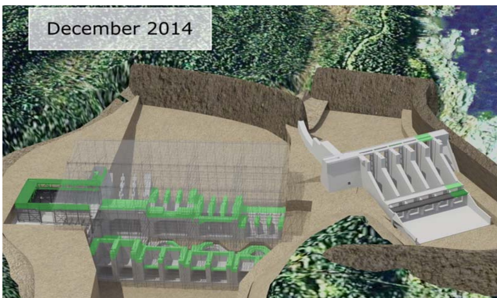
Figure 17: Intake, Powerhouse and Spillway civil works end-2014
