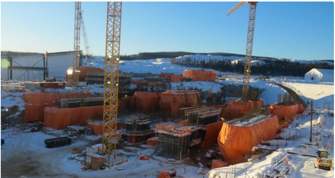
Progress on the Spillway at the Muskrat Falls Site – December 2014
