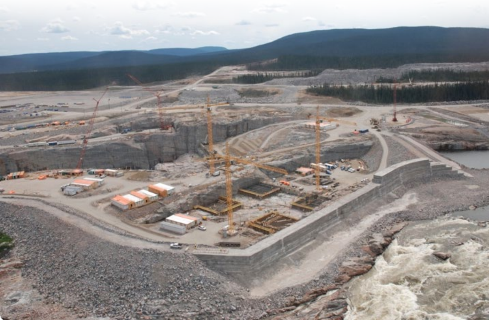
Muskrat Falls Construction Site – Powerhouse and Spillway - August 2014
