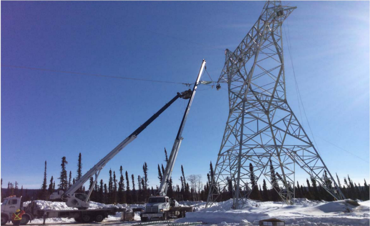
Labrador Transmission Assets – Stringing Operations – March 2015
