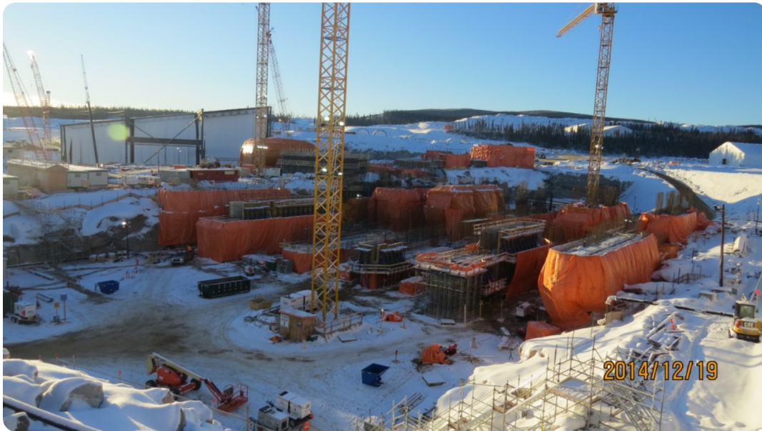
Progress on the Spillway at the Muskrat Falls Site - December 19, 2014
