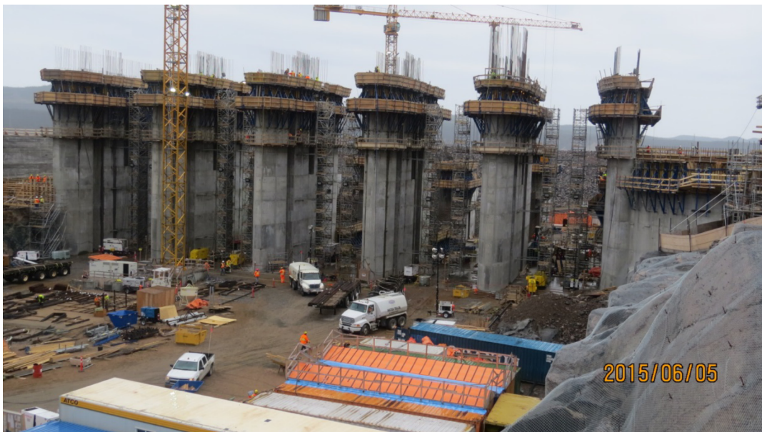
Progress on the Spillway, June 5, 2015
