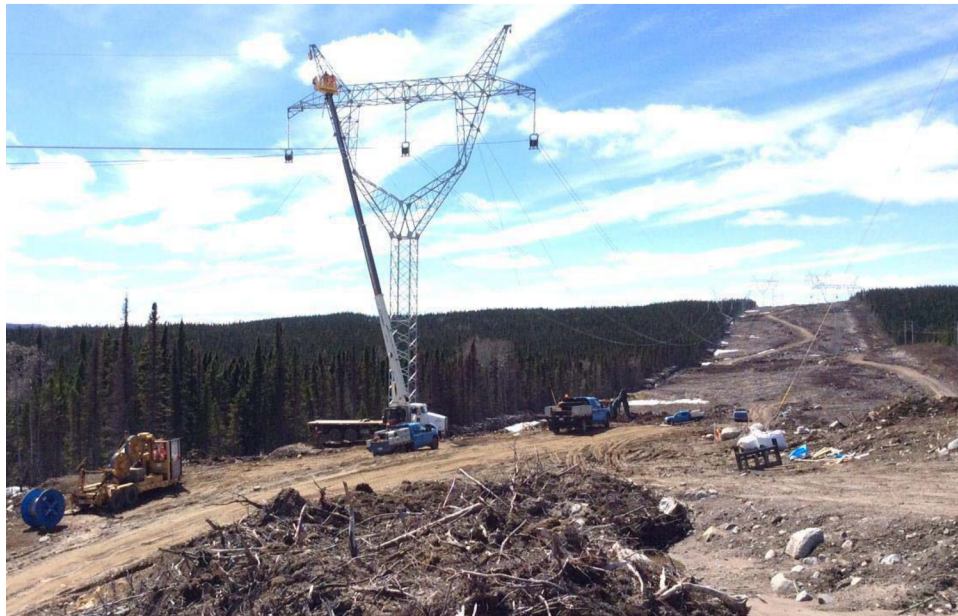
LTA Stringing Operations
