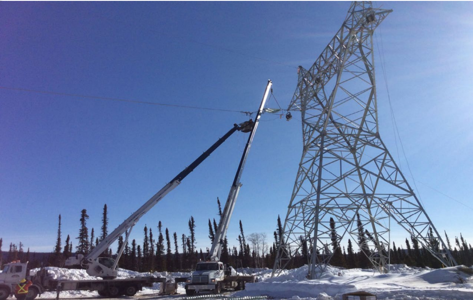
Labrador Transmission Assets – Stringing Operations – March 2015
