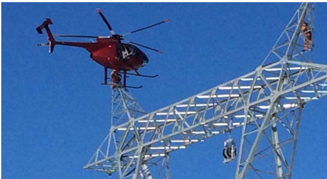
Labrador Transmission Assets Stringing Operations
