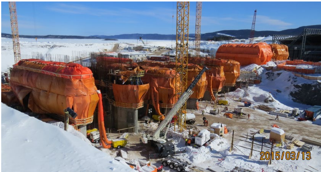
Progress on the Spillway at the Muskrat Falls Site – March 13, 2015
