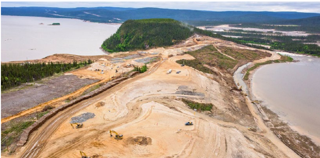
Muskrat Falls Site – Progress on North Spur – August 2015
