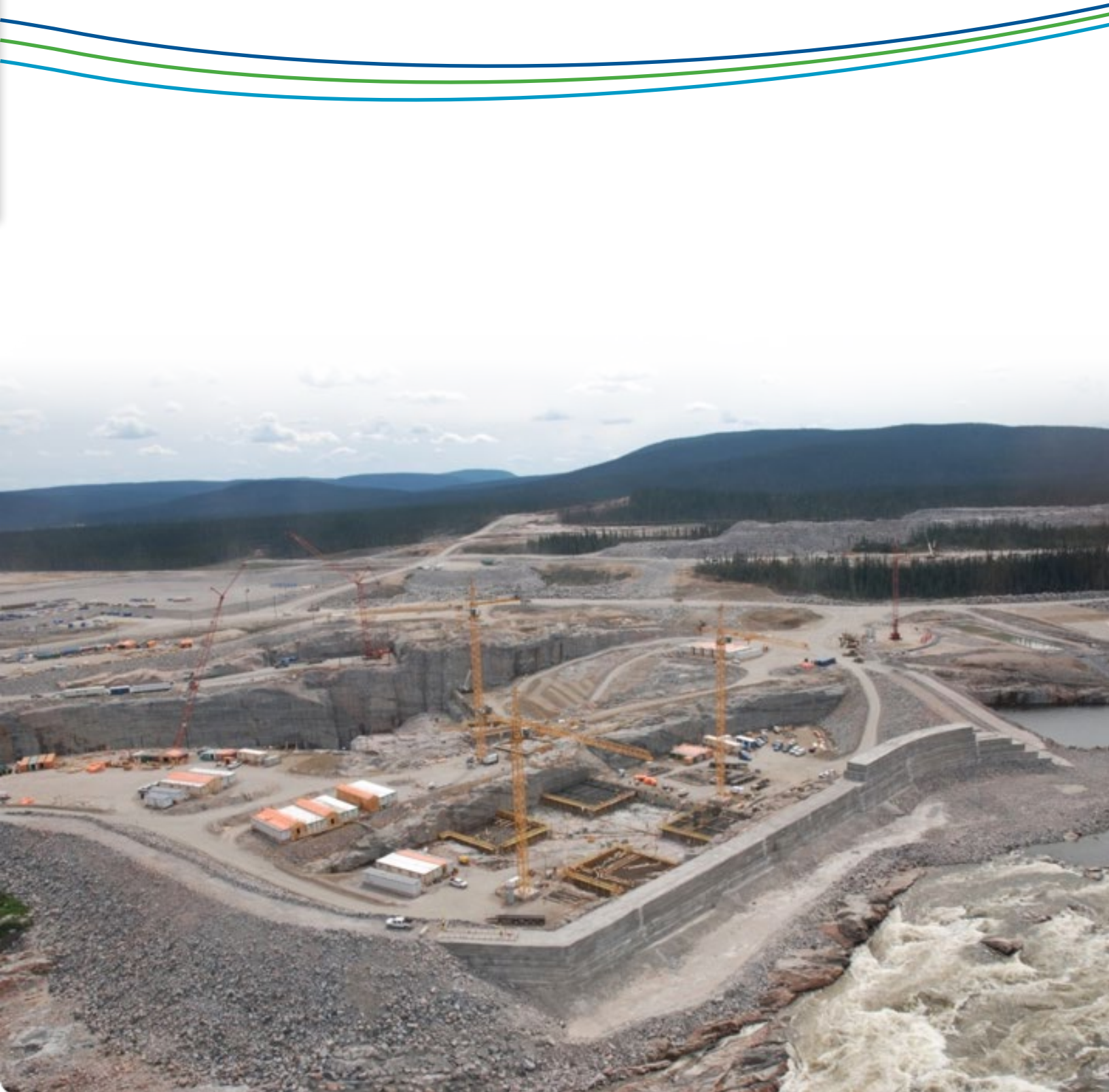
Muskrat Falls Construction Site – Powerhouse and Spillway - August 2014
