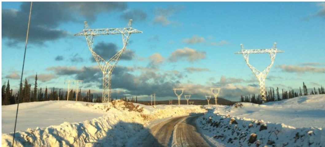
Installed towers for the Labrador Transmission Assets transmission line – November 2014
