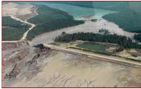
Mount Polley dam in BC. The downstream slope failed on August 14 th , 2014.
