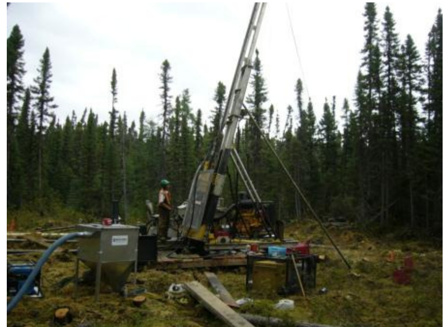
Borehole Operations at Muskrat Falls
