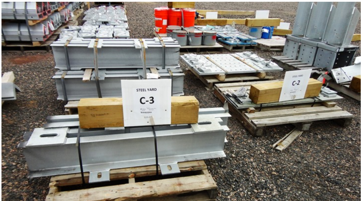
Photo 5.2: Goose Bay Marshalling Yard. Labeled transmission components for tower foundation (July 16, 2014)
