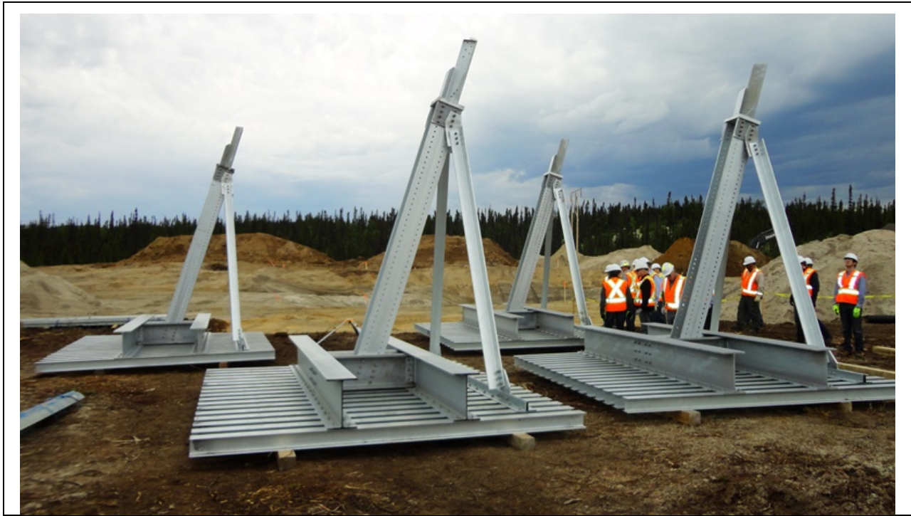
Photo 8.3: Transmission Tower Erection and Foundations. Assembled grillage footings. (July 16, 2014)
