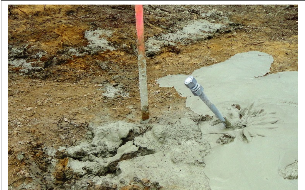
Photo 8.7: Transmission Tower Erection and Foundations. Installed, fully grouted ground anchor. (July 16, 2014)
