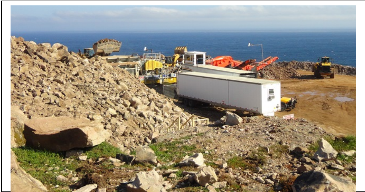
Photo 4.2: Forteau quarry. Crushing and screening plant in operation.
