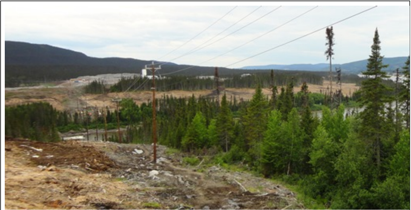
Photo 7.1: North Spur. View from top of North Spur looking towards the upstream Churchill River. Note reservoir clearing in center field and right bank quarry aggregate stockpile in background. (July 16, 2014)
