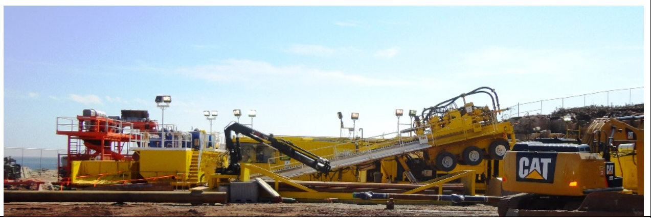
Photo 2.1: Forteau Directional Drilling. Inclined drill and equipment. (July 15, 2014)
