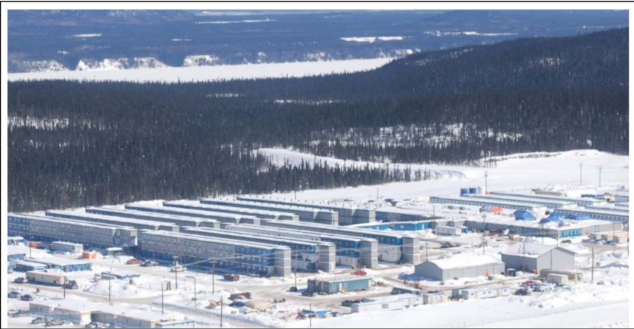
Photo 5.3: Muskrat Falls Camp, permanent and starter (Nalcor photo -Winter 2014)
