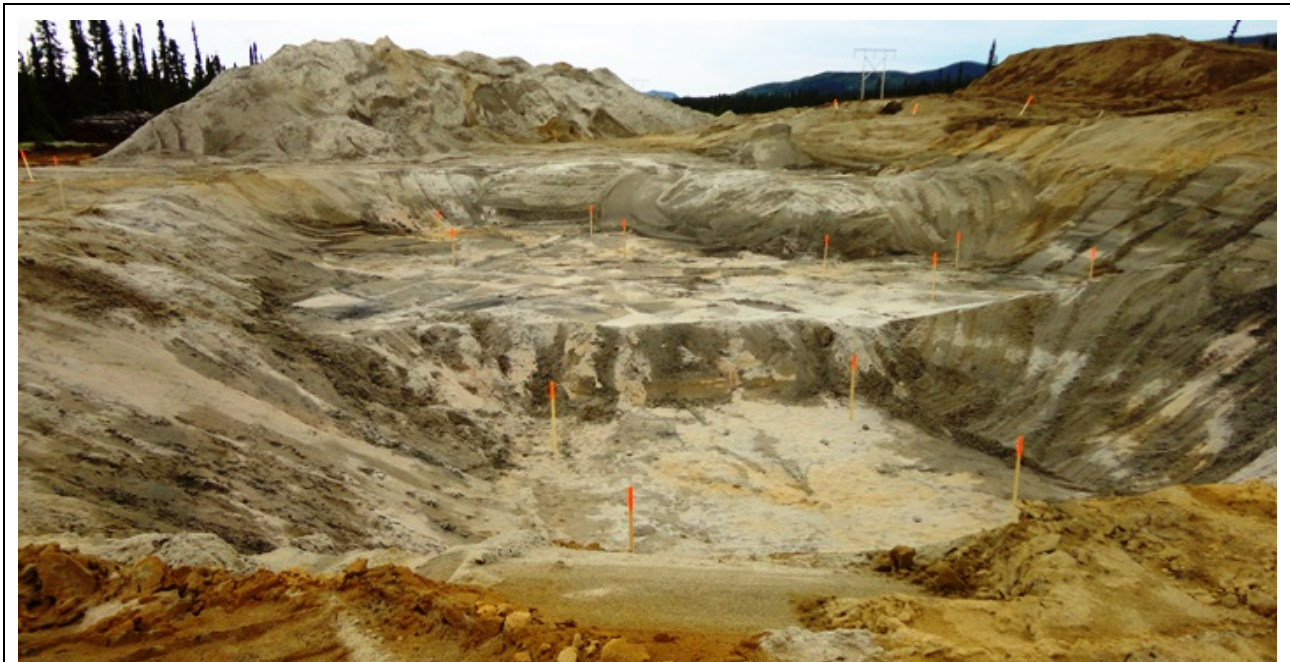
Photo 8.2: Transmission Tower Erection and Foundations. Excavated and prepared tower foundation (July 16, 2014)
