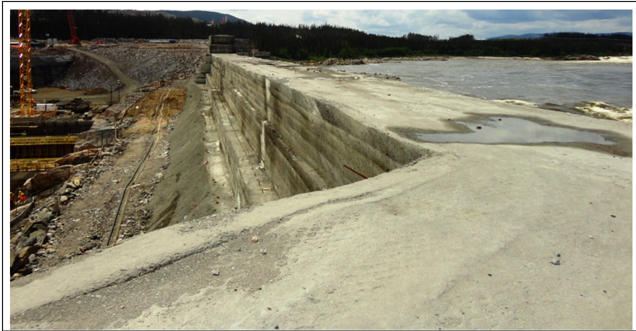
Photo 6.4: RCC cofferdam above spillway left wall. (July 17, 2014)
