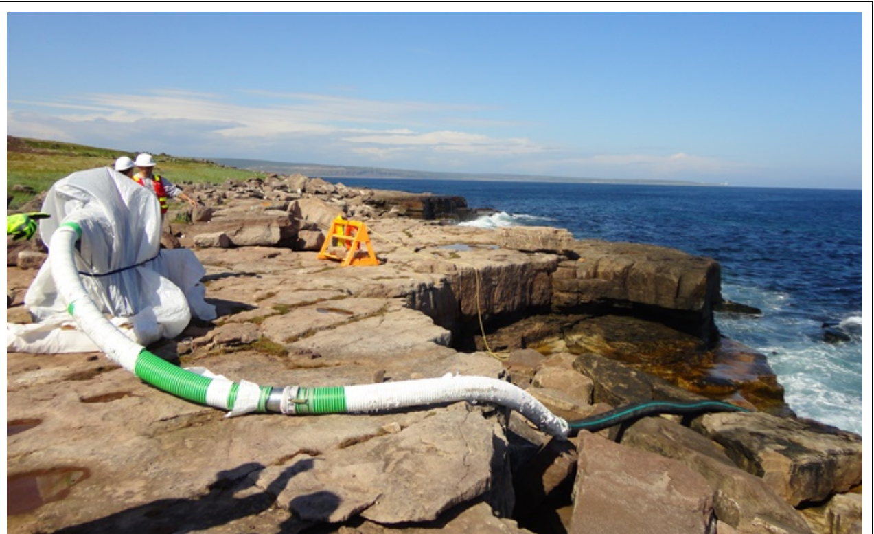
Photo 2.2: Forteau Directional Drilling. Subhorizontal bedded sandstone at the Forteau drilling site.
