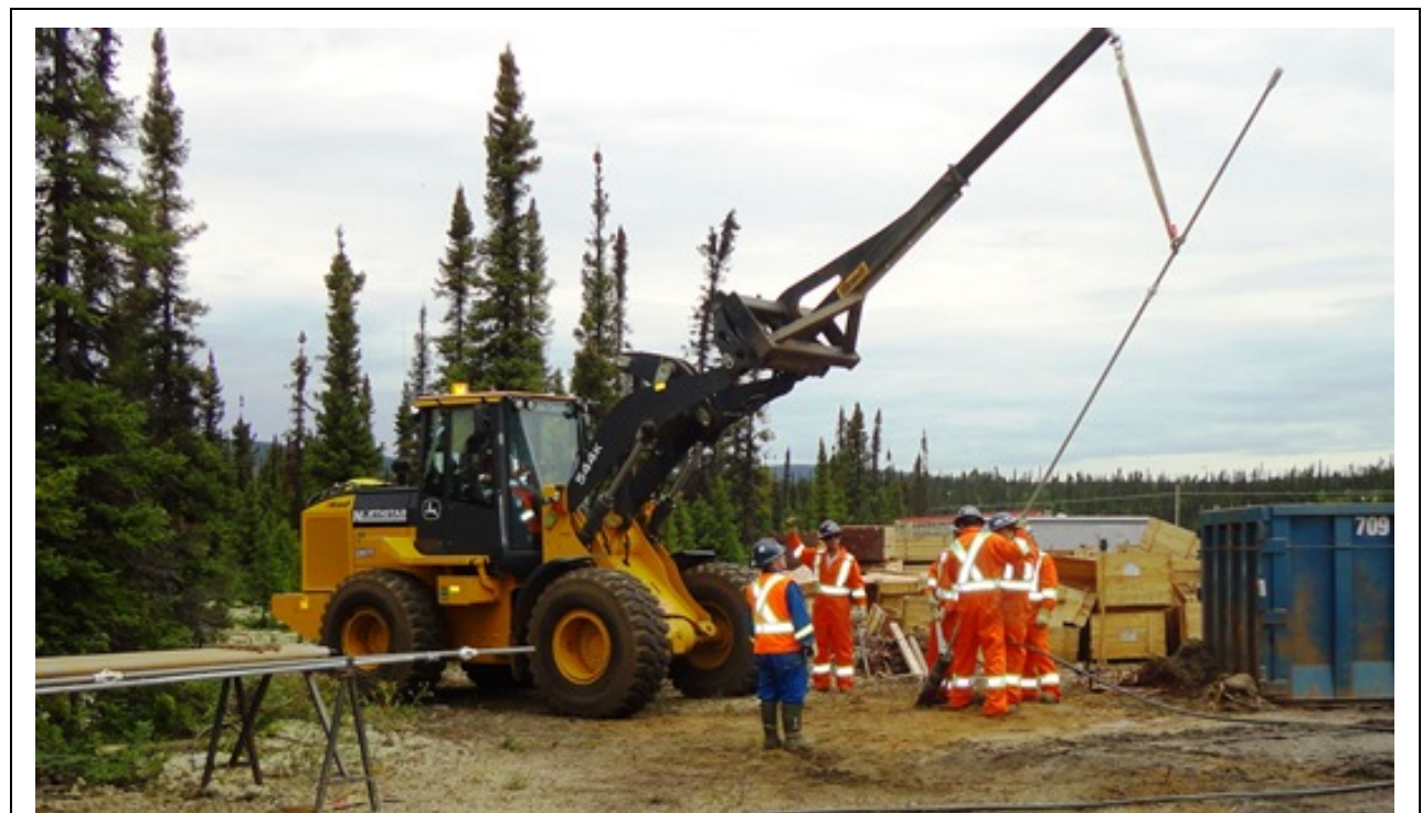
Photo 8.6: Transmission Tower Erection and Foundations. Installing a ground anchor. (July 16, 2014)
