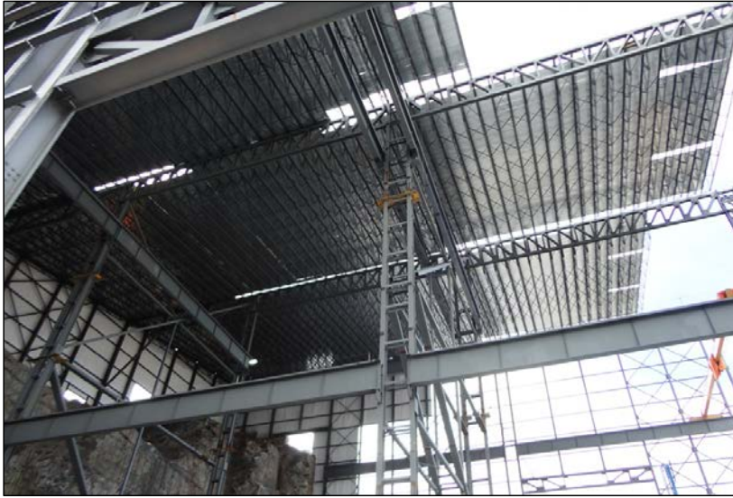
Photo 8.5: Powerhouse ICS Roof over Units 1 and 2. (November 26, 2014)
