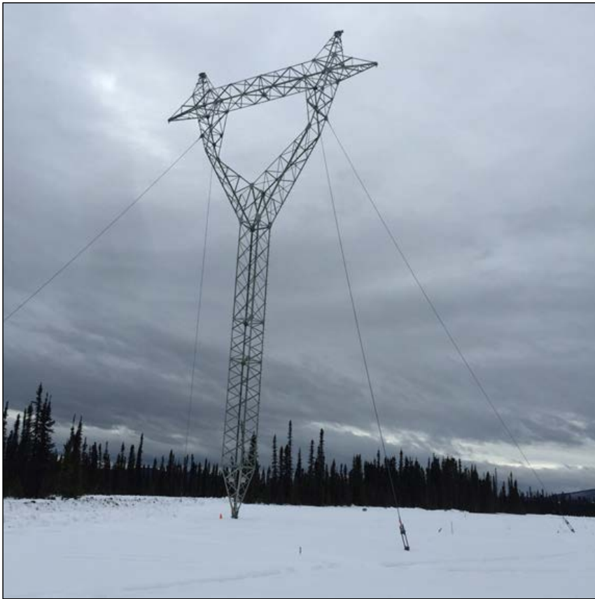
Photo 5.1a: HVac transmission line – erected guyed structure. (November 26, 2014)
