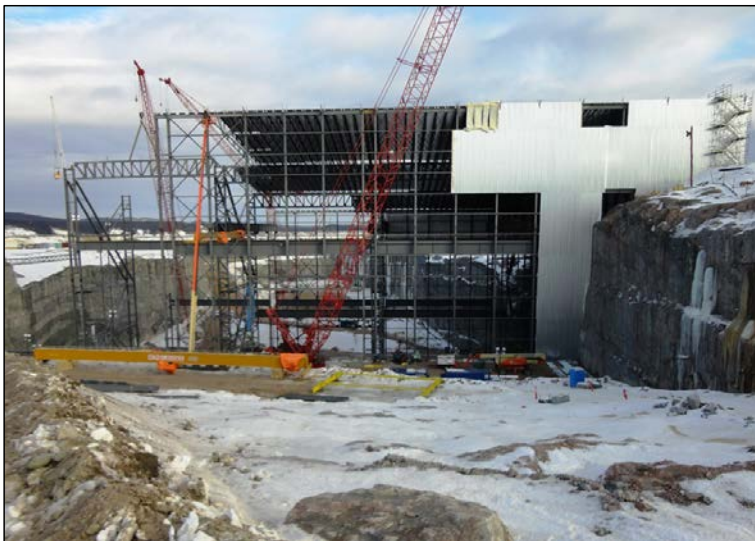
Photo 8.2: Powerhouse ICS looking downstream. Framework and cladding in Units 1, 2 and 3 can be seen. (November 26, 2014.)
