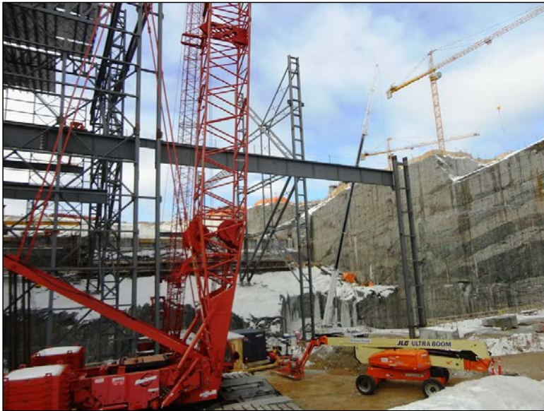
Photo 8.4: View looking upstream at the initial ICS framework erection over Unit 3 (November 26, 2014)
