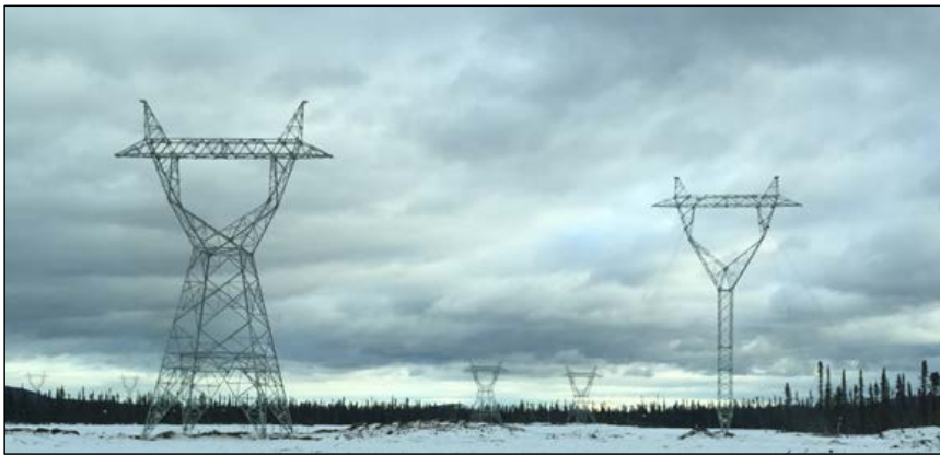
Photo 5.1c: HVac transmission line – erected Structures – Looking South toward both Lines. (November 26, 2014)
