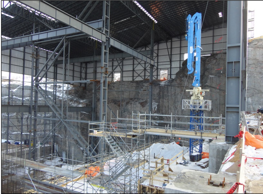
Photo 8.13: Putzmeister concrete pump on a fixed swivel mounting between Bays 2 and 3 in the Powerhouse. Additional pumps will be installed throughout the powerhouse to make sure that all areas can be reached. (November 26, 2014)
