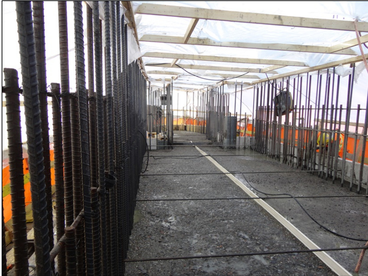
Photo 7.9: Current top of Pier 3 looking upstream. The concrete was green cut on the previous day and was currently being washed at the time of the photograph. Note the cut-out for the upstream stop logs in the background and the white water stop running down the centerline of the pier. (November 26, 2014)
