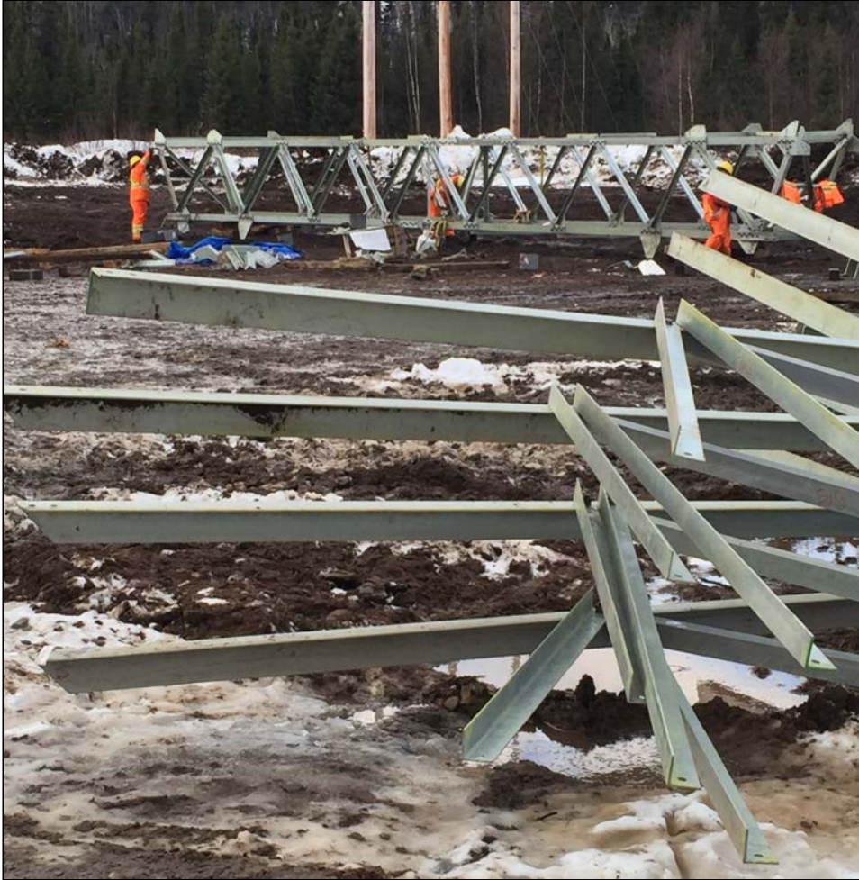
Photo 3.3: HVac transmission line structure assembly, November 25, 2014
