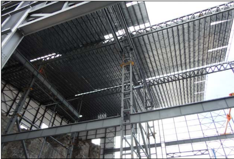
Photo 8.5: Powerhouse ICS Roof over Units 1 and 2. (November 26, 2014)
