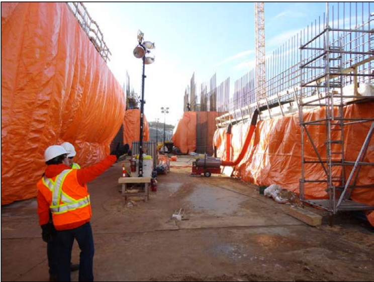
Photo 7.4: Spillway; view looking upstream between North Piers and Pier 1. (November 26, 2014)
