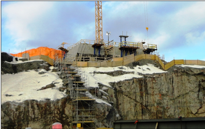
Photo 8.14: Right end of transition dam adjoining the powerhouse intake. (November 26, 2014)
