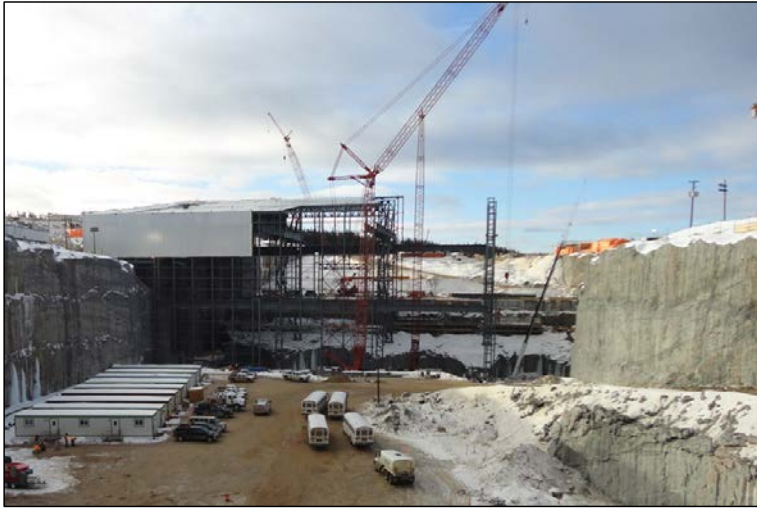
Photo 8.1: Powerhouse ICS looking upstream. Units 1 and 2 framework erection and first roof covering are substantially complete and almost half of the wall cladding has been erected. At Unit 3 the framework and first roof covering are substantially complete but no progress has been made on the wall cladding. No progress with the ICS in the area of Unit 4. . (November 26, 2014.)
