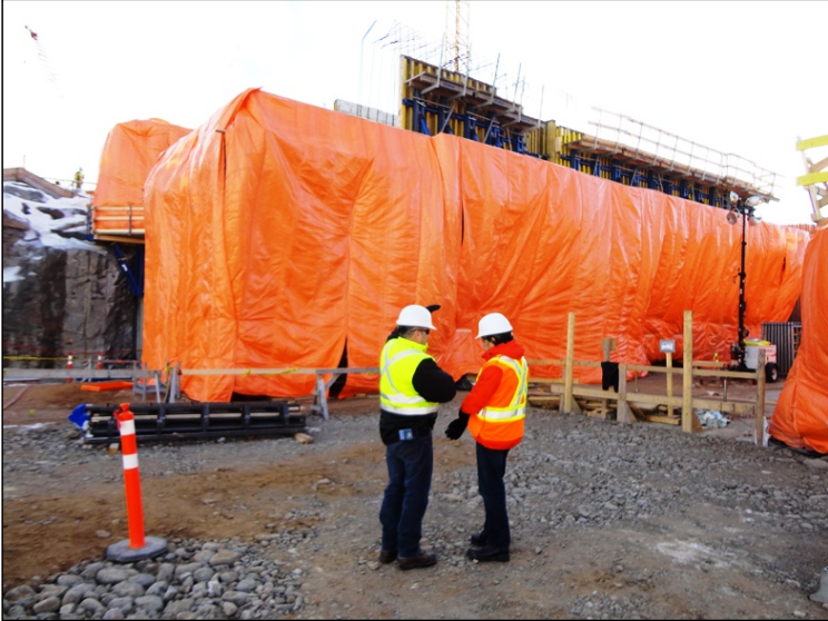
Photo 7.3: Right side of the spillway. Transition dam is visible at the top of the photograph. (November 26, 2014)
