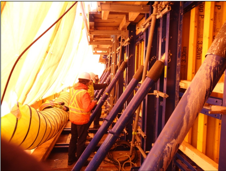
Photo 7.6: Spillway; shrouded and heated formwork. (November 26, 2014)
