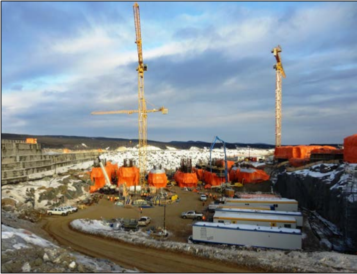
Photo 7.1: Spillway; view looking downstream towards the piers. RCC cofferdam is visible on the left side and the orange tarp covered transition dam is on the right. (November 26, 2014)
