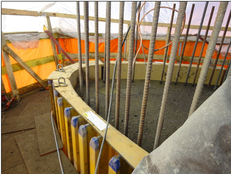
Photo 7.8: Spillway; Upstream nose of Pier 3. (November 26, 2014)
