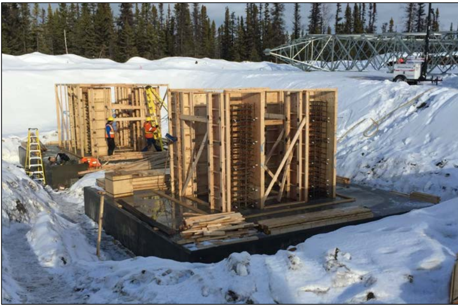
Photo 1.1 HVAC transmission line foundation installation. (November 25, 2014)
