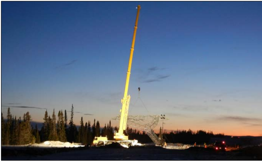
Photo 4.1: HVac transmission line – structure erection, November 26, 2014
