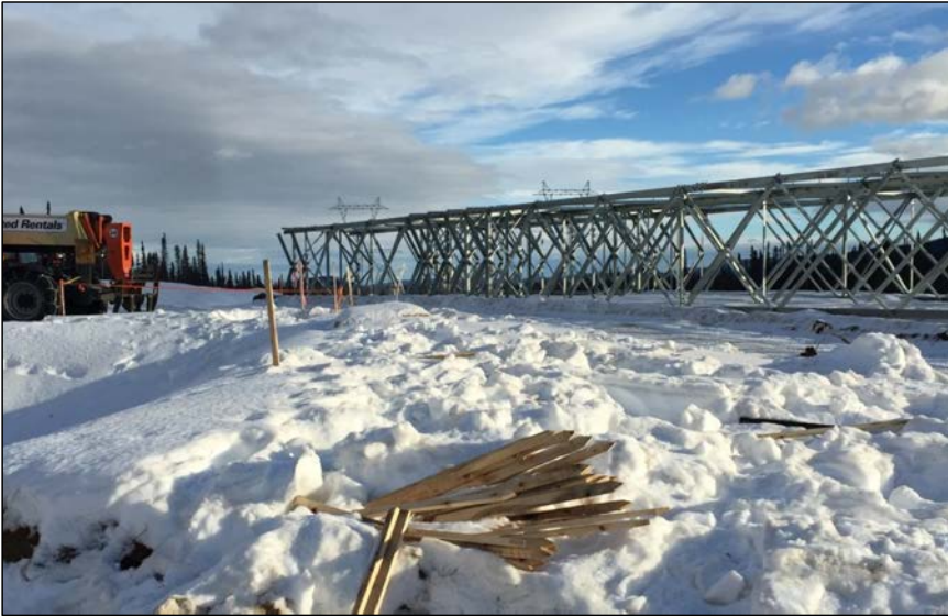
Photo 3.1: HVac transmission line structure assembly, November 25, 2014
