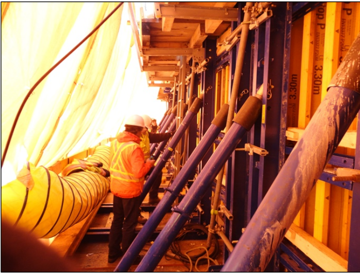
Photo 7.6: Spillway; shrouded and heated formwork. (November 26, 2014)
