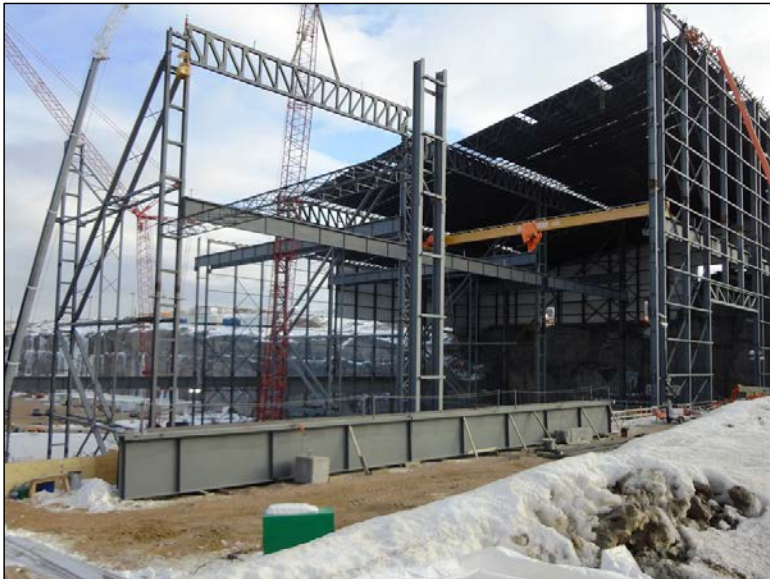
Photo 8.10: View looking downstream at the ICS framework over Bay 3. (November 26, 2014)
