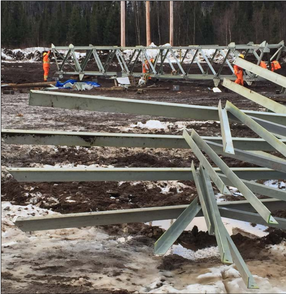
Photo 3.3: HVac transmission line structure assembly, November 25, 2014
