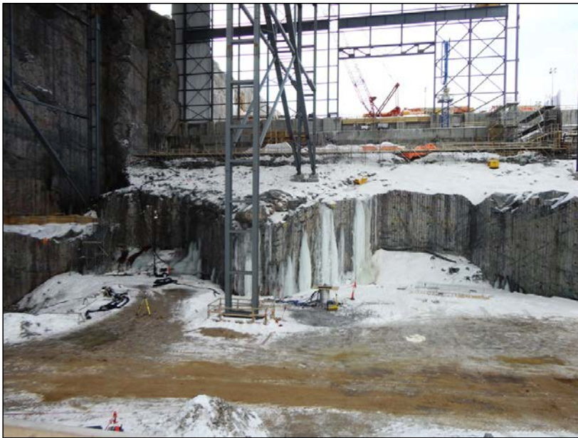
Photo 8.6: Final rock faces in Powerhouse bays 1 and 2. (November 26, 2014)
