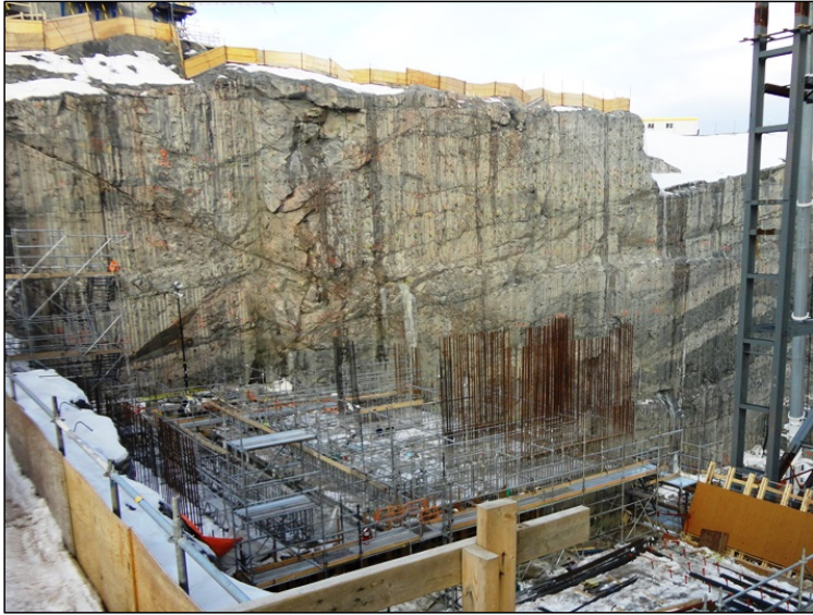
Photo 8.11 Powerhouse, Bay 4. Permanent concrete at base of intake structure at Bay 4. This is the only permanent concrete in the powerhouse/intake structures. (November 26, 2014)
