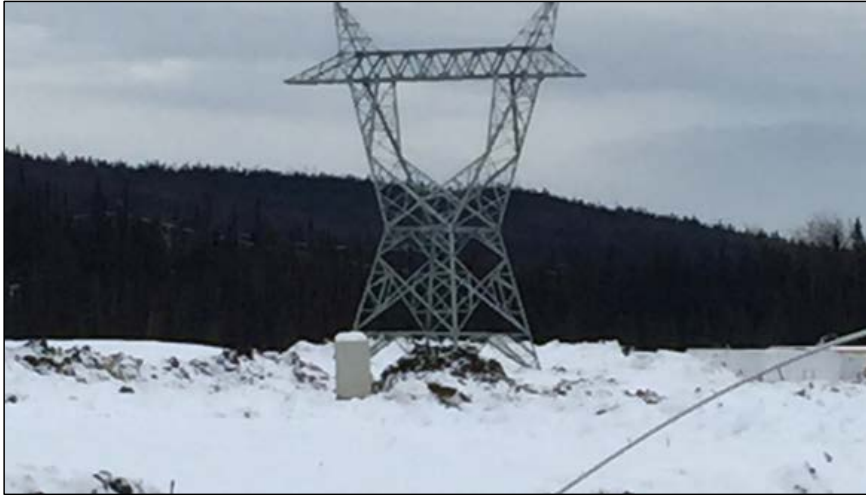
Photo 5.1b: HVac transmission line – erected Self Supporting Structure. (November 26, 2014)
