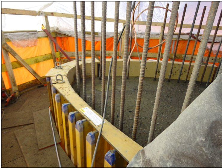
Photo 7.8: Spillway; Upstream nose of Pier 3. (November 26, 2014)
