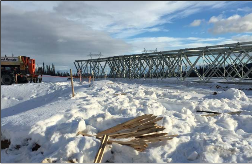
Photo 3.1: HVac transmission line structure assembly, November 25, 2014
