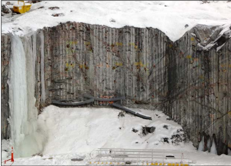
Photo 8.7: Powerhouse Bay 2. Photo shows the excellent quality of the blasting. (November 26, 2014)
