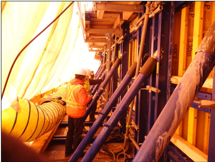
Photo 7.6: Spillway; shrouded and heated formwork. (November 26, 2014)
