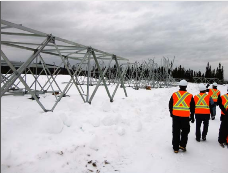
Photo 3.2: Assembling a HVacAC transmission tower near the North Spur. (November 25, 2014)
