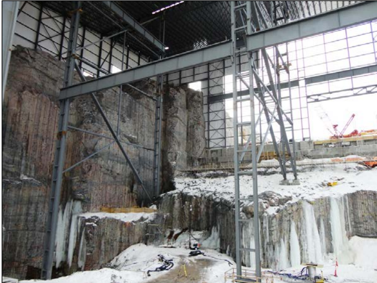
Photo 8.9: View looking upstream at the interior of the ICS over Bays 1 and 2. (November 26, 2014)
