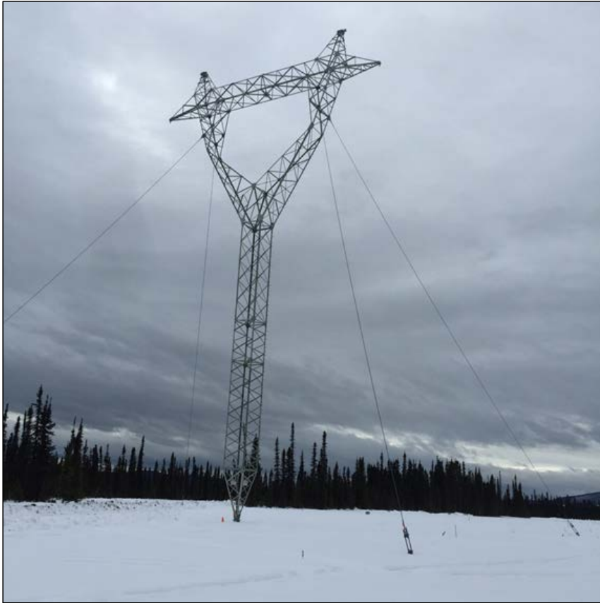
Photo 5.1a: HVac transmission line – erected guyed structure. (November 26, 2014)
