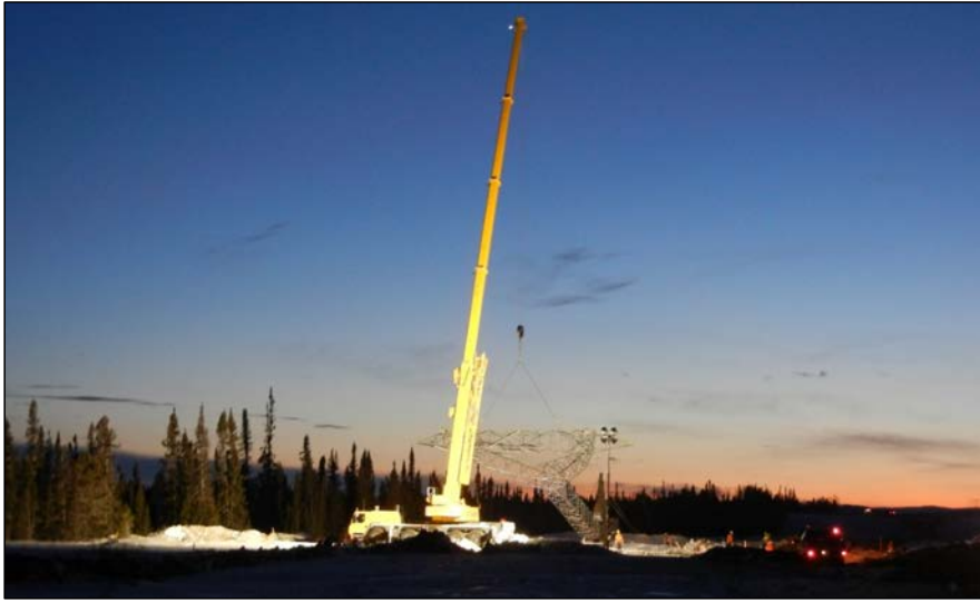
Photo 4.1: HVac transmission line – structure erection, November 26, 2014
