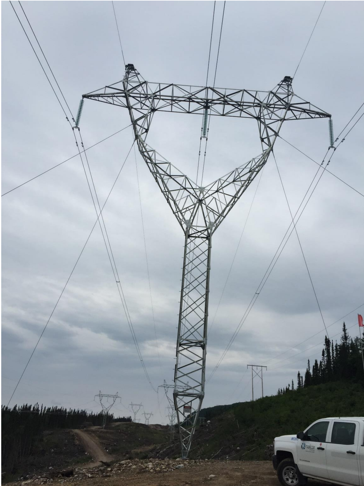
Photo 4.3 HVac transmission line erection (July 7, 2015).
