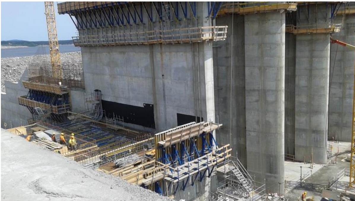
Photo 6.2 Upstream view of Spillway piers and North Transition Dam (July 7, 2015).
