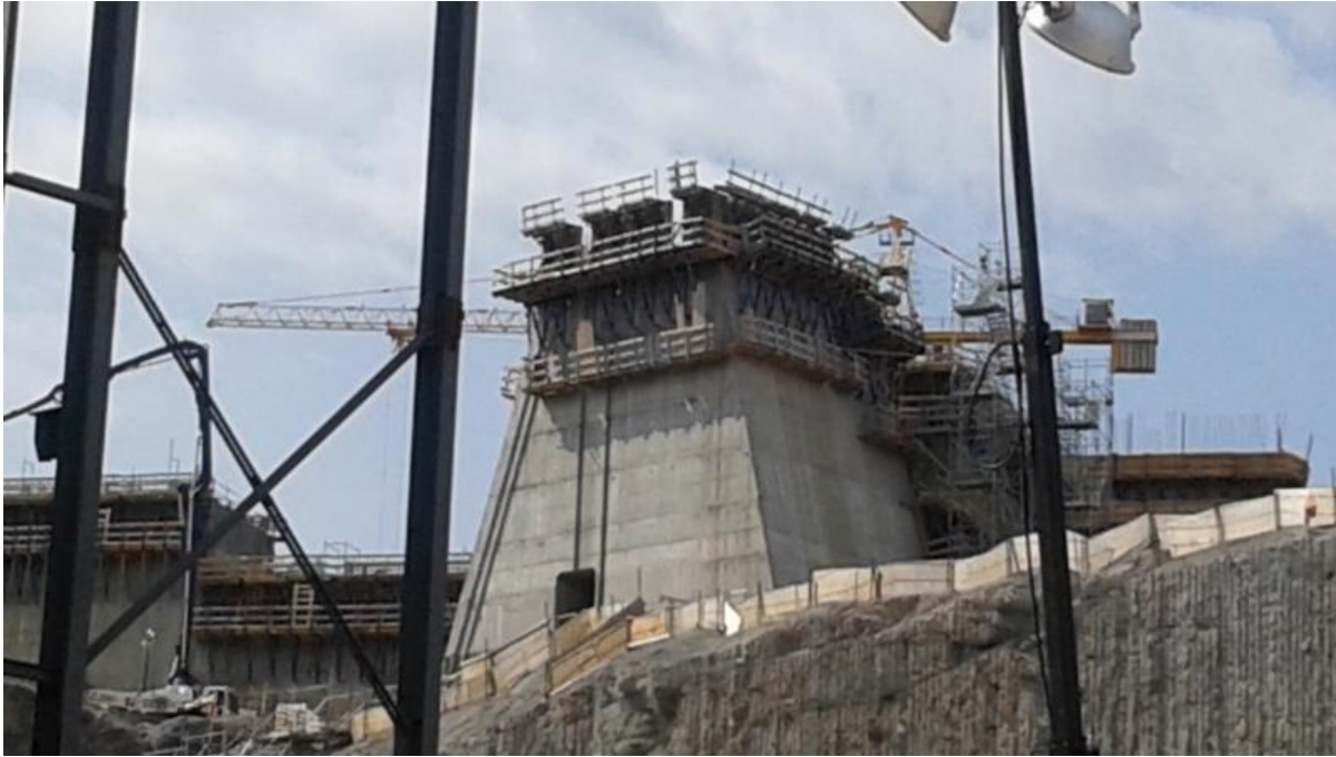
Photo 6.3 Upstream view of Central Transition Dam (July 7, 2015).
