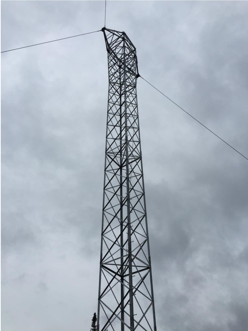
Photo 3.3 HVdc transmission line installation ( July 8, 2015 ).
