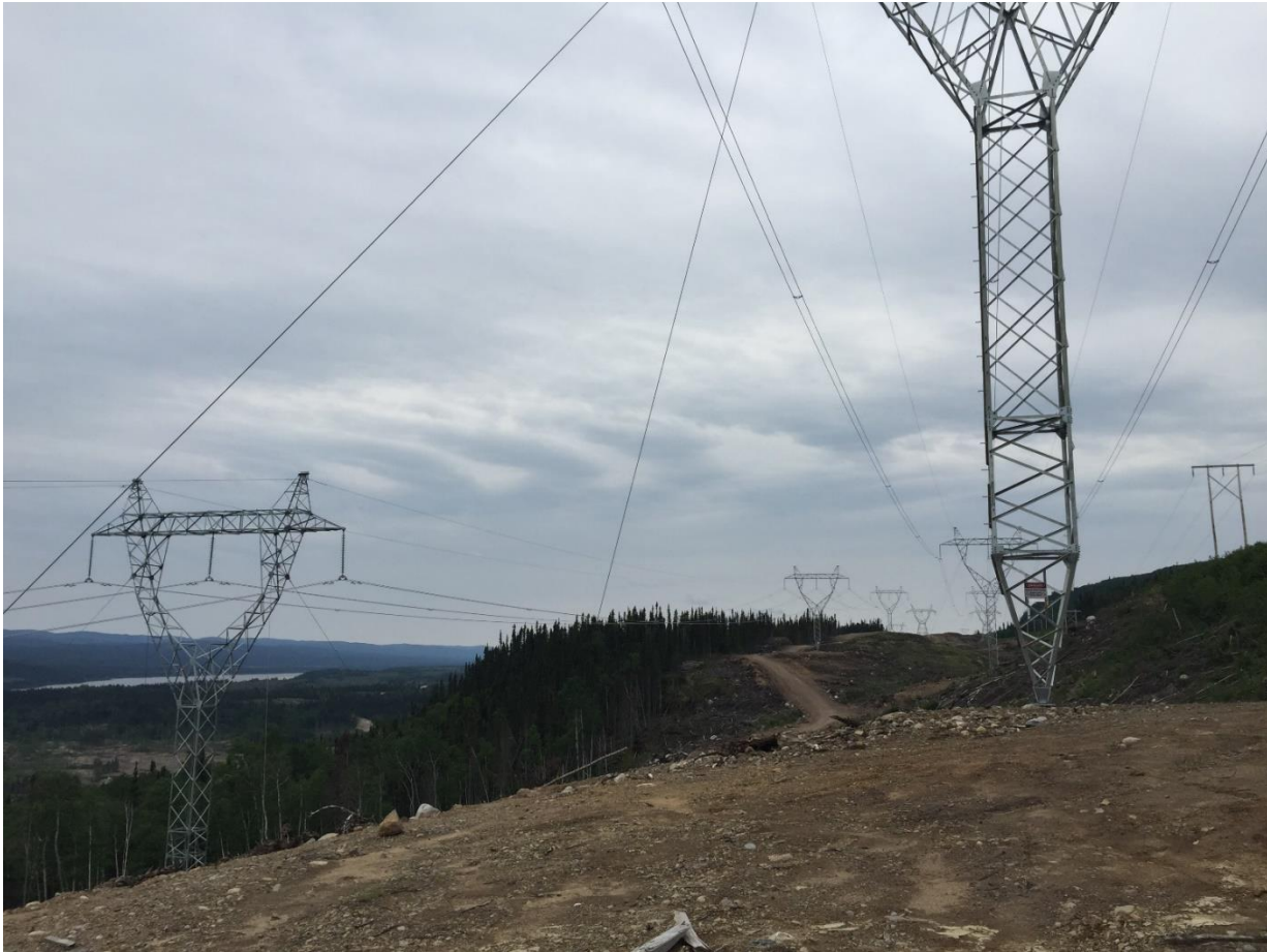
Photo 4.2 HVac transmission line clearing and clean up ( July 7, 2015 ).
