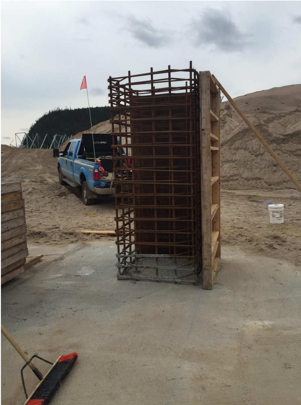
Photo 4.5 HVac transmission line – Concrete foundation ( July 7, 2015 ).
