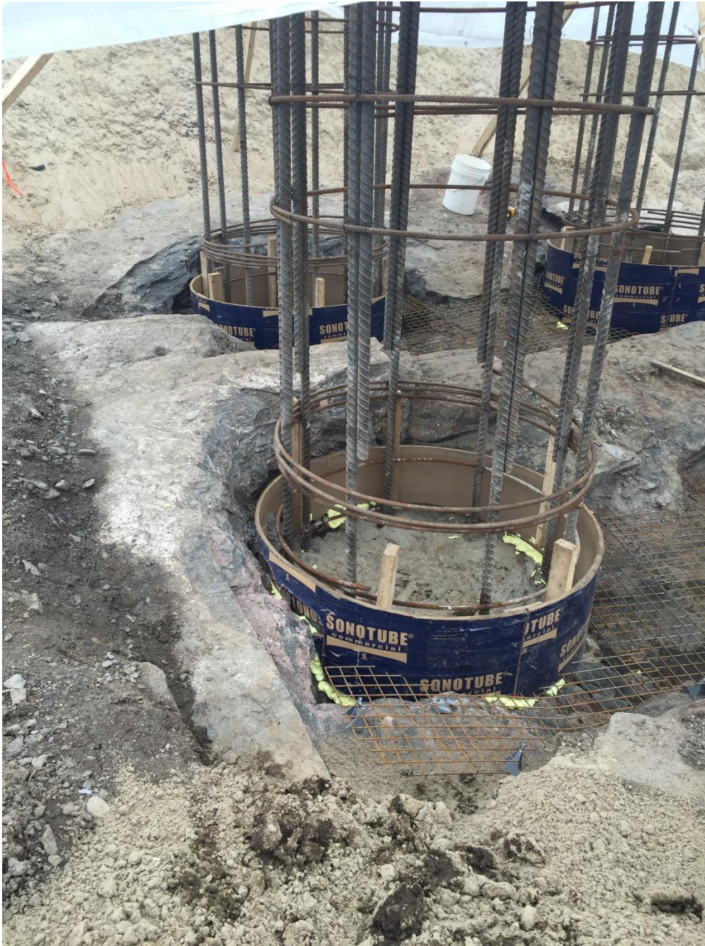
Photo 4.4 HVac transmission line – Rock foundation (July 7, 2015).
