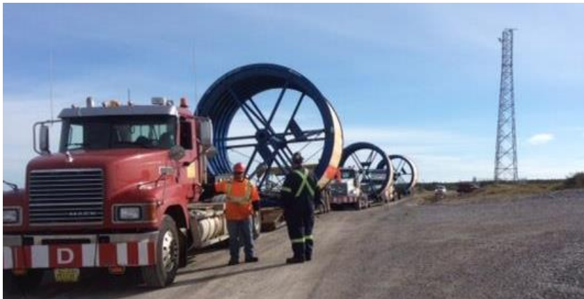
Arrival of land cables in Shoal Cove
