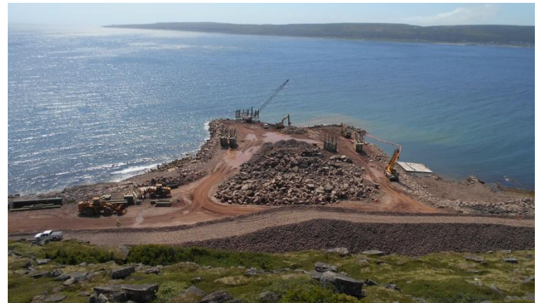
Quay construction, Forteau
