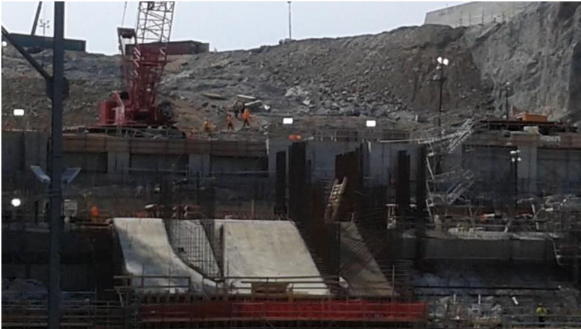
Photo 7.1 Unit 3 – Intake invert slab completed with central pier reinforcement dowels in place (July 7, 2015).
