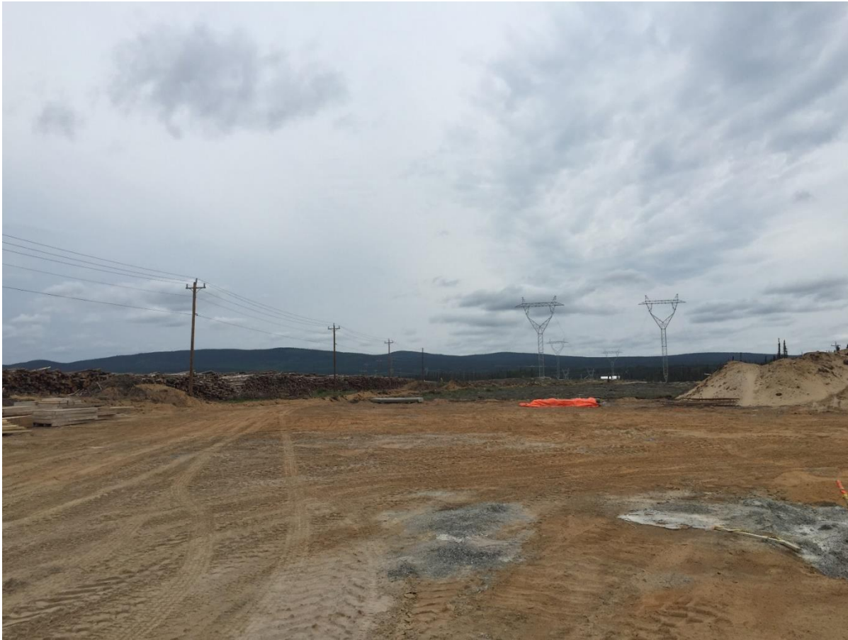
Photo 4.1 HVac transmission line clearing and clean up ( July 7, 2015 )
