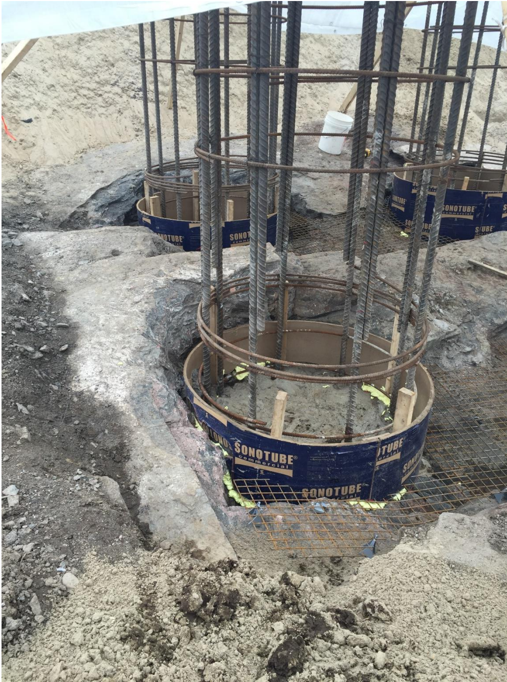
Photo 4.4 HVac transmission line – Rock foundation (July 7, 2015).
