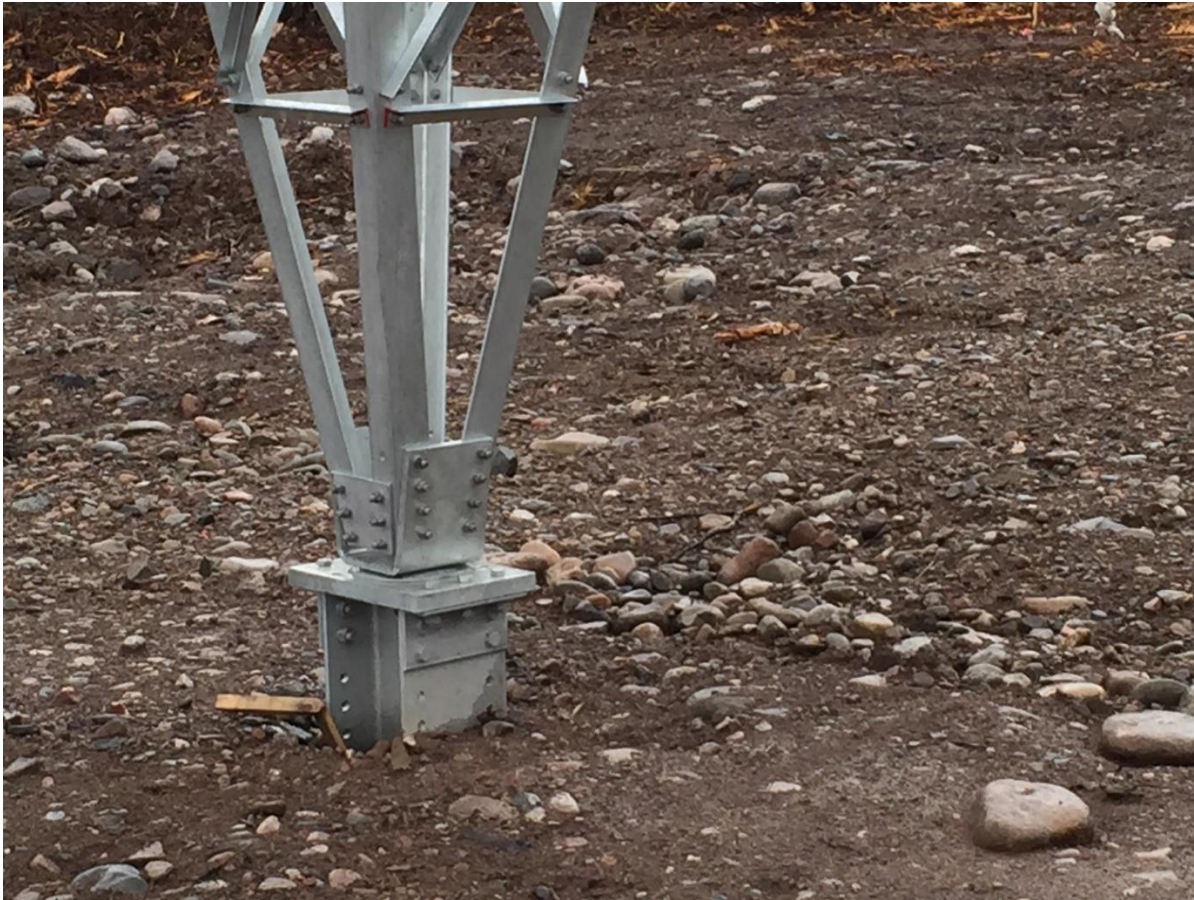
Photo 3.2 HVdc transmission line foundation installation ( July 8, 2015 ).
