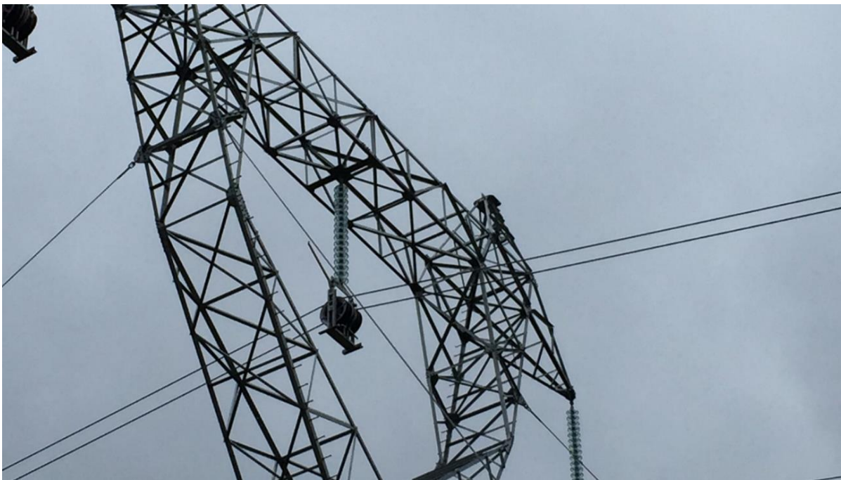
Photo 4.7 HVac transmission line – Stringing (July 8, 2015).
