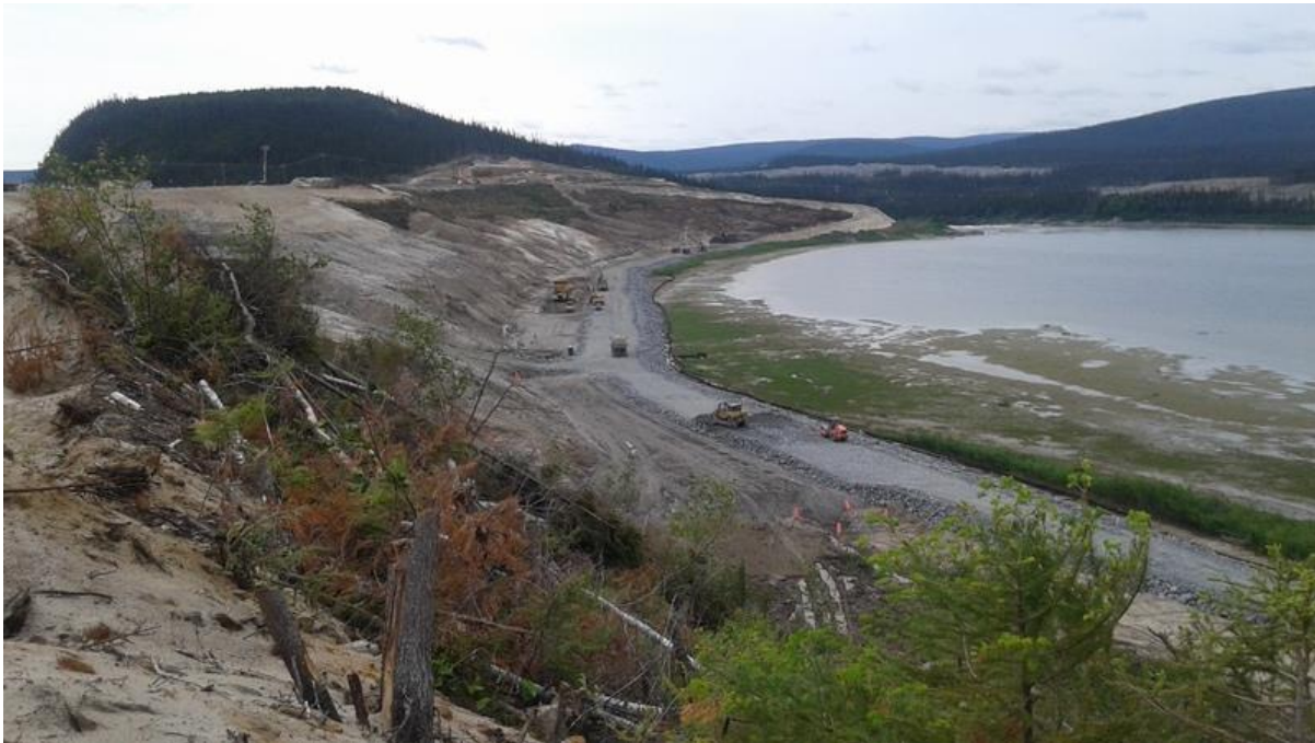
Photo 1.1 Looking at Upstream Slope of North Spur. Clearing and OM excavation completed. Contractor working on preparation of CB Work platform (July 7, 2015)
