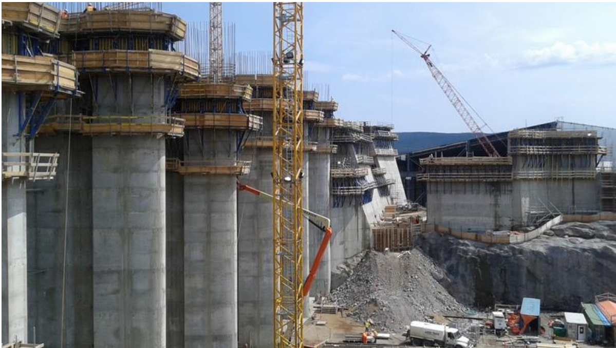
Photo 6.4 Side view of Spillway piers, Central Transition Dam and Separation Wall (July 7, 2015).
