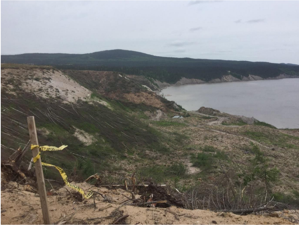
Photo 1.2 Looking at Downstream Slope of North Spur. (July 7, 2015)
