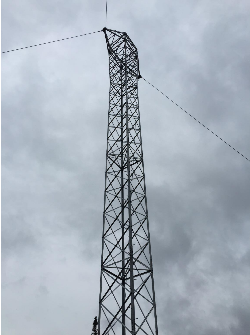
Photo 3.3 HVdc transmission line installation ( July 8, 2015 ).
