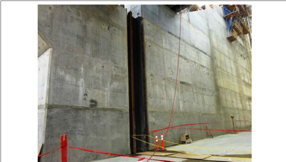
Photo 4.3: Spillway, Bay No. 2. Guide for downstream stop logs.
