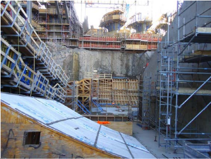
Photo 4.11: Powerhouse, Unit 2. Formworks are visible.
