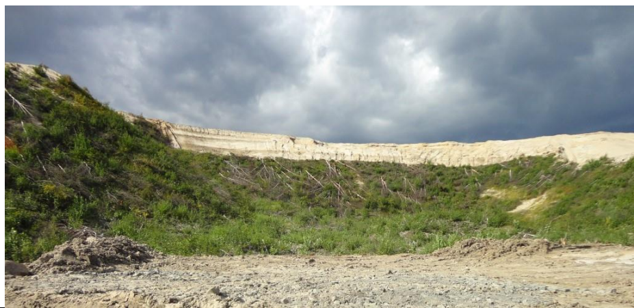
Photo 3.19: Downstream slope. View of the scarp of the 1978 landslide.
