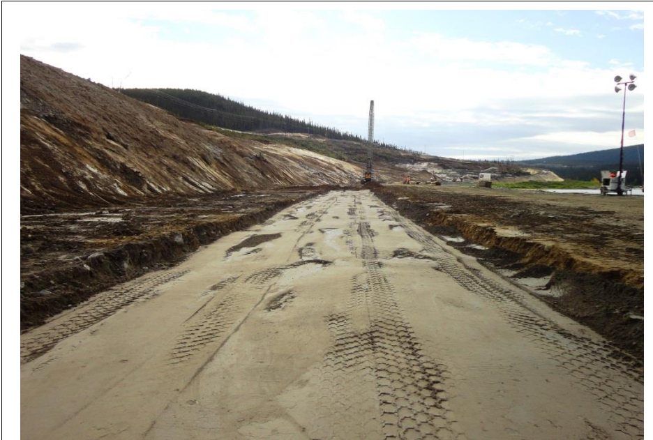
Photo 3.9: Upstream slope - Compacted fine grained till placed over the top of the cut-off wall at el 20m.
