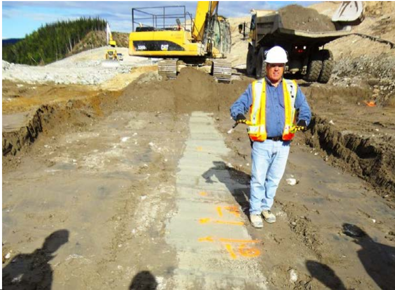
Photo 3.8: Upstream slope. Top of the cement/bentonite cut-off wall at el 20m. Note ongoing placement of the till blanket covering the wall in the background of the photograph.
