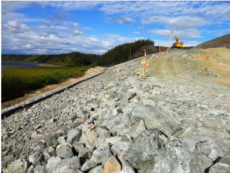
Photo 3.5: Upstream slope. Upstream rip rap blanket as viewed looking north from the el 24 m level.
