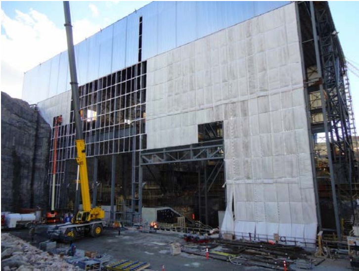
Photo 4.7: Powerhouse – ICS shelter structure over units 1 and 2 is currently being dismantled.
