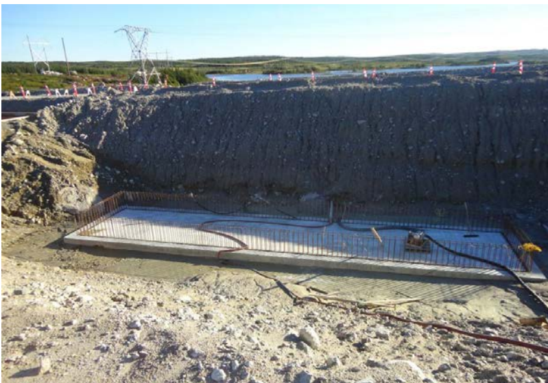
Photo 2.6: Base slab for oil/water separator
