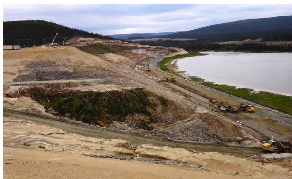
Photo 3.3: Upstream slope works, looking south from the north end.
