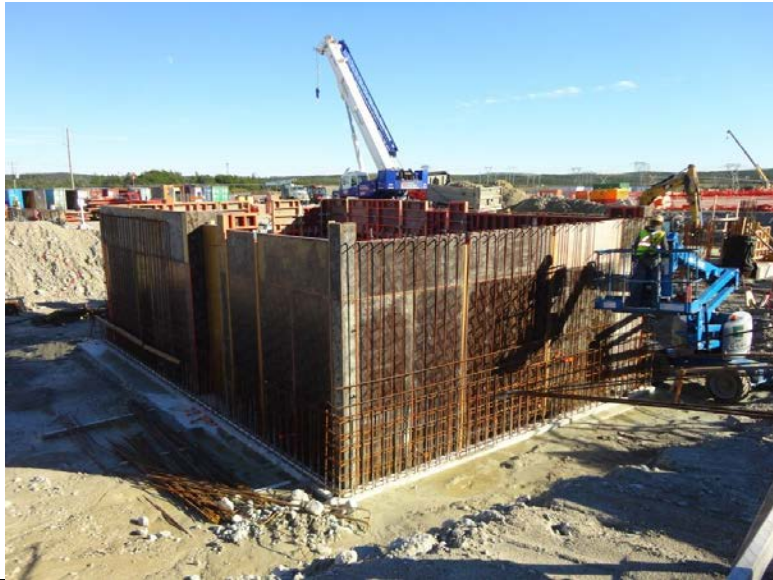
Photo 2.3: Formwork and rebar installation for water tank for synchronous condenser facility
