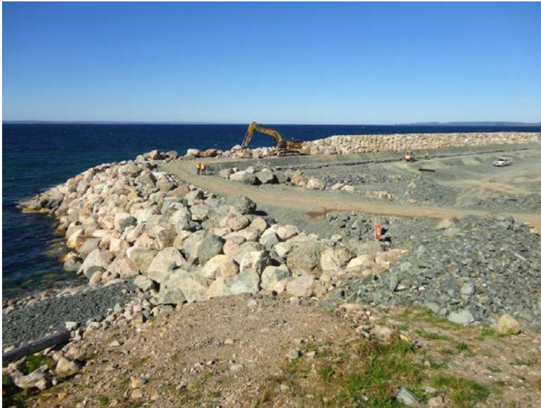
Photo 1.3: West end of the Dowden's Point dyke. Note the ongoing armour stone placement work.
