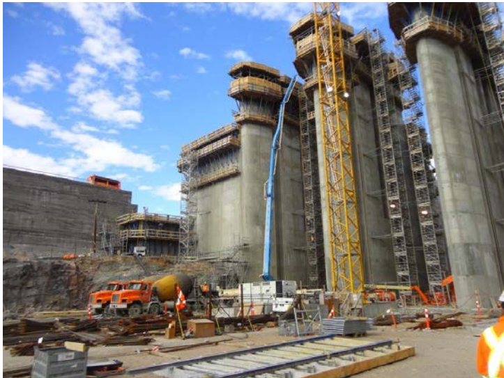
Photo 4.6: Spillway, right upstream corner. The RCC cofferdam and partially completed concrete transition dam are visible.
