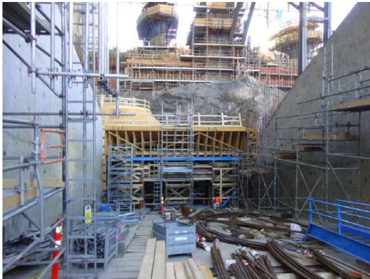
Photo 4.10: Powerhouse, Unit 1. Formwork for the scroll case is visible
