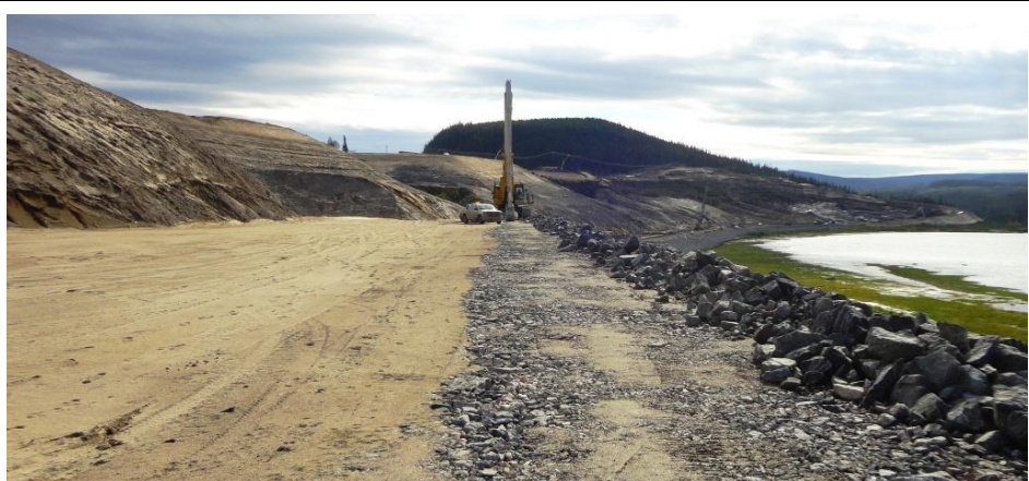
Photo 3.4: Upstream slope. El 28m berm at the north end of the cutoff. View shows, from right to left, the zoning of the rip rap, transition zones, and sandy fill/liner and till blanket.
