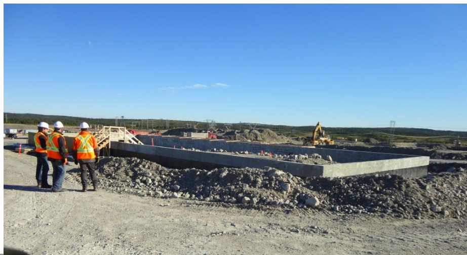
Photo 2.4: AC Substation Control Building foundation
