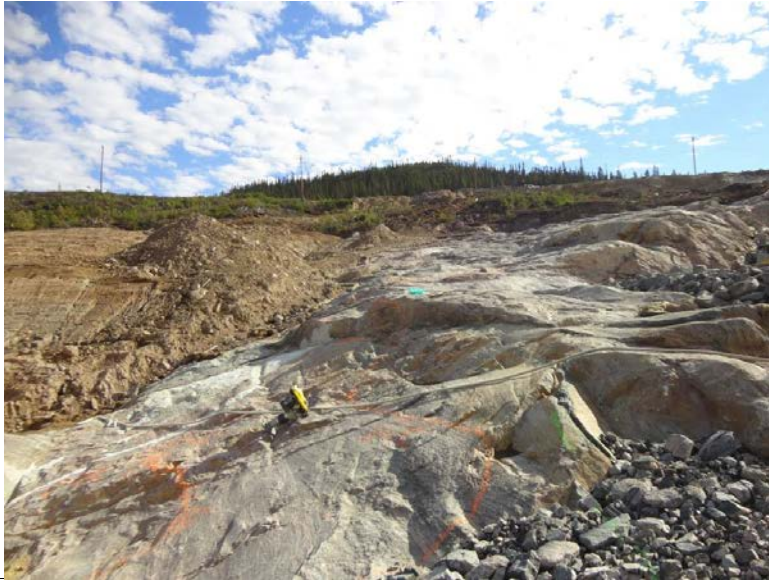
Photo 3.11: Upstream slope. Granitic bedrock exposed at the periphery of the rock knob at the south end of the upstream slope.
