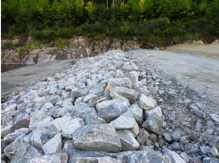
Photo 3.23: Downstream slope. Toe rip rap and granular transition zone.
