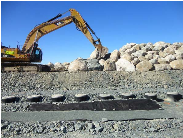
Photo 1.6: Placing and dressing the armour stone at the west end of the dyke. Electrode wells visible in foreground.
