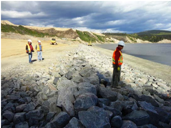
Photo 3.24: Downstream slope, toe rip rap
