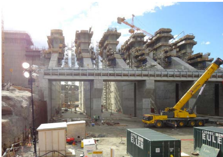
Photo 4.2: Spillway, downstream side as viewed looking upstream.
