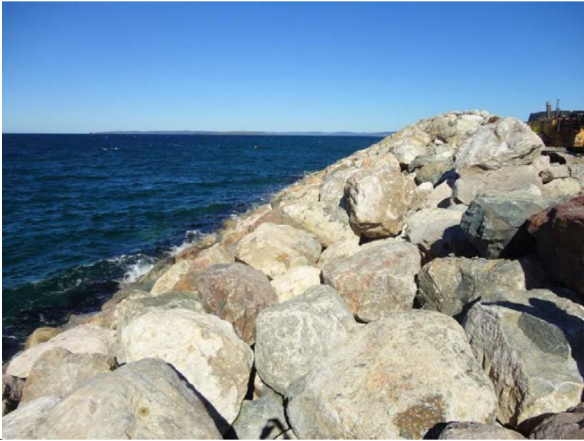
Photo 1.7: Armour stone blanket on the outer slope.
