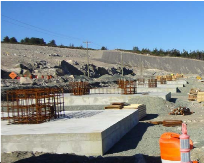
Photo 2.8: Foundation pads of the gantries in the AC transformers substation
