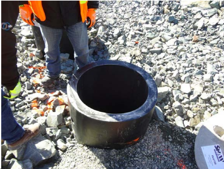
Photo 1.5: Electrode well casing installation
