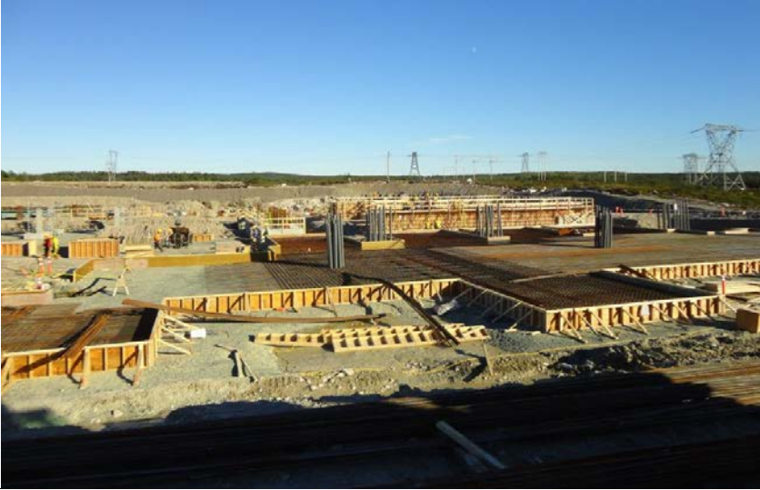
Photo 2.9: DC transformer foundation pads, southern area
