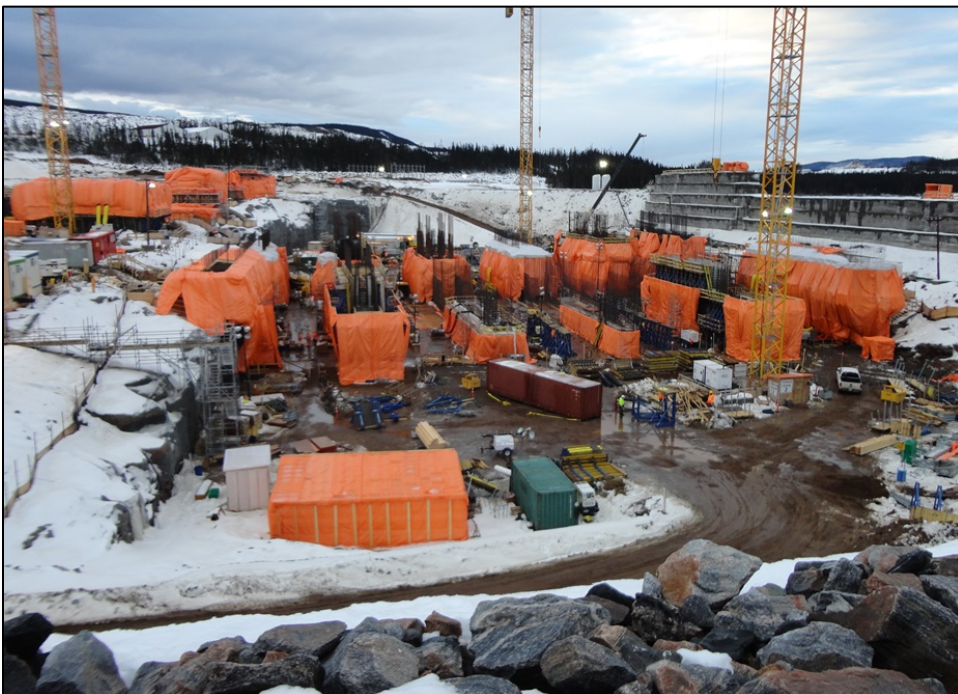
Photo 7.2: Spillway; view looking upstream towards the piers. RCC cofferdam is visible on the right side and the orange tarp covered transition dam is on the left. (November 25, 2014)
