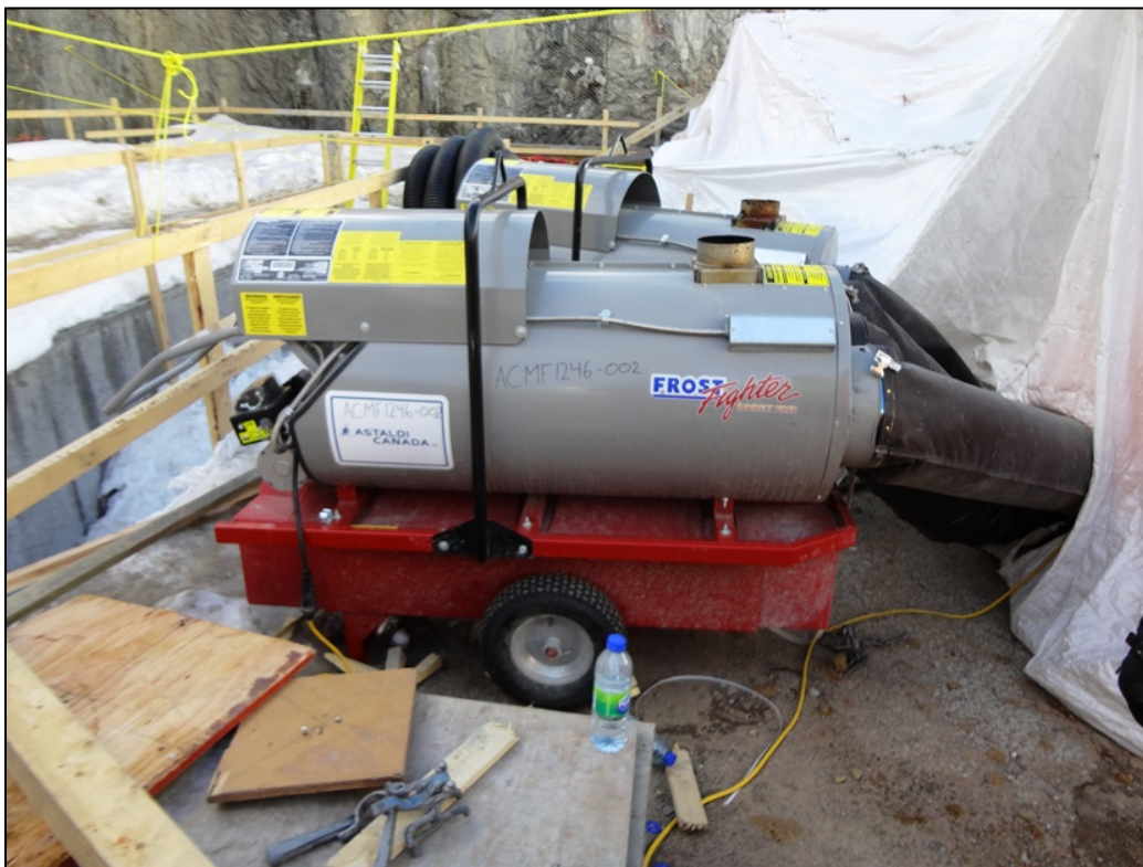
Photo 9.6: Backup heating plants for the north service bay foundation works. (November 26, 2014)
