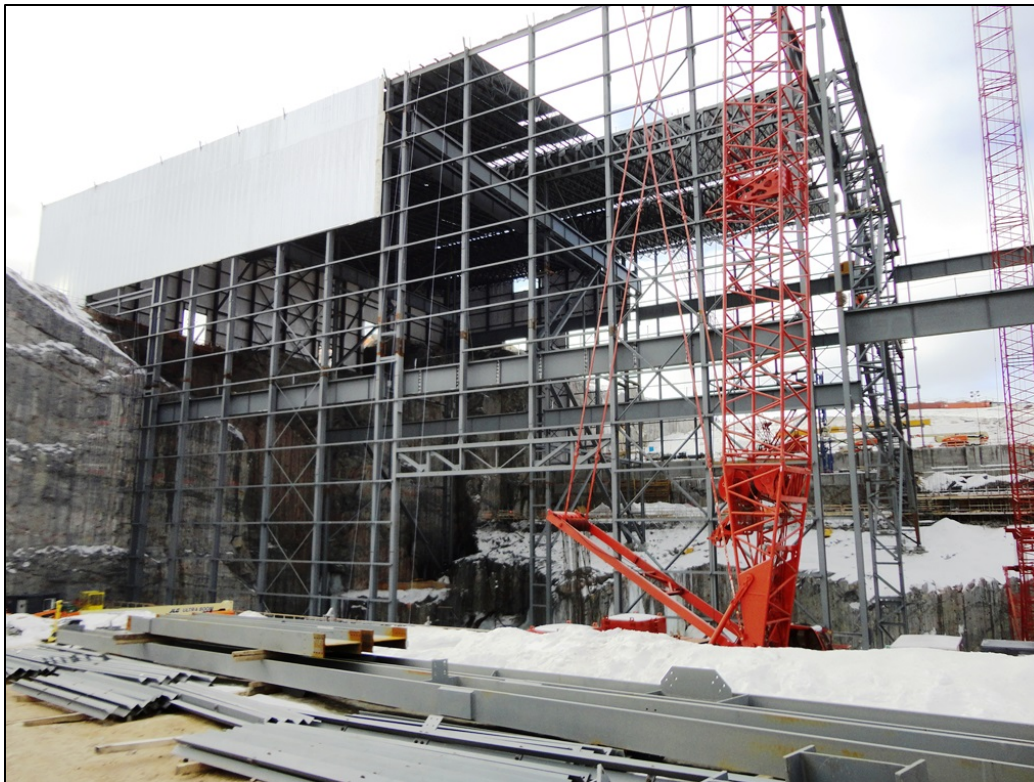
Photo 8.3: View looking upstream at the ICS construction over Units 1 and 2. (November 26, 2014)
