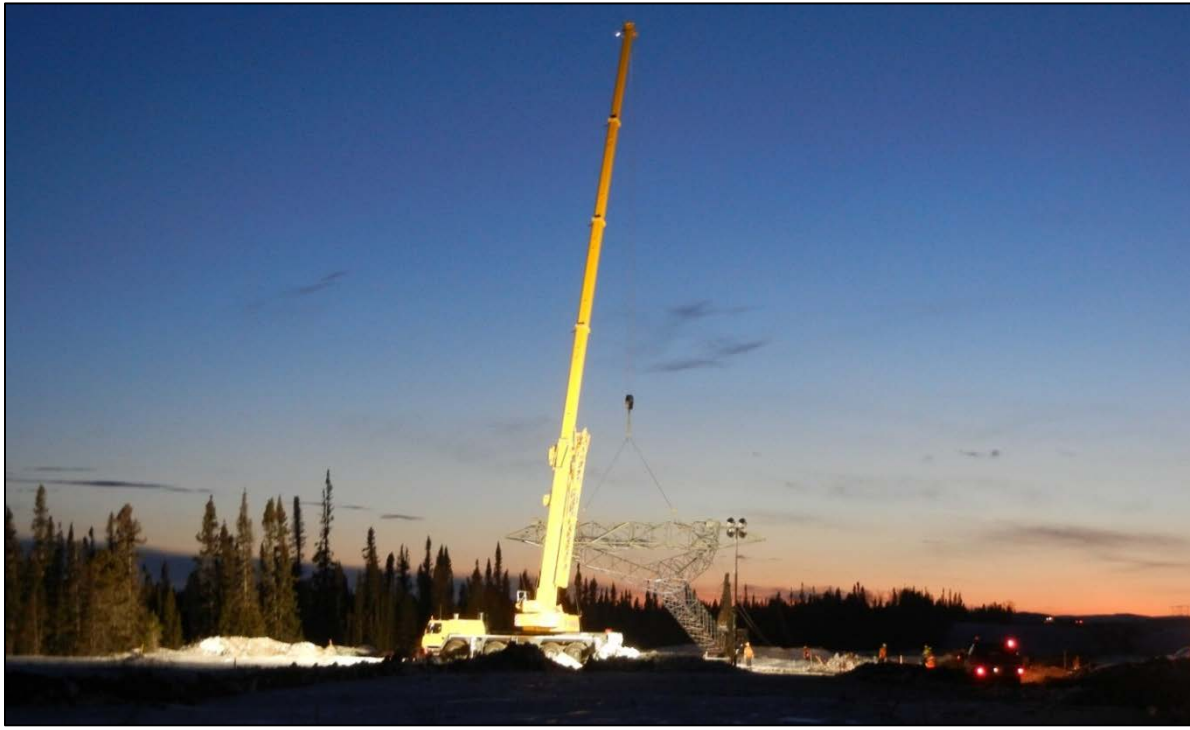
Photo 4.1: HVac transmission line – structure erection. (November 26, 2014)
