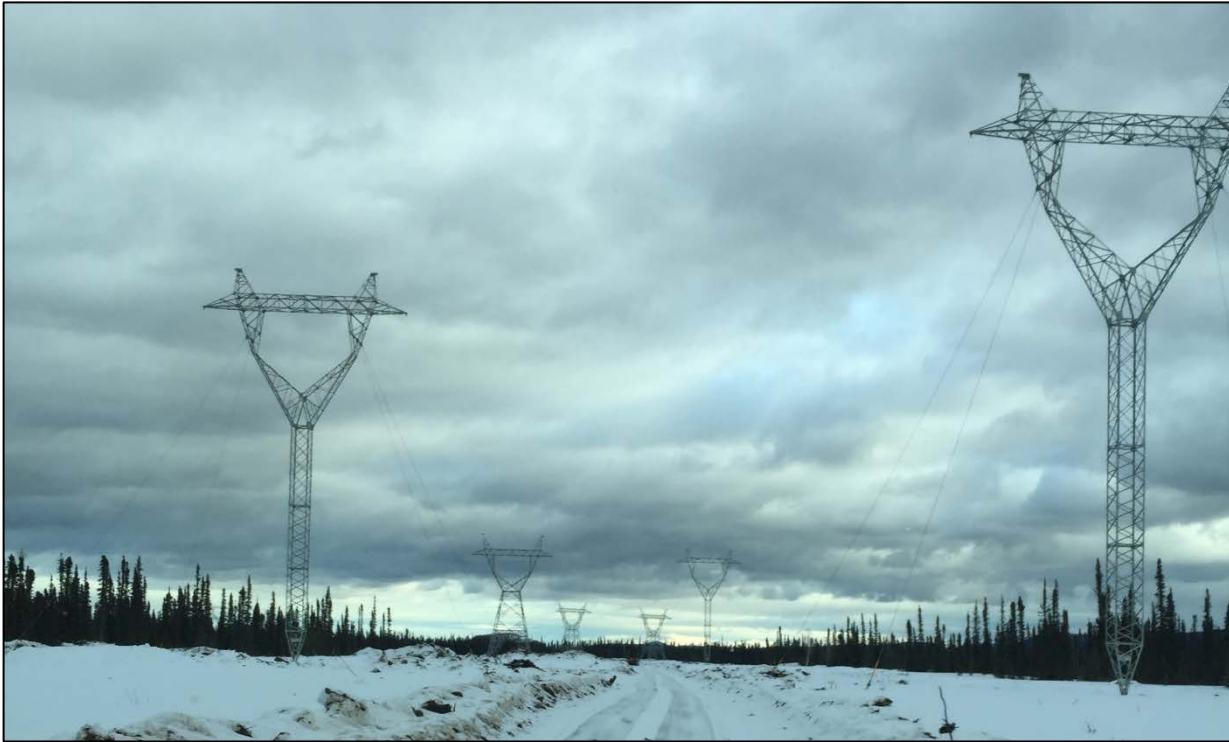
Photo 5.1d: Hvac transmission line – erected structures – Looking South toward both Lines, (November 26, 2014)
