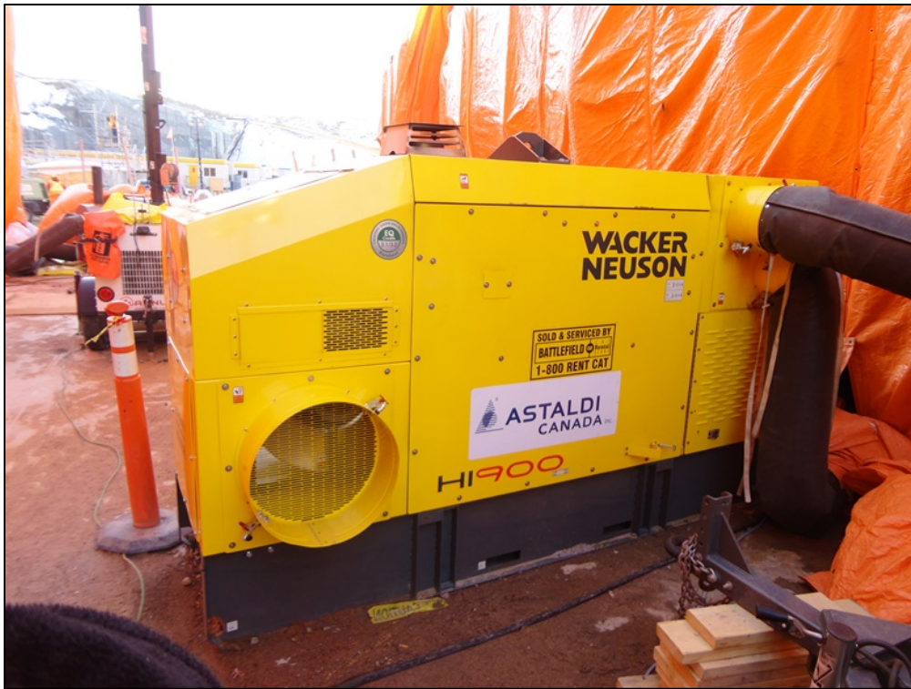
Photo 7.7: Spillway; Wacker Neuson heater, one of many used for heating the formwork and concrete pours of the piers. (November 26, 2014)
