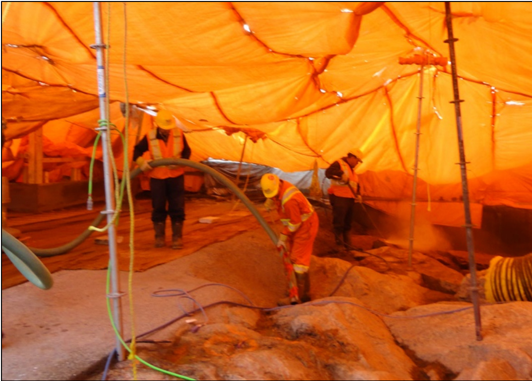
Photo 9.3: Powerhouse north service bay foundation. Cleaning the rock surface with an air vacuum and water jet. (November 26, 2014)
