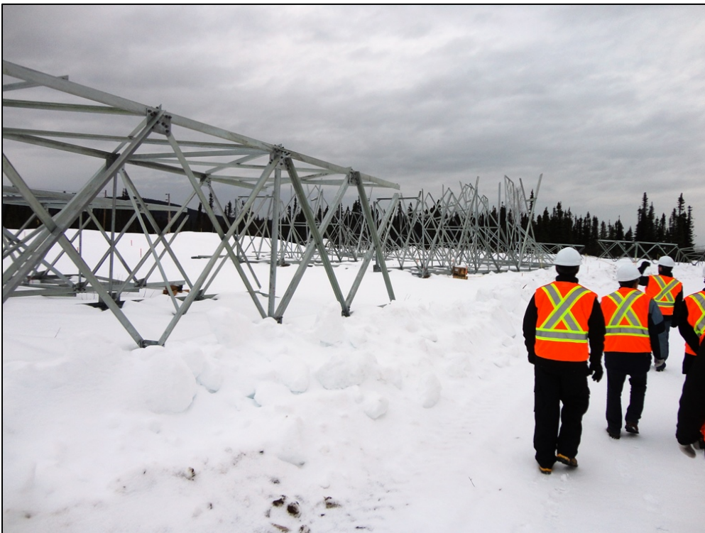
Photo 3.2: Assembling a HVAC transmission tower near the North Spur. (November 25, 2014)
