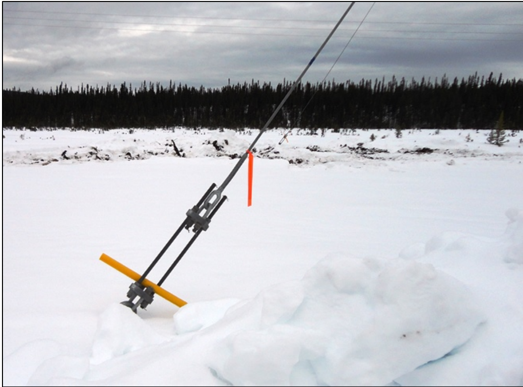
Photo 4.3: Lower connection of guy cable on single footing transmission tower. (November 26, 2014)
