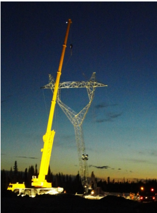
Photo 4.2 a (left) and b (right) : Erection of HVac Transmission Tower 58 at sundown. (a) tower being hoisted into place with crane and excavator and (b) in final position, still suspended from the crane; note untethered guy wires at this stage of erection. (November 26, 2014)
