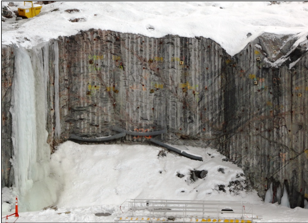
Photo 8.7: Powerhouse Bay 2. Photo shows the excellent quality of the blasting. (November 26, 2014)
