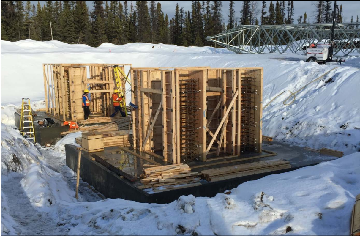
Photo 1.1 HVAC transmission line foundation installation. (November 25, 2014)
