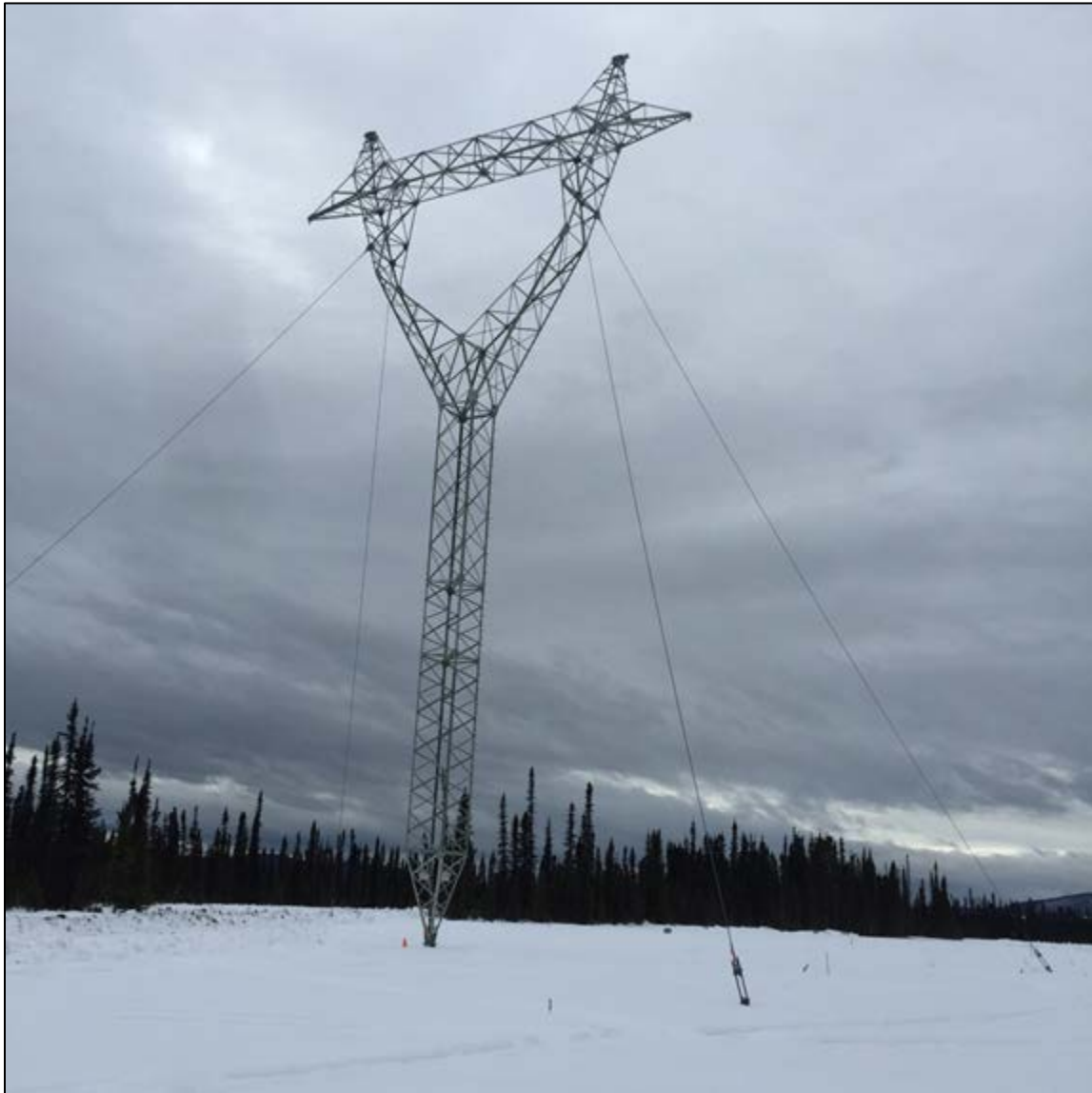
Photo 5.1a: HVac transmission line – erected guyed structure. (November 26, 2014)
