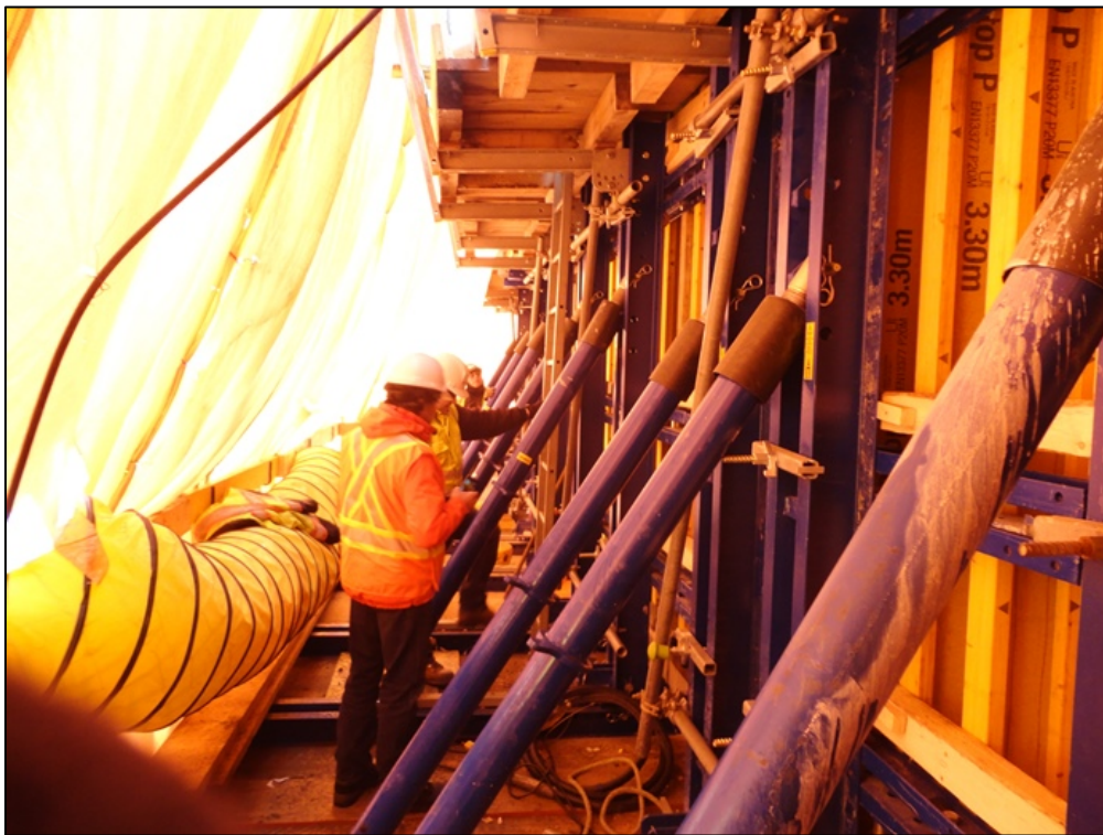
Pier .7.6: Spillway; shrouded and heated formwork. (November 26, 2014)
