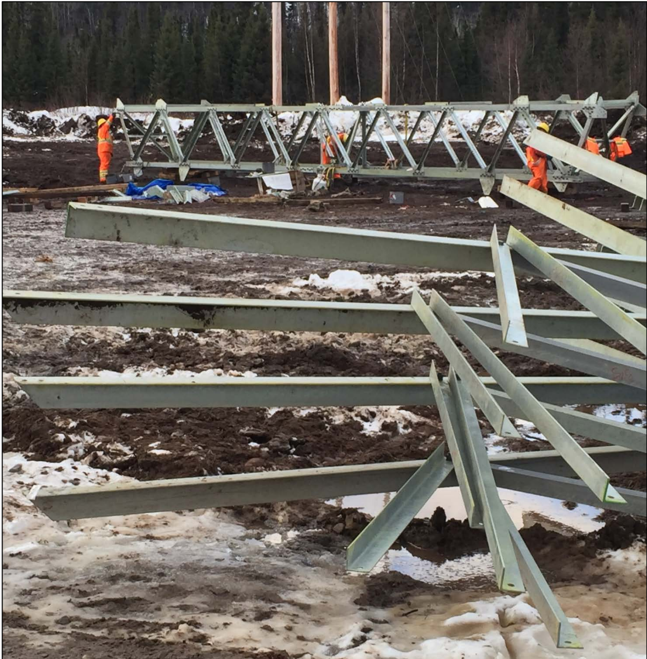
Photo 3.3: HVAC transmission line structure assembly. (November 25, 2014)
