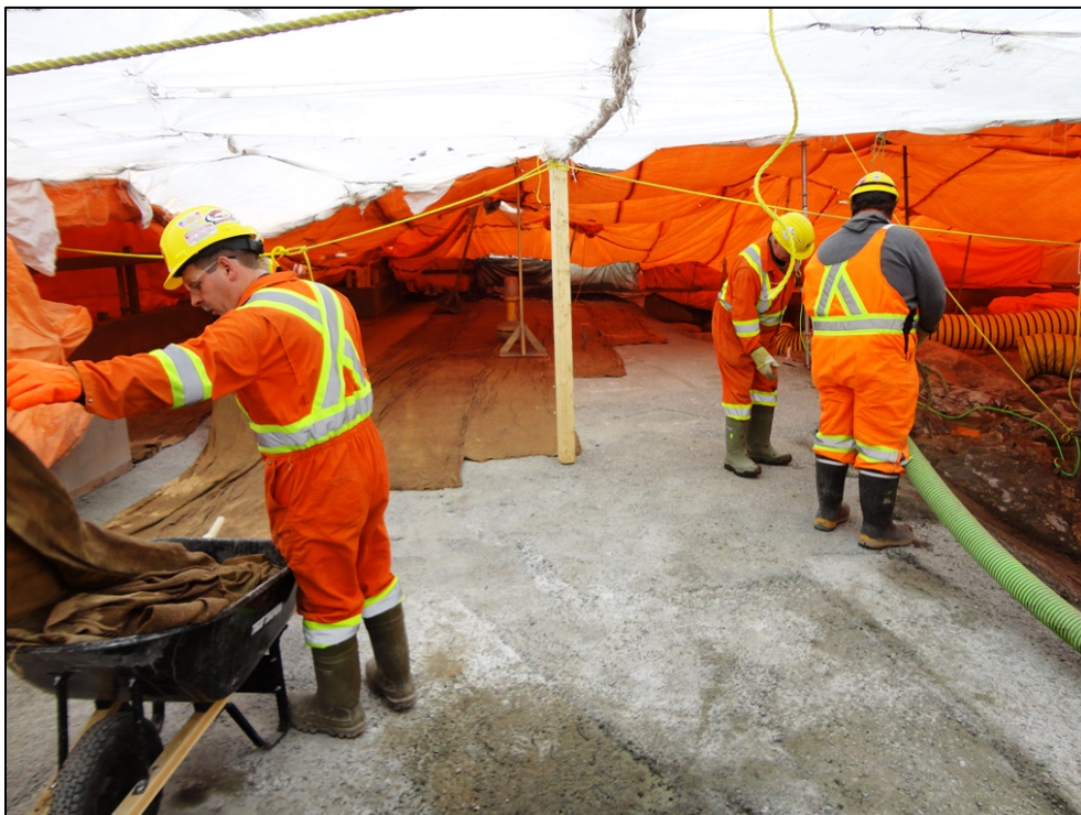
Photo 9.2: Powerhouse north service bay foundation. Note wetted burlap mats being placed on the surface of the base slab. (November 26, 2014)
