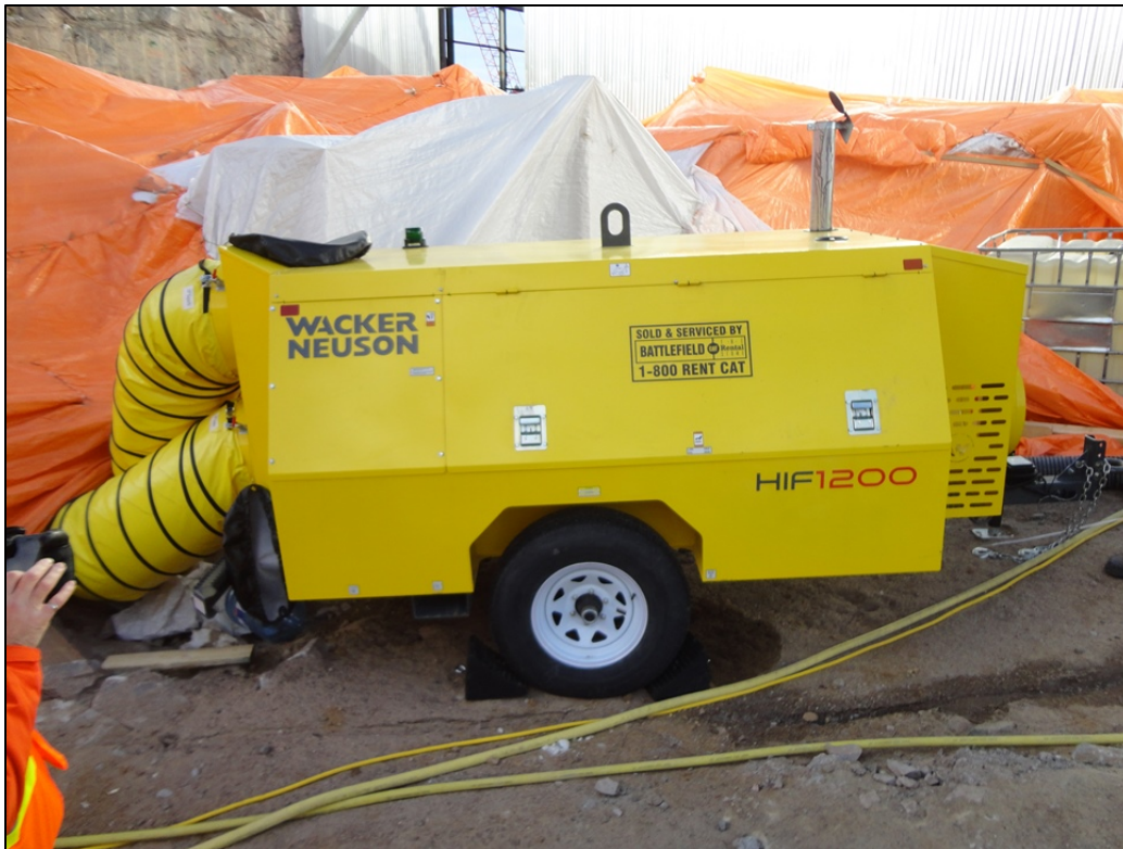
Photo 9.5: Wacker Neuson heating unit used for heating the works in the north service bay. (November 26, 2014)
