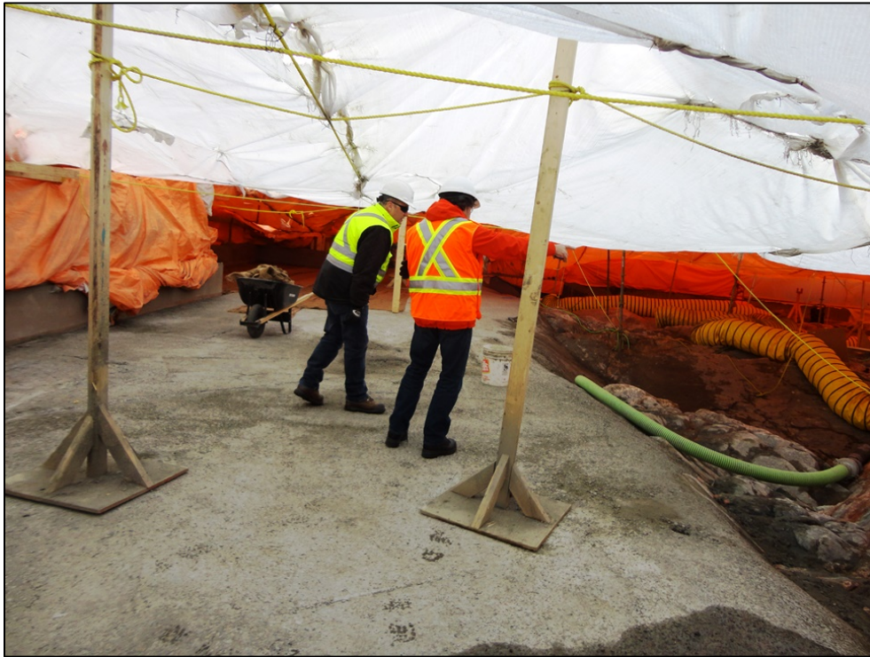
Photo 9.1: Powerhouse north service bay foundation. Recently poured base concrete. (November 26, 2014)
