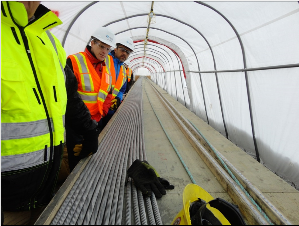
Photo 2.1: Laydown and preparation of guy cables for HVac transmission towers. (November 25, 2014)
