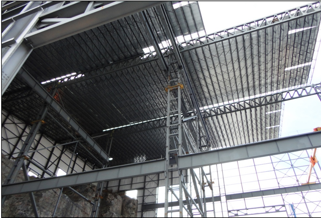
Photo 8.5: Powerhouse ICS Roof over Units 1 and 2. (November 26, 2014)
