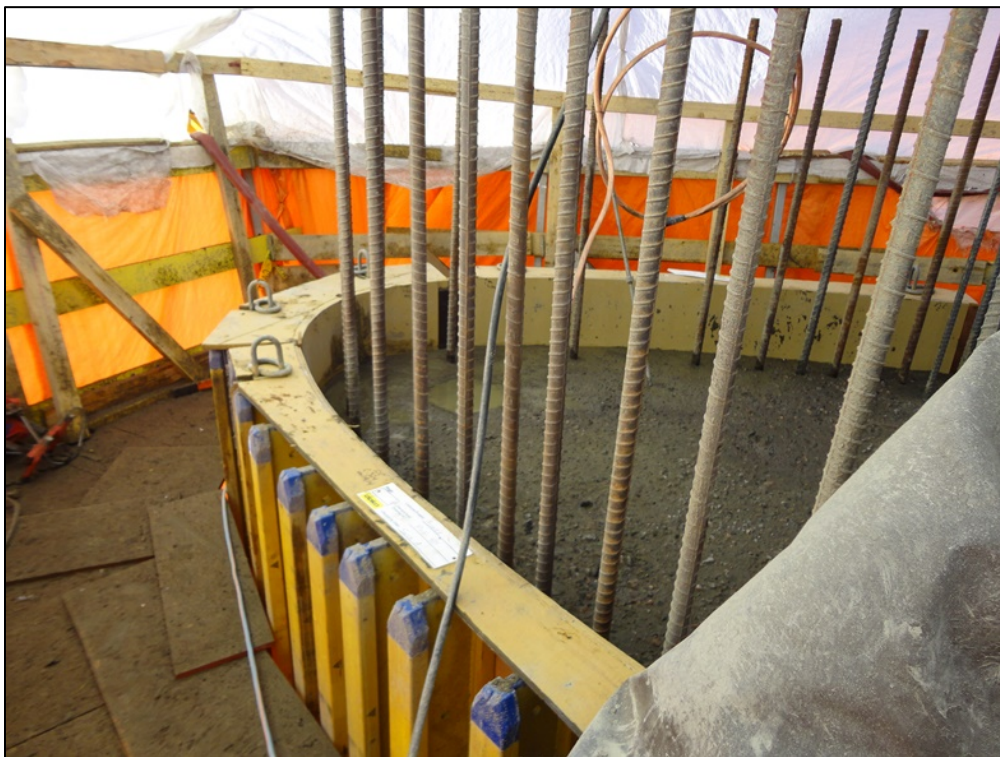
Photo 7.8: Spillway; Upstream nose of Pier 3. (November 26, 2014)
