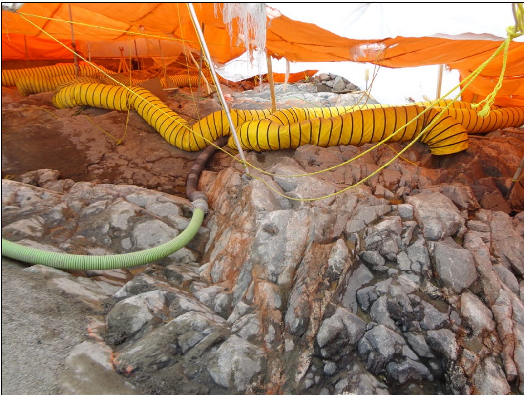
Photo 9.4: Powerhouse north service bay foundation. Cleaned surface in blocky granitic gneiss. (November 26, 2014)
