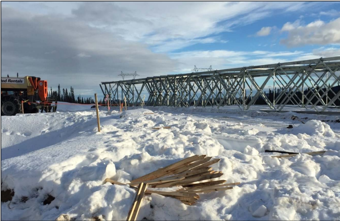
Photo 3.1: HVAC transmission line structure assembly. (November 25, 2014)
