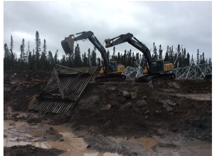
S1-70 Leg C, reclamation of grillage footing, saturated founding base and backfill
