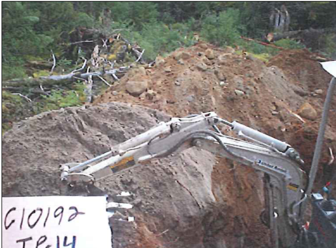
Figure 33: Sample test pit represented in the project Geotechnical Report. The test-pit spoil pile is dry, yet the test pit report notes “some water observed”.
