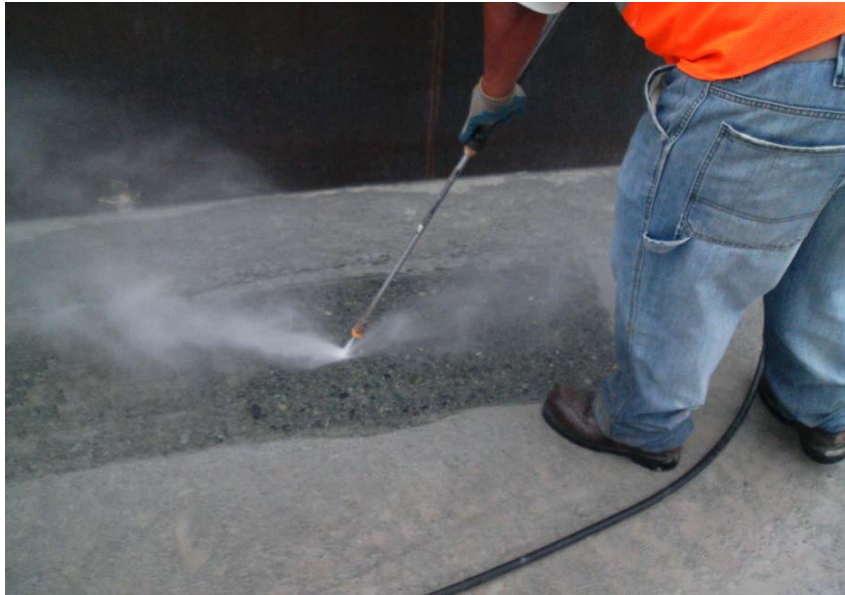
Figure 44: Green Cutting with Water Blasting (Portugues Dam-Test Section, PR, USA)
