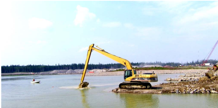
Figure 24: Underwater Excavation, Wuskwatium Generating Station, MB
