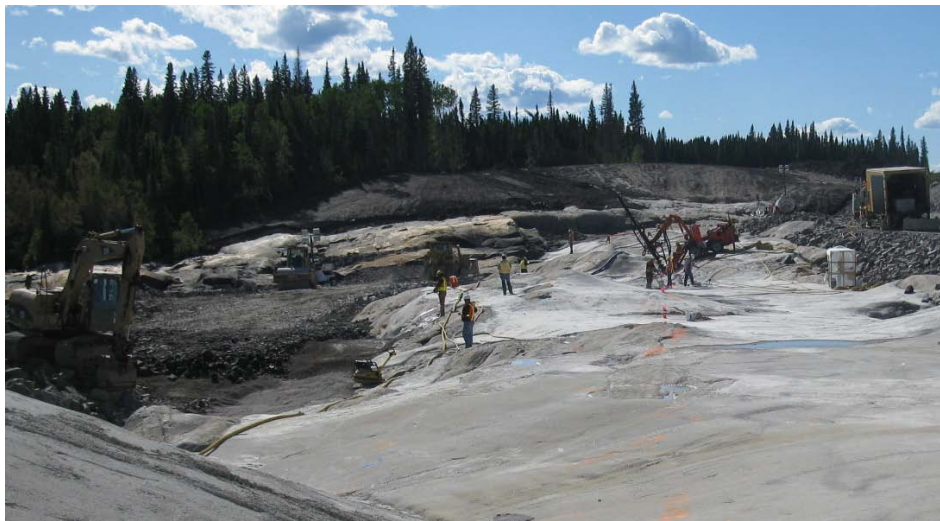
Figure 22: Foundation Prep of Main Dam, Wuskwatim, MB
