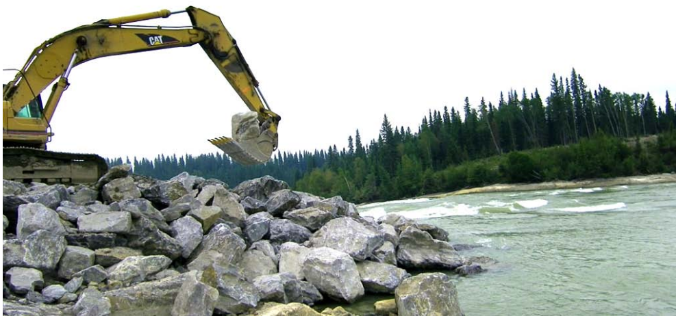
Figure 28: Building River Closure, Wuskwatim, MB
