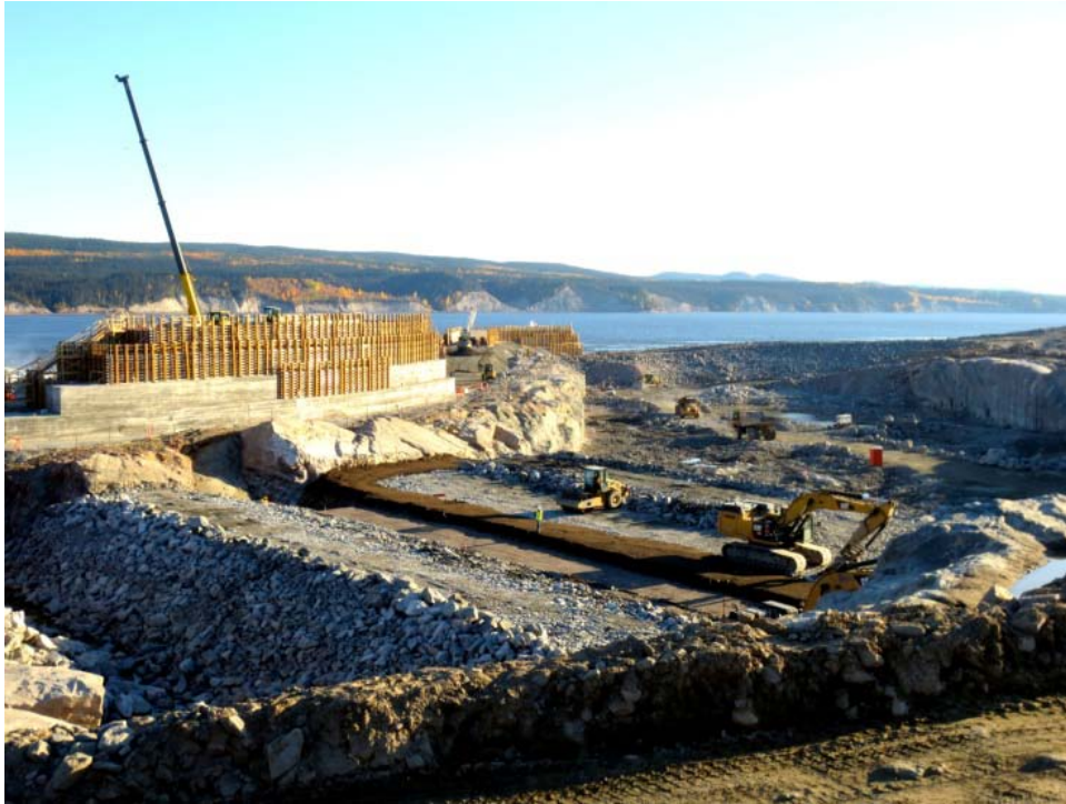
Figure 30: Earthfill Cofferdam Construction, Muskrat Falls, NL
