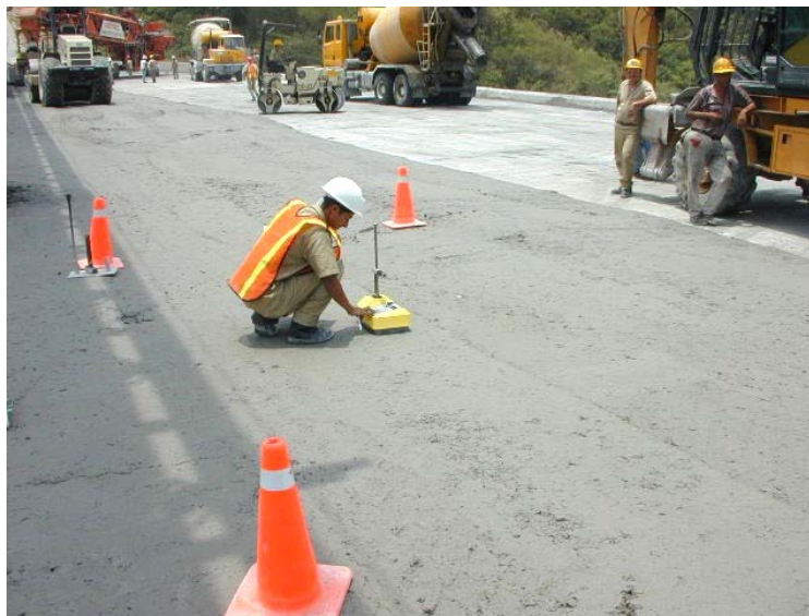
Figure 12: RCC Density Measurement (Porce II Dam, Colombia)
