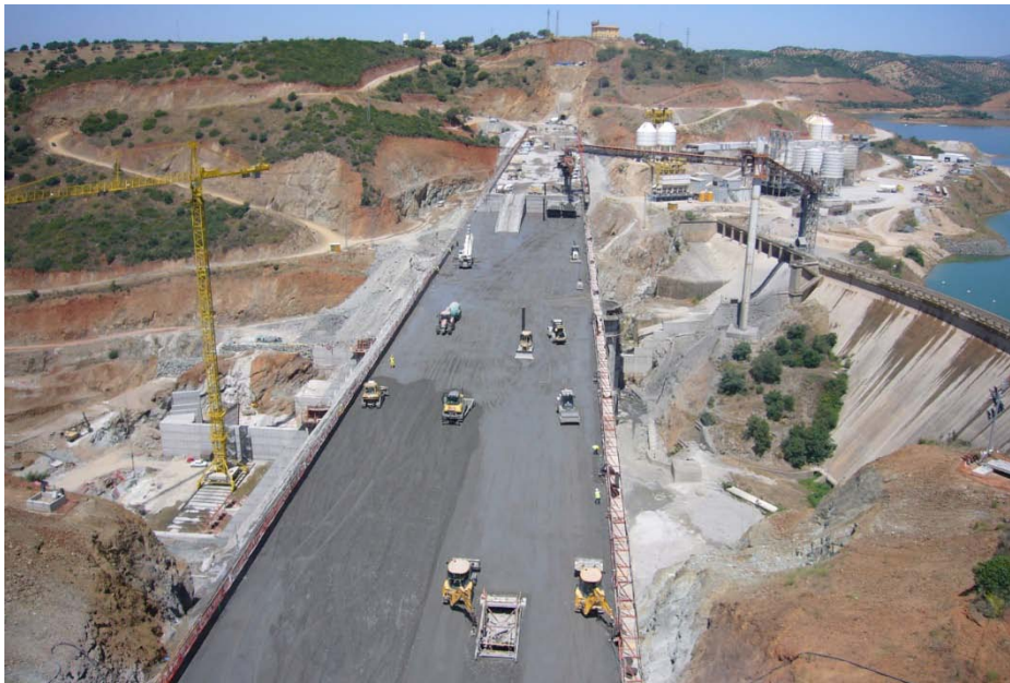
Figure 32: Split-level Placement Method Implemented at La Breña II Dam in Spain (2007-2008)
