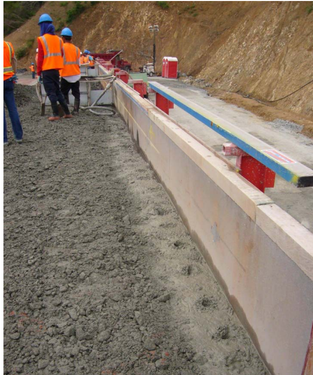
Figure 42: GERCC after Vibration (Portugues Dam-Test Section, PR, USA)
