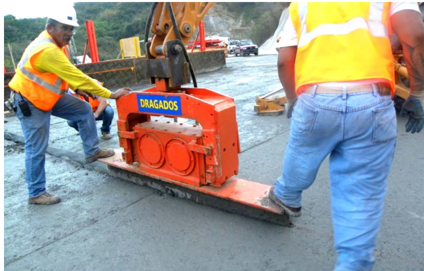
Figure 40: Transverse Joint Cutting with Vibrating Plate (Portugues Dam-Test Section, PR, USA)
