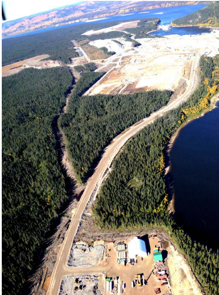
Figure 21: Site Roads at Muskrat Falls
