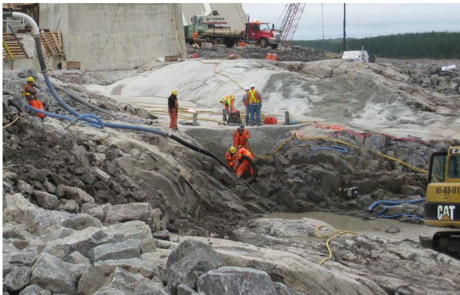
Figure 36: Dental Concreting of Uneven Foundation (Wuskwatim Generating Station, MB)
