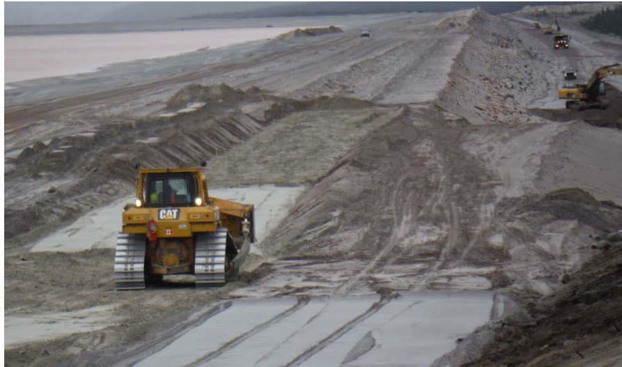
Figure 29: Earthfill Dam construction, Mont Wright, QC.
