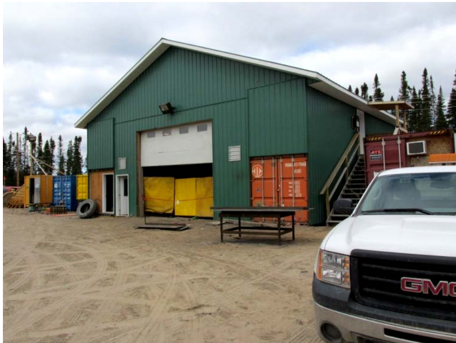
Figure 18: Welding Facility at the Muskrat Falls site
