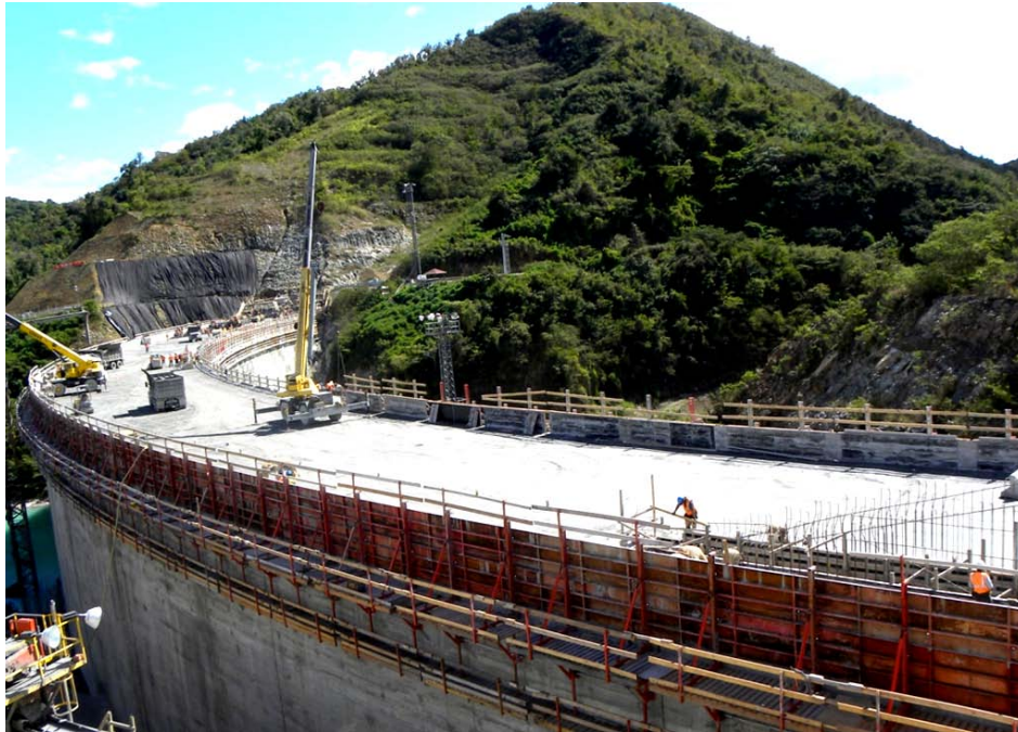
Figure 38: Upstream Formwork (Portugues Dam, PR, USA)
