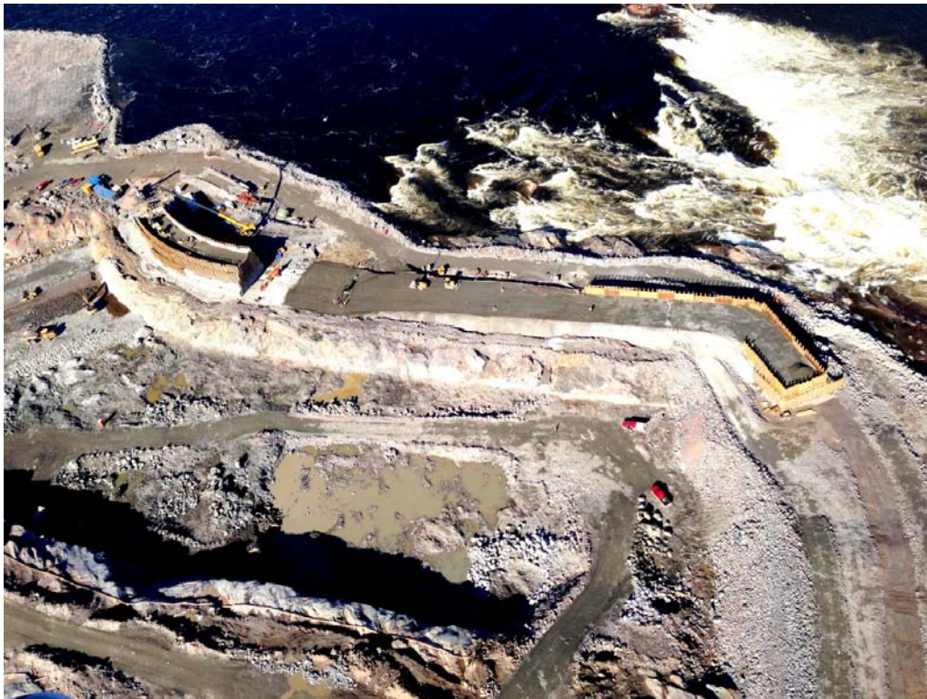
Figure 23: RCC Cofferdam to be removed
