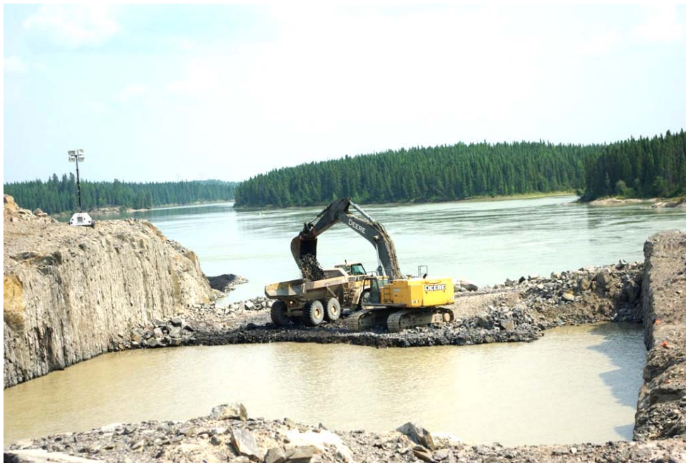
Figure 26: Downstream Rock Plug Removal, Wuskwatim Generating Station, MB
