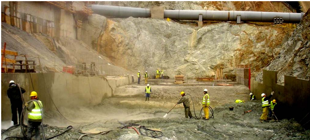
Figure 35: Foundation Clean-up (La Breña II Dam, Spain)
