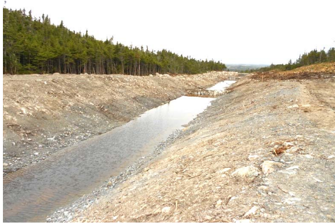
Figure 10: Trench with Rock Check Dam, Sandy Pond, Long Harbour site, NL
