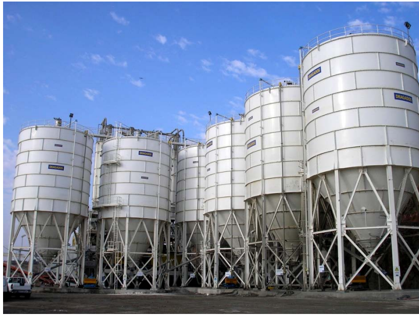
Figure 6: 6 x 1000 t Silos at La Breña II Dam, Spain
