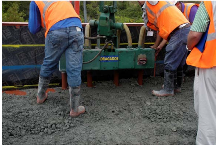
Figure 41: Vibrating GERCC (Portugues Dam-Test Section, PR, USA)
