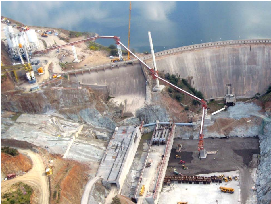
Figure 1: RCC Conveyors at La Breña II Dam, Spain
