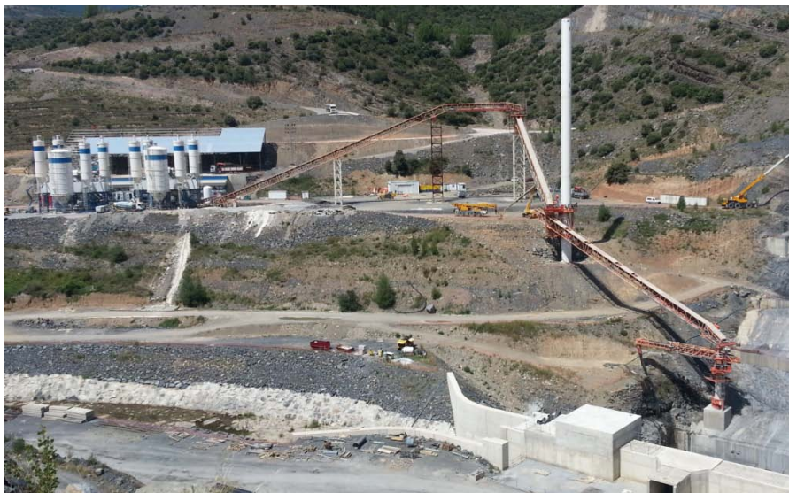
Figure 39: Concrete Plant and Conveyors at Enciso Dam, Spain, currently under construction
