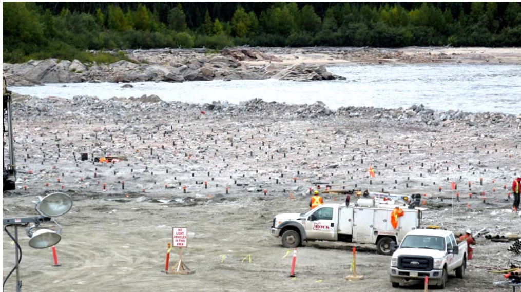
Figure 17: Drill holes ready for Blasting at Muskrat Falls site
