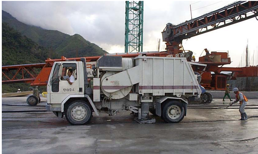
Figure 45: Excess Water Removal with Vacuum Truck (Porce II Dam, Colombia)
