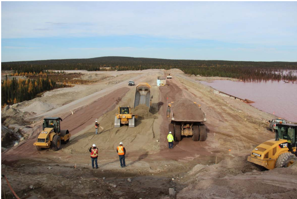
Figure 47: Earthfill Dam Construction, Mont Wright, QC
