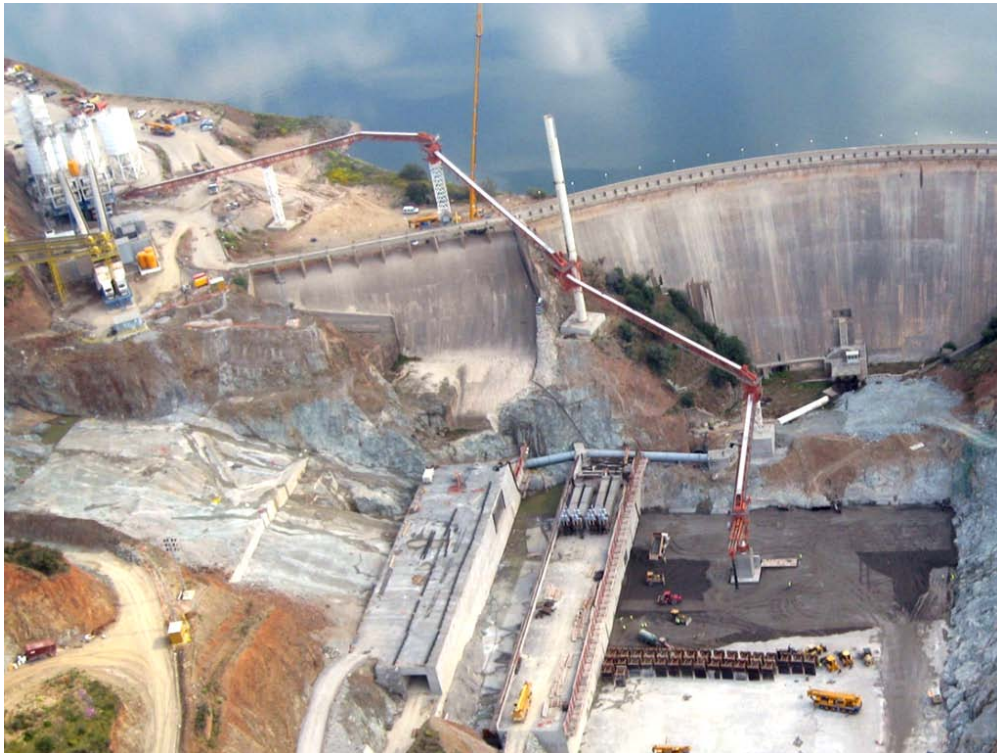
Figure 46: RCC Conveyors at La Breña II Dam, Spain
