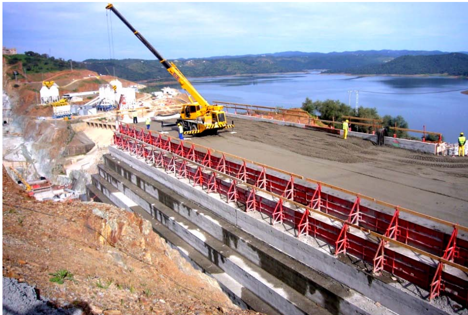
Figure 37: Downstream Formwork (La Breña II Dam, Spain)
