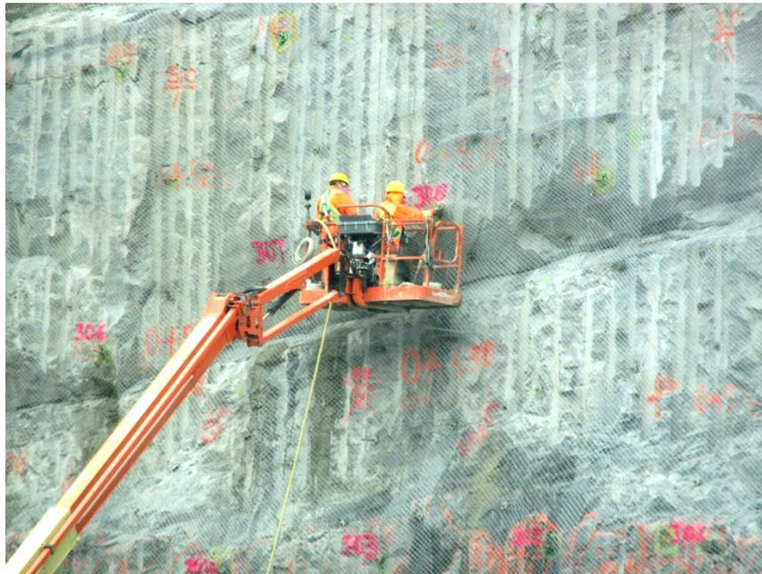
Figure 27: Rock Bolts being Installed, Muskrat Falls, NL
