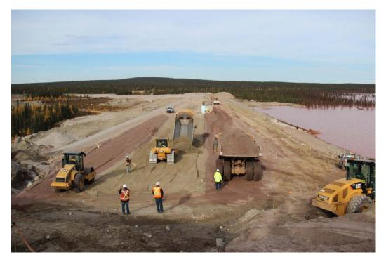
Figure 47: Earthfill Dam Construction, Mont Wright, QC
