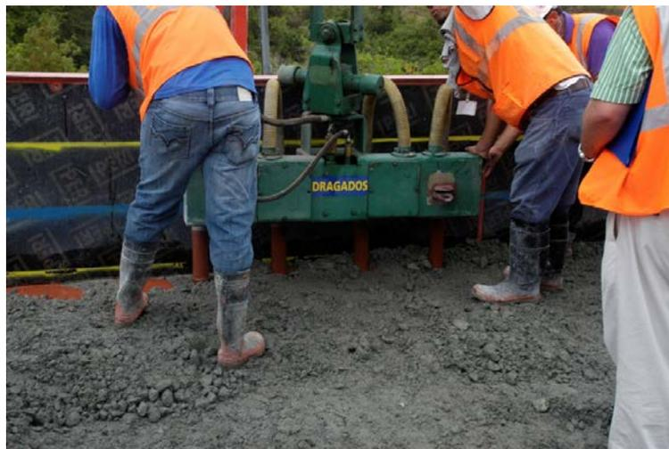
**Figure 41: Vibrating GERCC (Portugues Dam-Test Section, PR, USA)**
