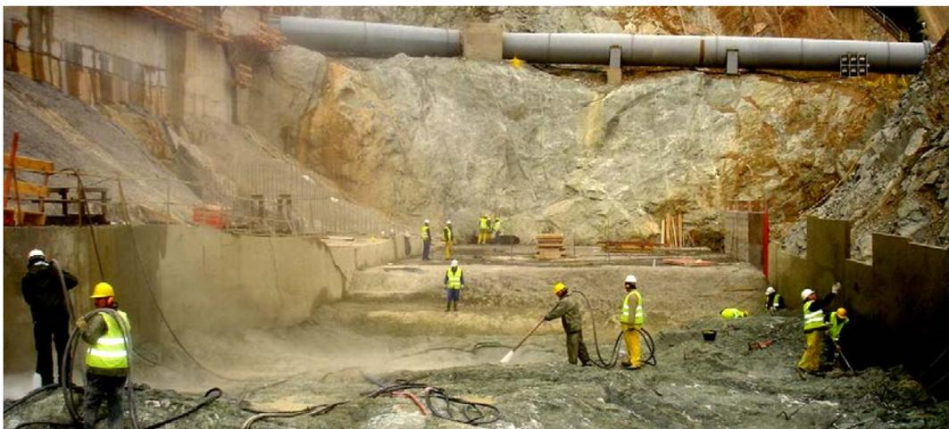
Figure 35: Foundation Clean-up (La Breña II Dam, Spain)
