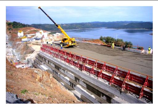
Figure 37: Downstream Formwork (La Breña II Dam, Spain)
