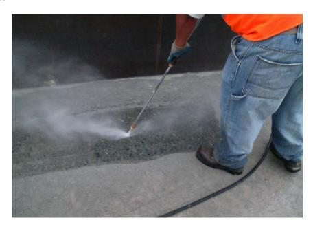
Figure 44: Green Cutting with Water Blasting (Portugues Dam-Test Section, PR, USA)
