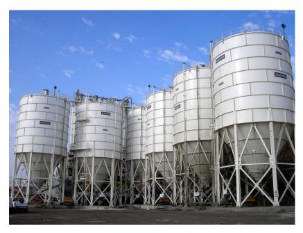
Figure 6: 6 x 1000 t Silos at La Breña II Dam, Spain
