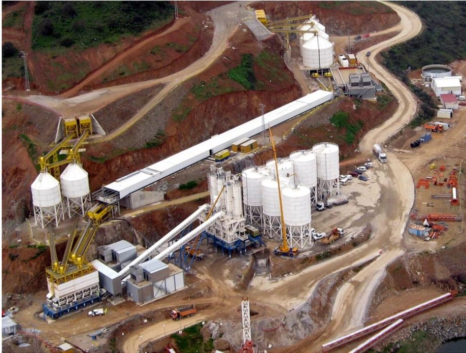
**Figure 5: Concrete Plant (La Breña II Dam, Spain)**
