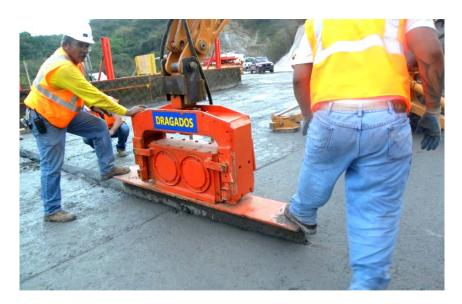
Figure 40: Transverse Joint Cutting with Vibrating Plate (Portugues Dam-Test Section, PR, USA)
