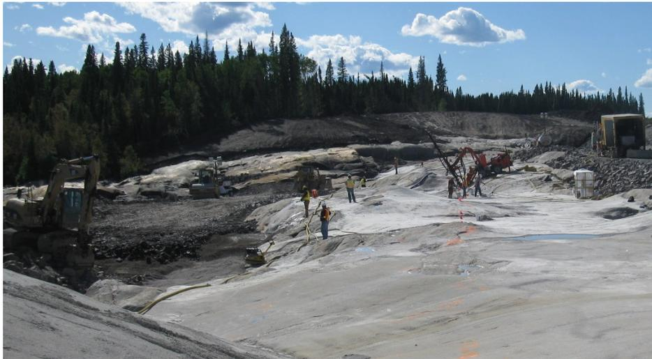
Figure 22: Foundation Prep of Main Dam, Wuskwatim, MB
