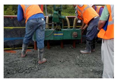
Figure 41: Vibrating GERCC (Portugues Dam-Test Section, PR, USA)
