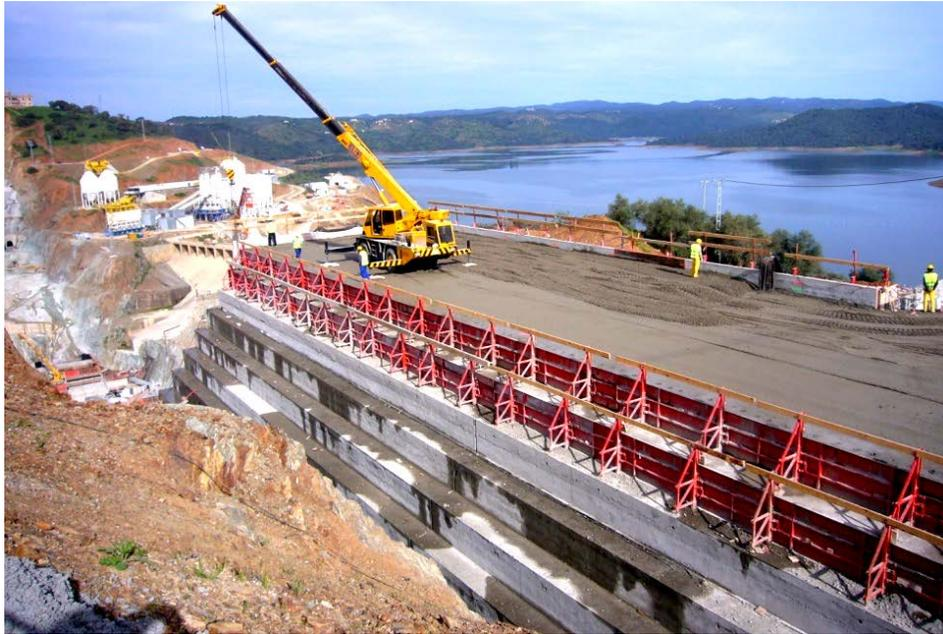
**Figure 37: Downstream Formwork (La Breña II Dam, Spain)**
