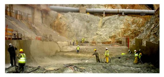
Figure 35: Foundation Clean-up (La Breña II Dam, Spain)
