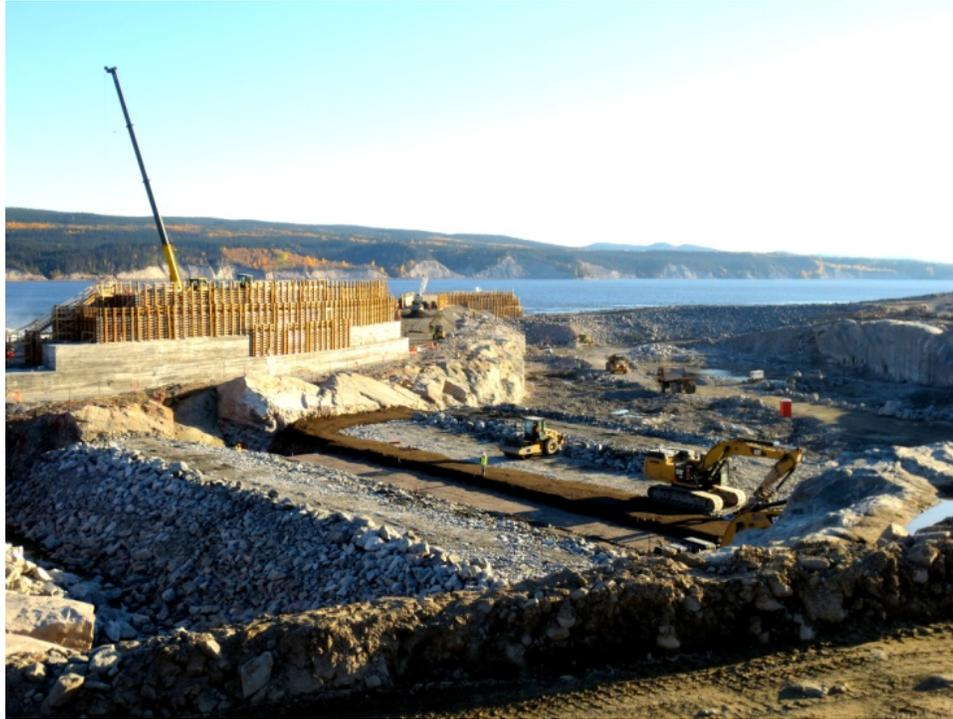
Figure 30: Earthfill Cofferdam Construction, Muskrat Falls, NL
