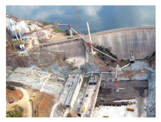
Figure 46: RCC Conveyors at La Breña II Dam, Spain
