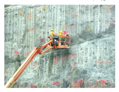
Figure 27: Rock Bolts being Installed, Muskrat Falls, NL
