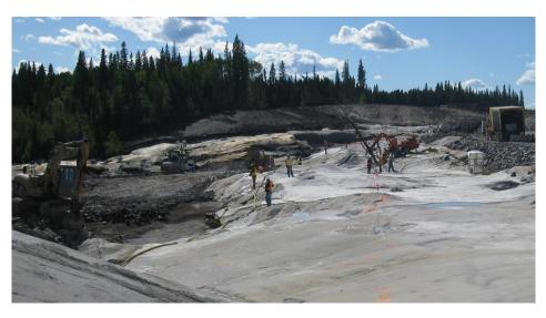
Figure 22: Foundation Prep of Main Dam, Wuskwatim, MB
