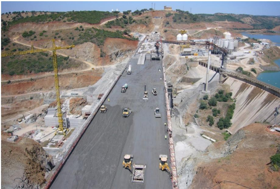
**Figure 32: Split-level Placement Method Implemented at La Brena II Dam in Spain (2007-2008)**
