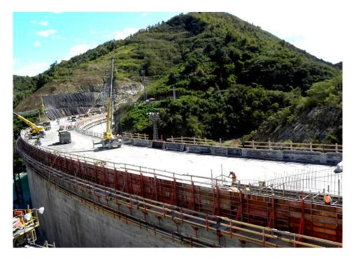
Figure 38: Upstream Formwork (Portugues Dam, PR, USA)
