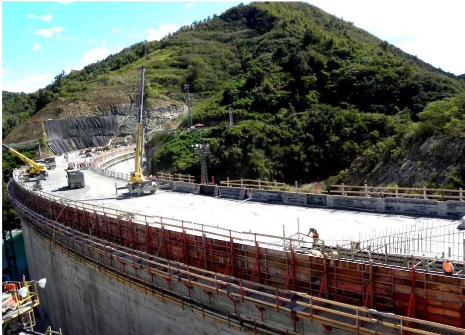
**Figure 38: Upstream Formwork (Portugues Dam, PR, USA)**
