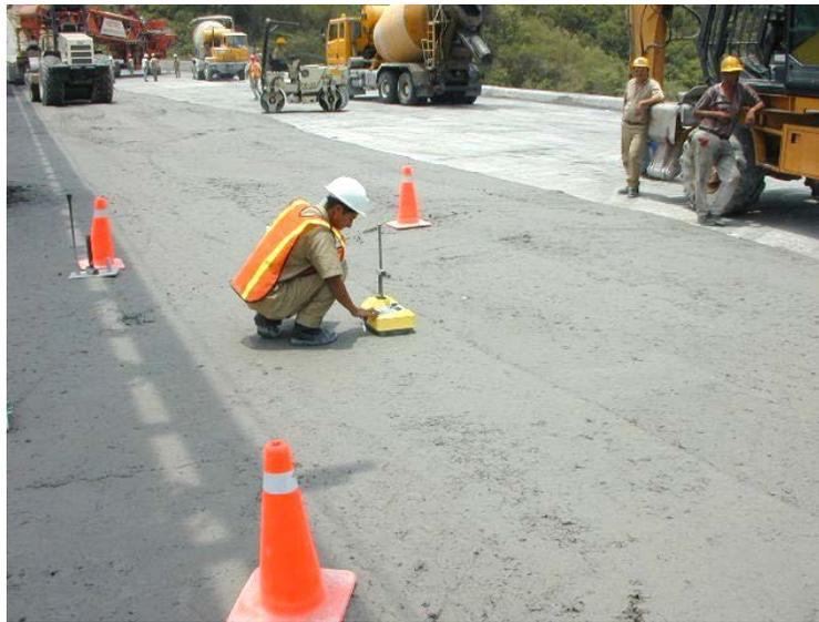
Figure 12: RCC Density Measurement (Porce II Dam, Colombia)
