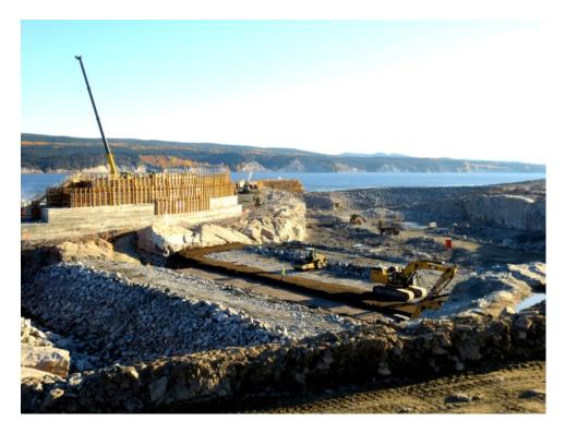
Figure 30: Earthfill Cofferdam Construction, Muskrat Falls, NL
