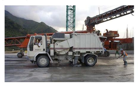
Figure 45: Excess Water Removal with Vacuum Truck (Porce II Dam, Colombia)
