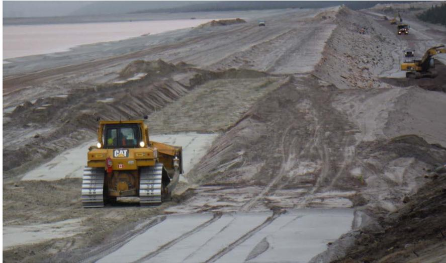
Figure 29: Earthfill Dam construction, Mont Wright, QC.
