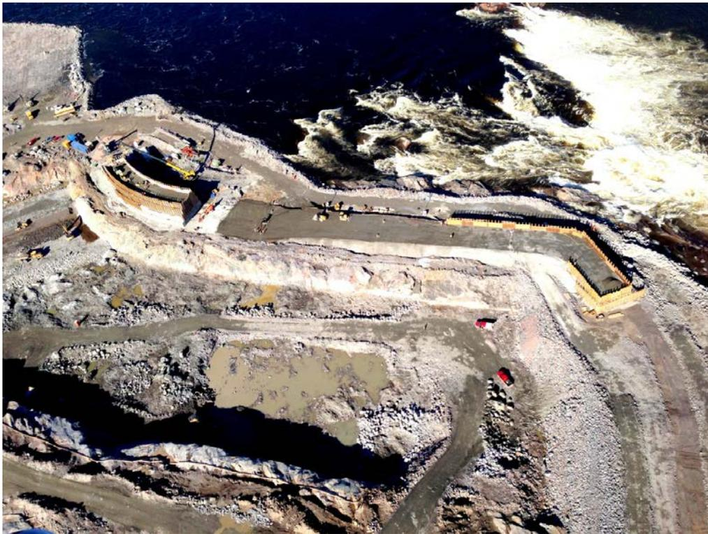
Figure 23: RCC Cofferdam to be removed
