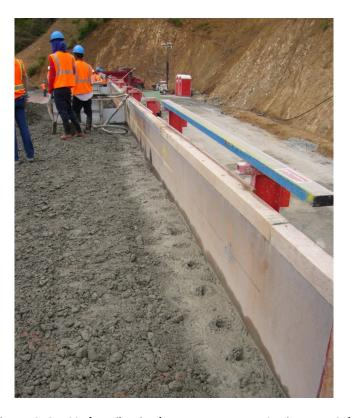
Figure 42: GERCC after Vibration (Portugues Dam-Test Section, PR, USA)
