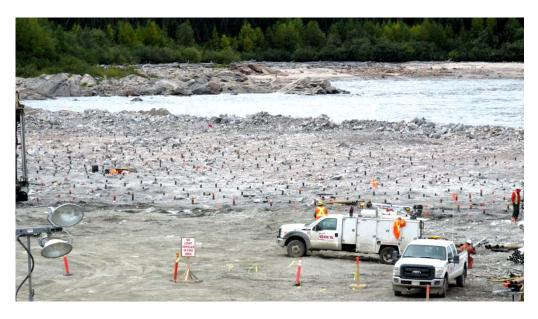
Figure 17: Drill holes ready for Blasting at Muskrat Falls site
