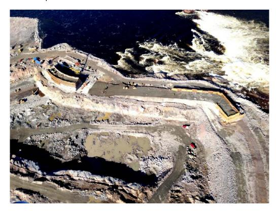
Figure 23: RCC Cofferdam to be removed
