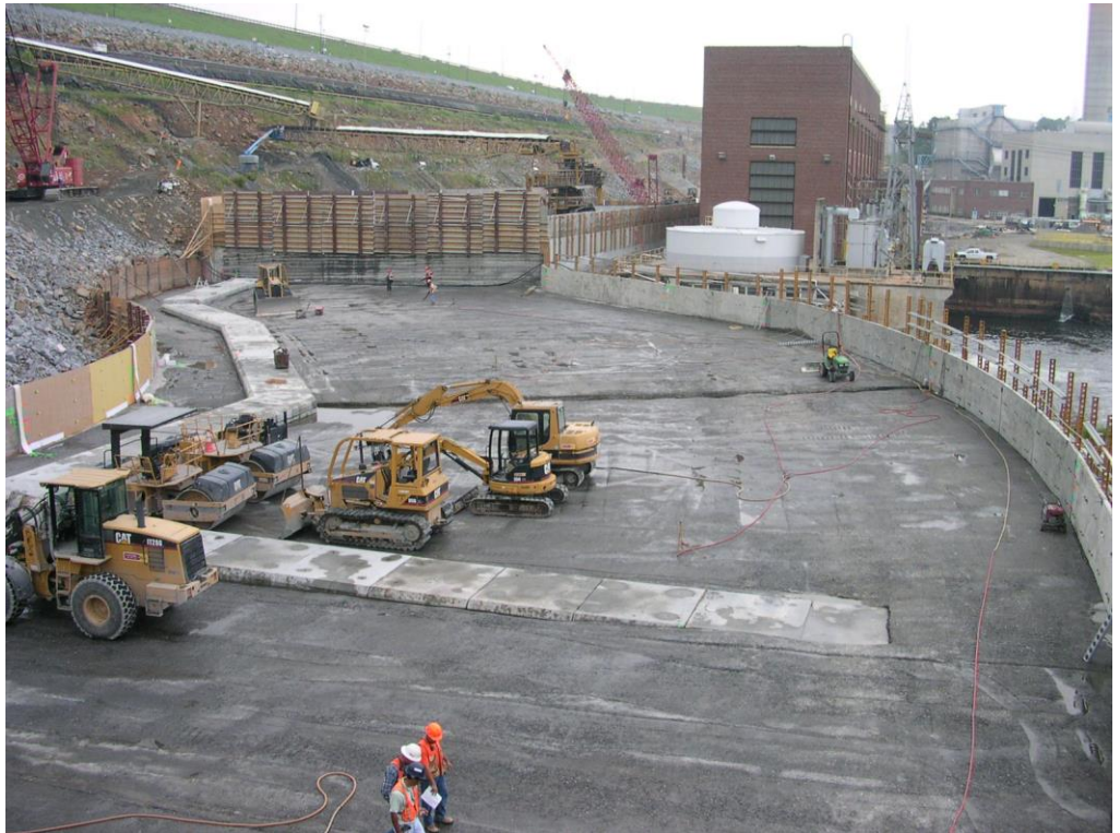
Typical joint preparation of warm joints
