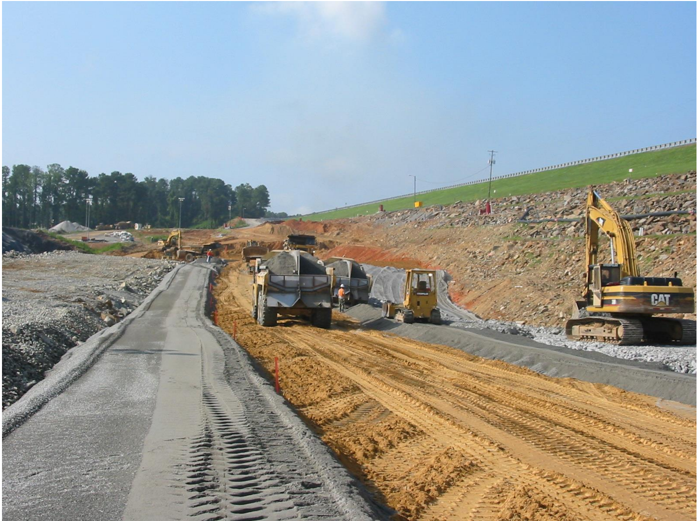
Multi-zone placement at Saluda Dam
