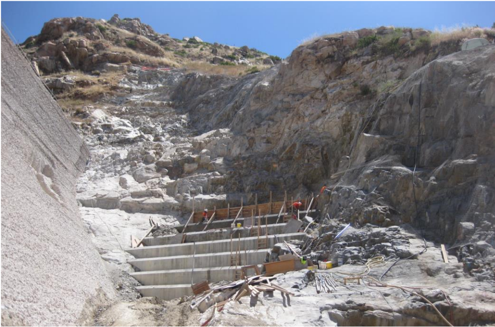
Levelling concrete on the left abutment at San Vicente Dam
