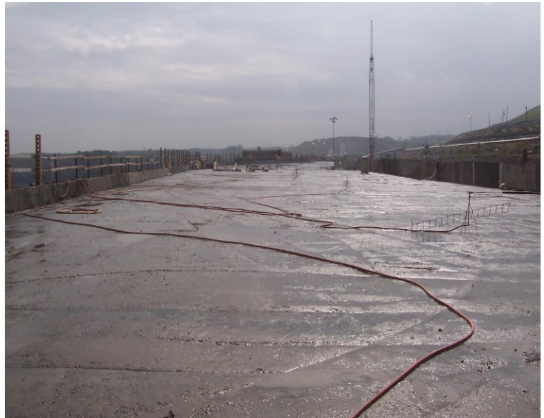
Proper curing of an RCC lift surface.
