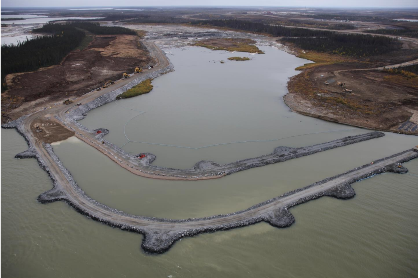
Keyask Powerhouse Cofferdam, Dual Groin, September 2014
