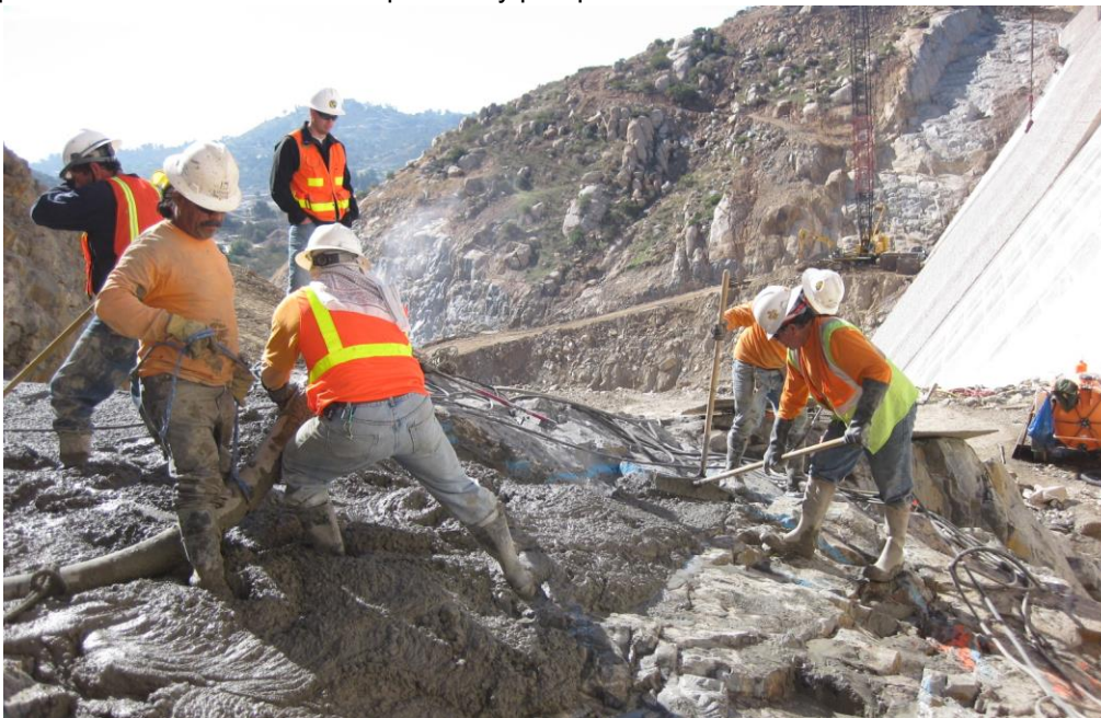
Dental concrete crew on the San Vicente Dam
