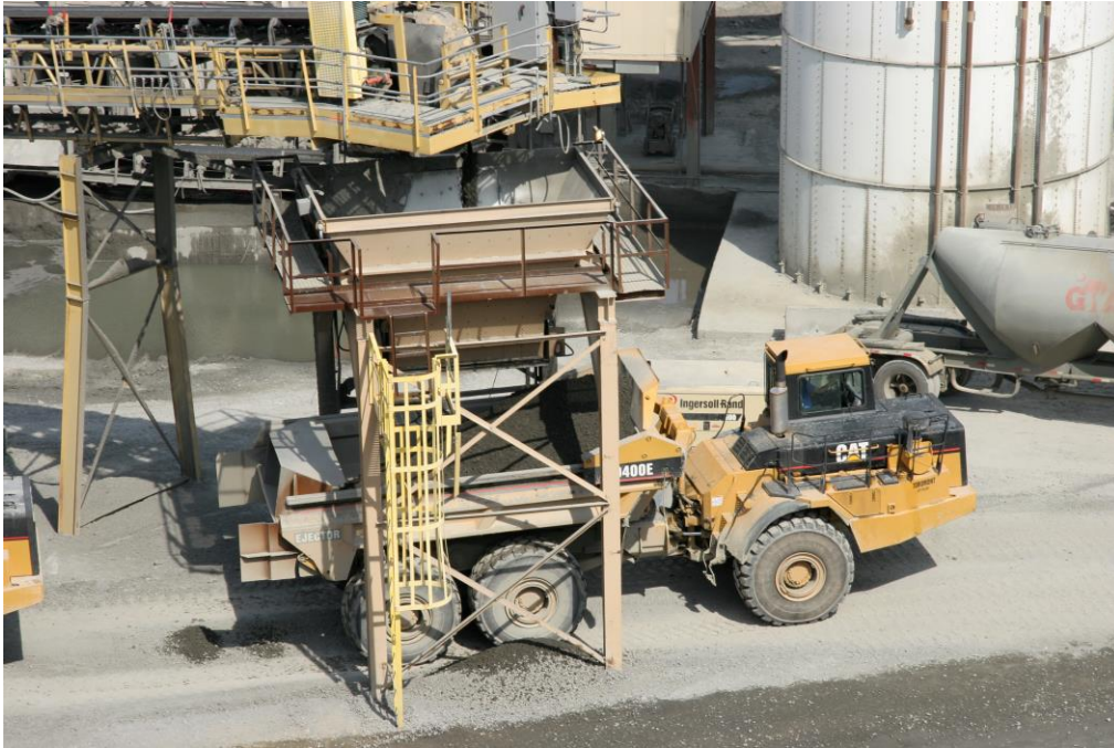
A gob hopper loads a haul truck from the RCC plant at the Saluda Dam Project
