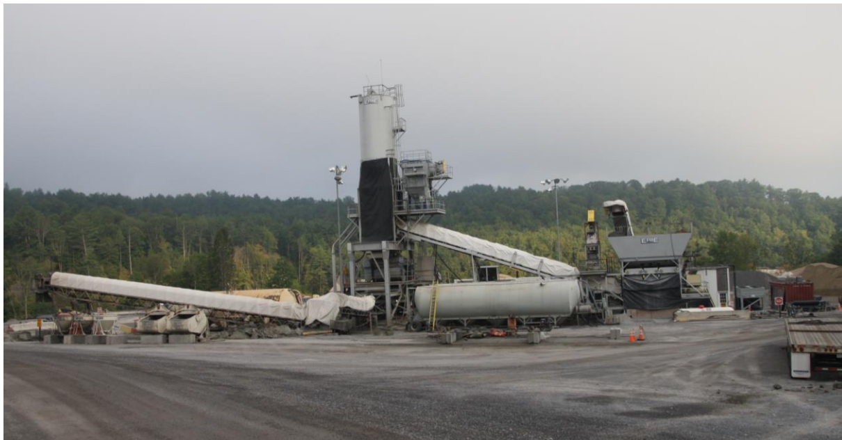
Single Plant – Dual Mix Capability at Barnard’s Gilboa Dam Project, New York
