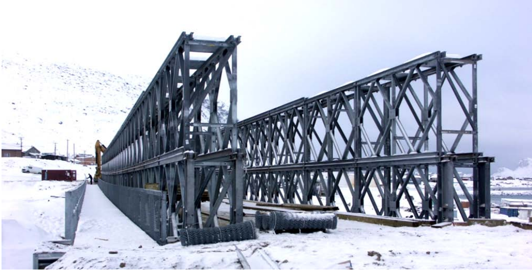
Figure 1: Spillway Bridge, Long-Sault Rapids, ON (Algonquin Bridge)
