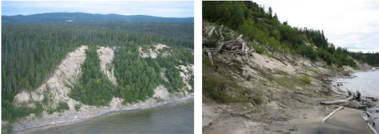
Figure 1-2: Instabilities along the North Spur
