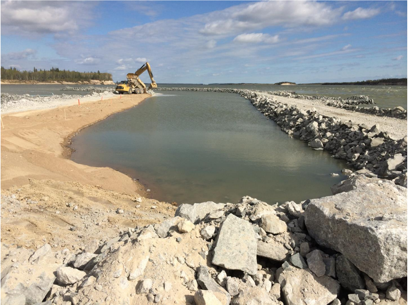
Transition Placement on Dual Groin Cofferdam at Keeyask, August 2014
