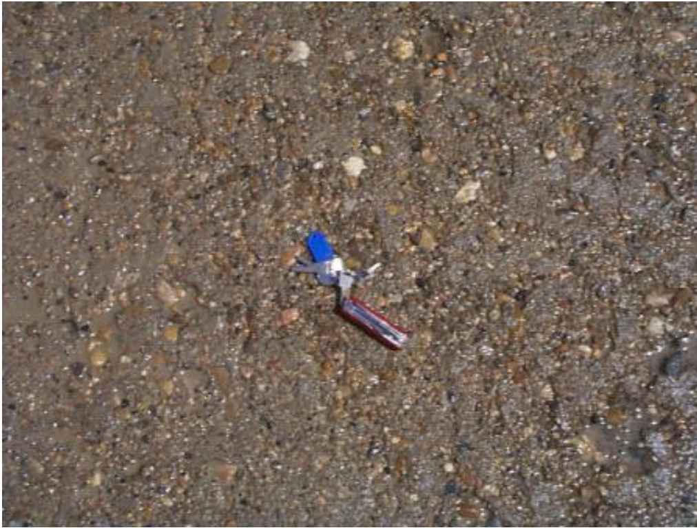
Typical surface of a treated cold joint
