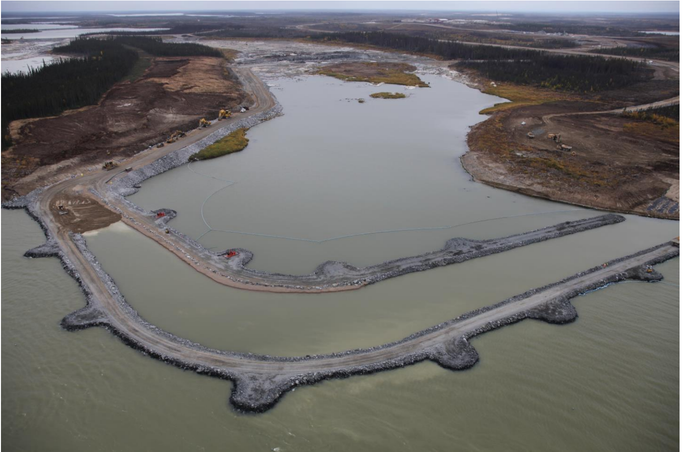
Keyask Powerhouse Cofferdam, Dual Groin, September 2014
