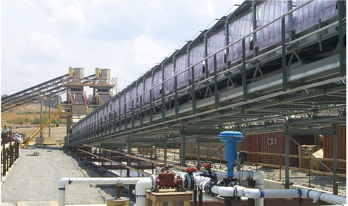
Wet belt at Saluda Dam, South Carolina
