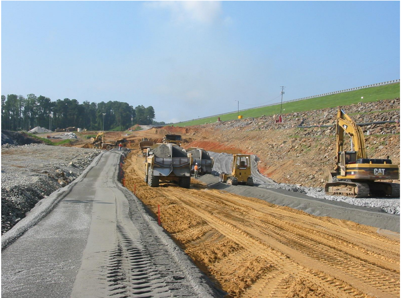
Multi-zone placement at Saluda Dam
