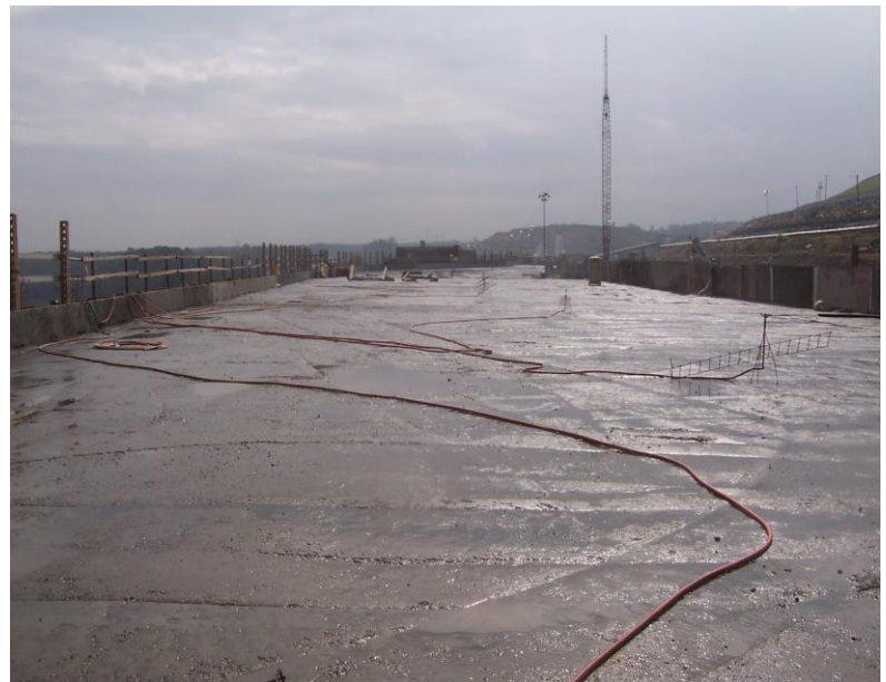
Proper curing of an RCC lift surface.
