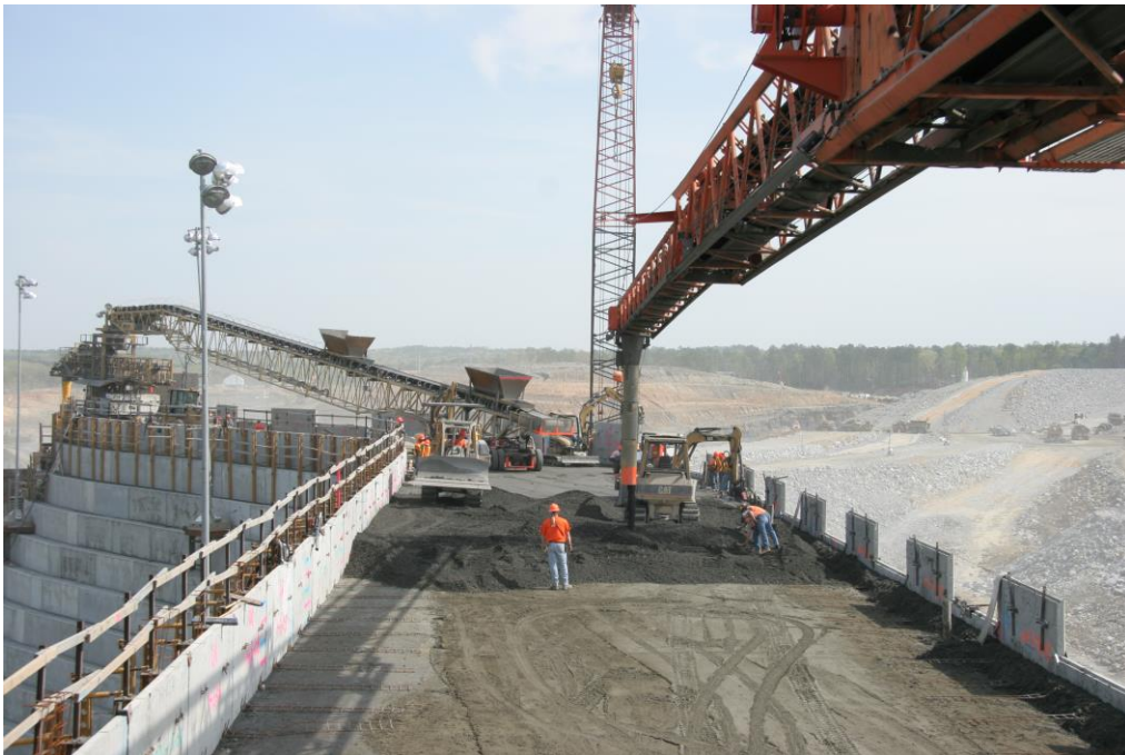
Bedding mix placement on the top lifts at Saluda Dam
