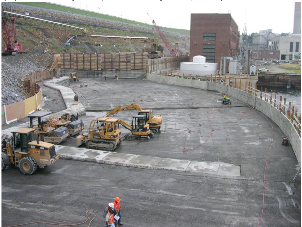
Typical joint preparation of warm joints
