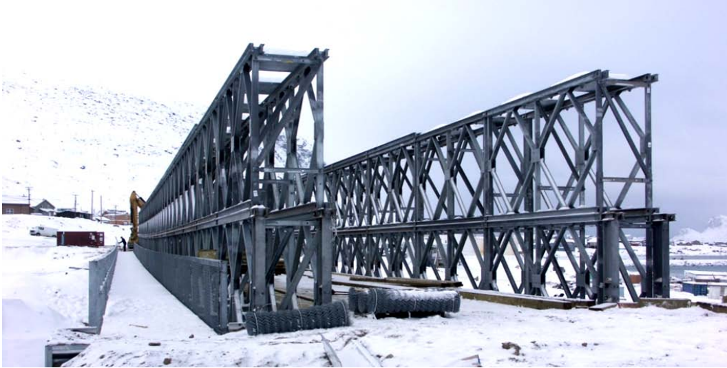
Figure 1: Spillway Bridge, Long-Sault Rapids, ON (Algonquin Bridge)
