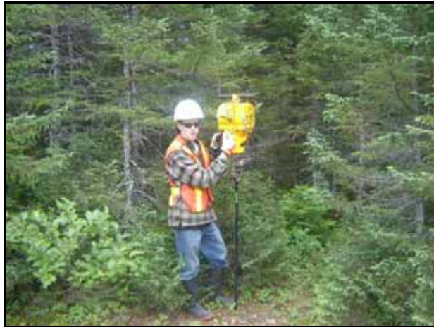
Photo 4: Probing for bedrock with a Pionjar drill and 1.8 m drill rod.
