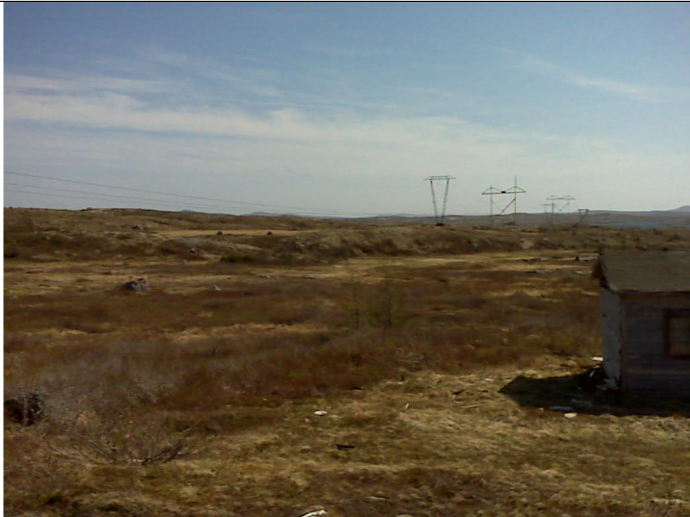
Photo 2 – View of Marshalling Yard Site E looking south.
