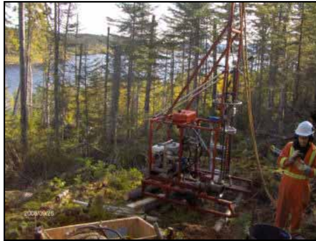
Photo 8: Drilling on the south side of the Churchill River crossing.
