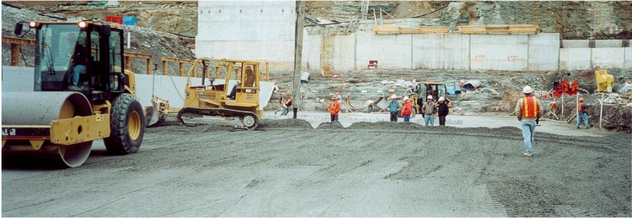
Spreading RCC with a Cat D5 dozer at North Fork Hughes River Dam. The laser detector is mounted on the blade for grade control.
