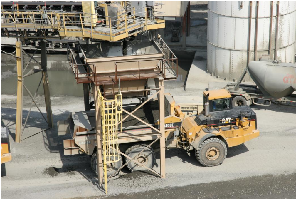
A gob hopper loads a haul truck from the RCC plant at the Saluda Dam Project
