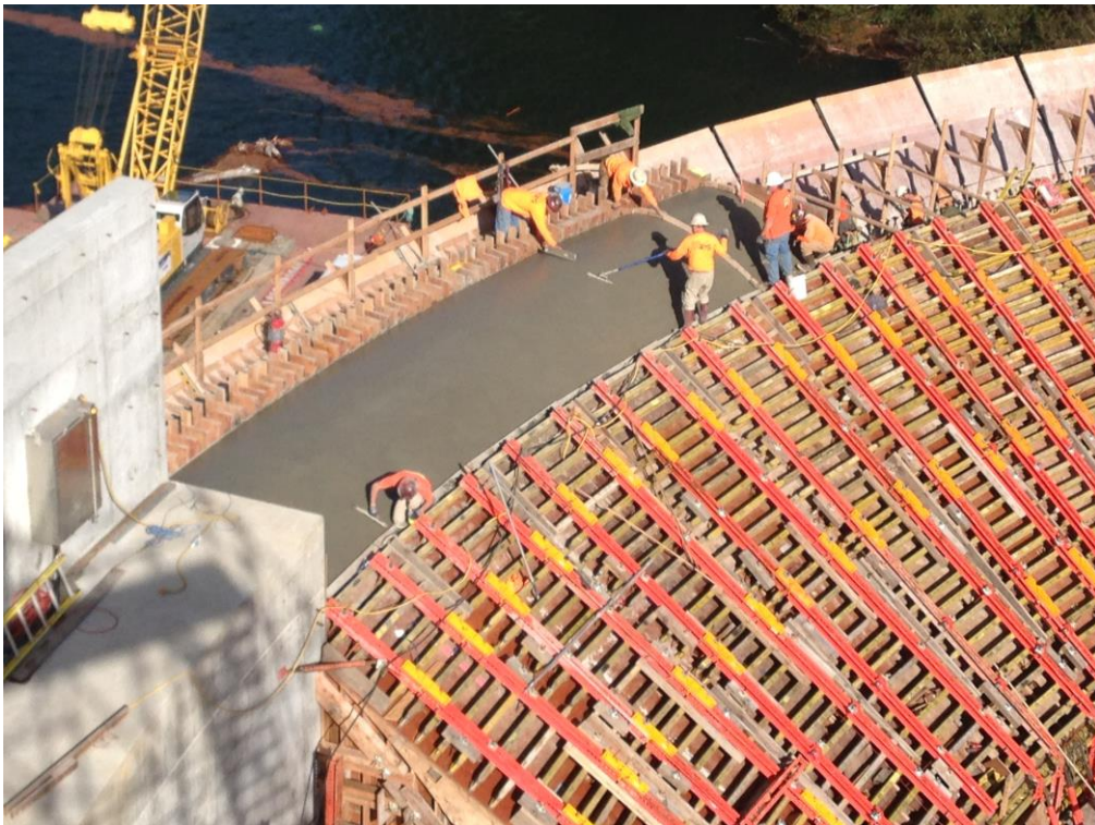
Ogee with Flip Bucket placed at the Crest of the Blue Lake Dam in Alaska, August 2014
