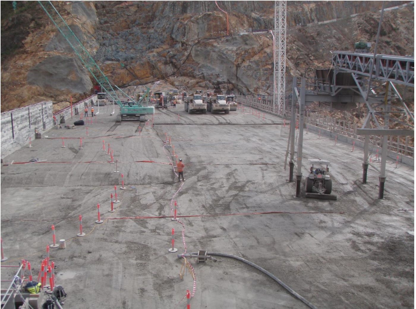
Gob Hopper on the Lift at Cotters Dam, NSW Australia
