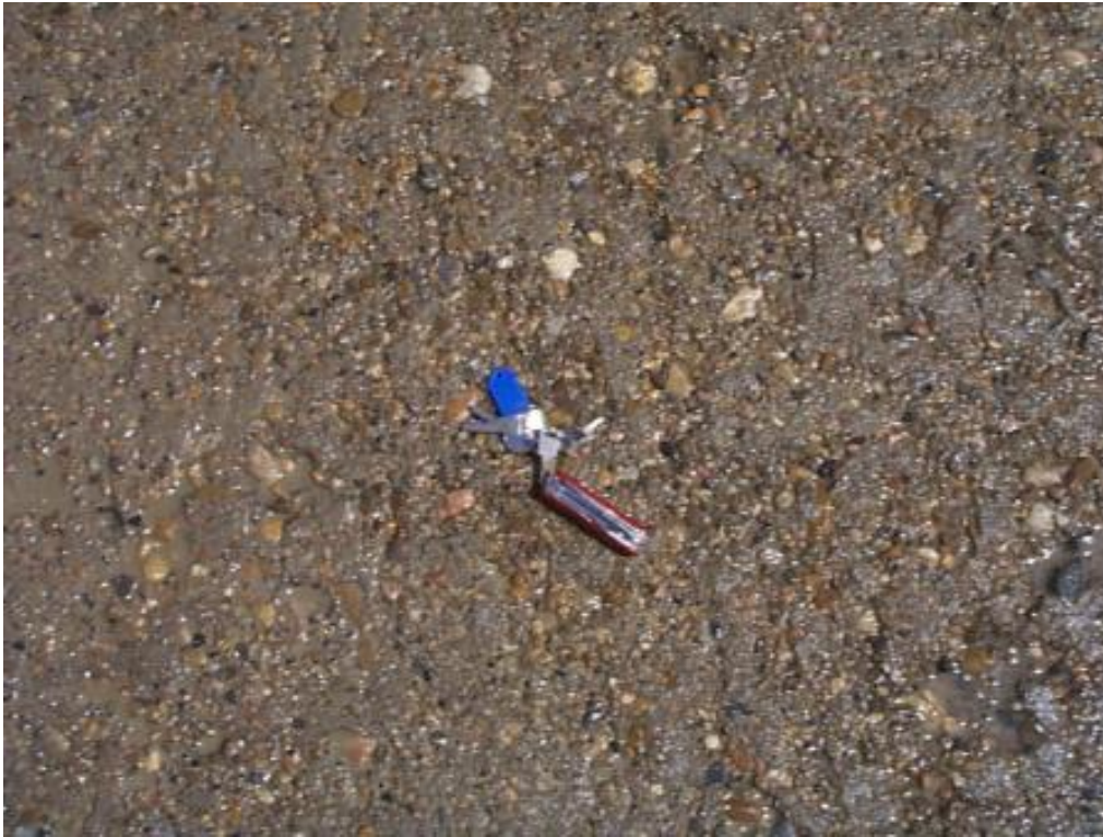
Typical surface of a treated cold joint
