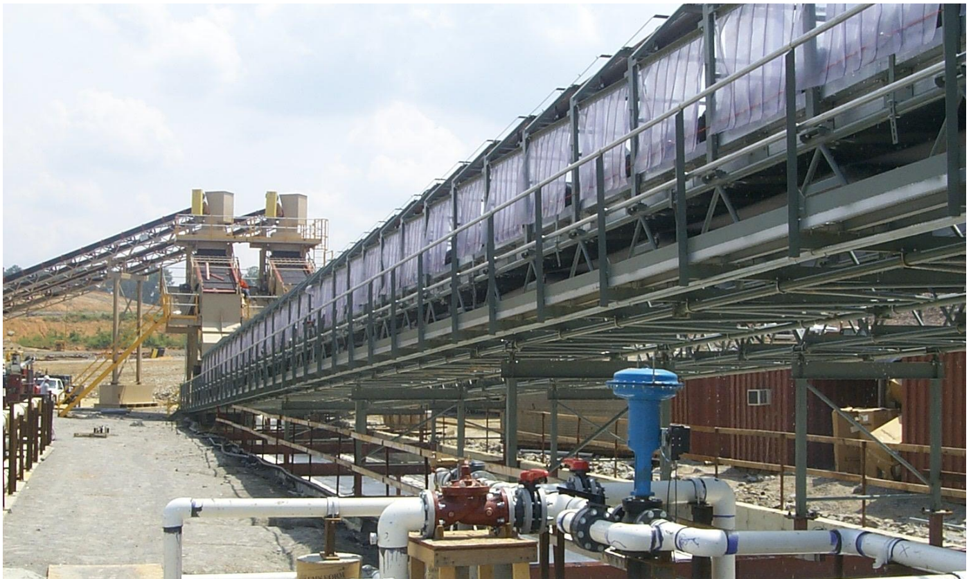
Wet belt at Saluda Dam, South Carolina
