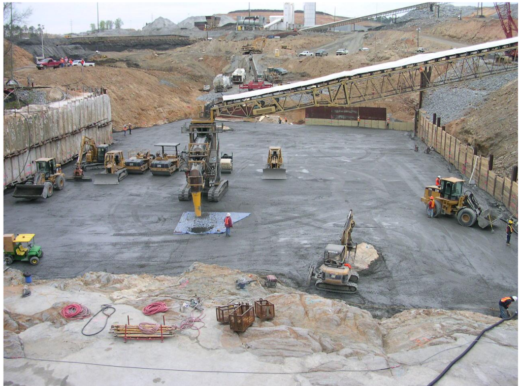
A crew uses a tarp to collect dry RCC as they prepare the lift surface for treatment
