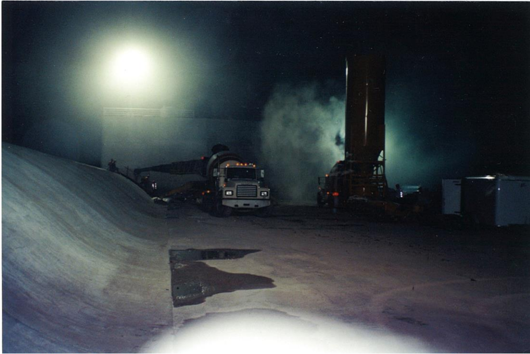
Ogee Crest placed over RCC at the North Fork Hughes River Dam
