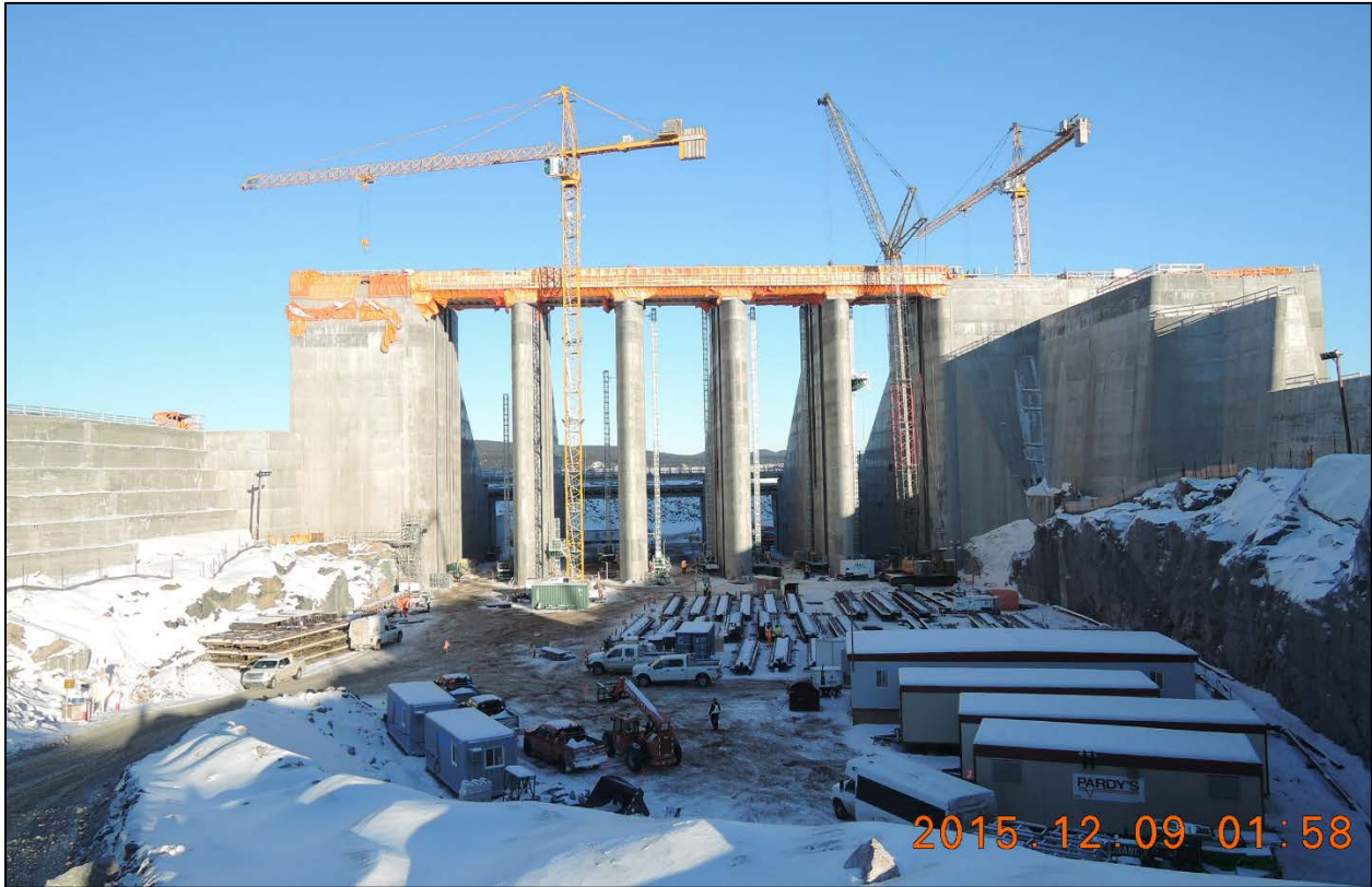
Figure 6: Civil Contractor Tower Crane Positioned in the Spillway, dated December 9, 2015
