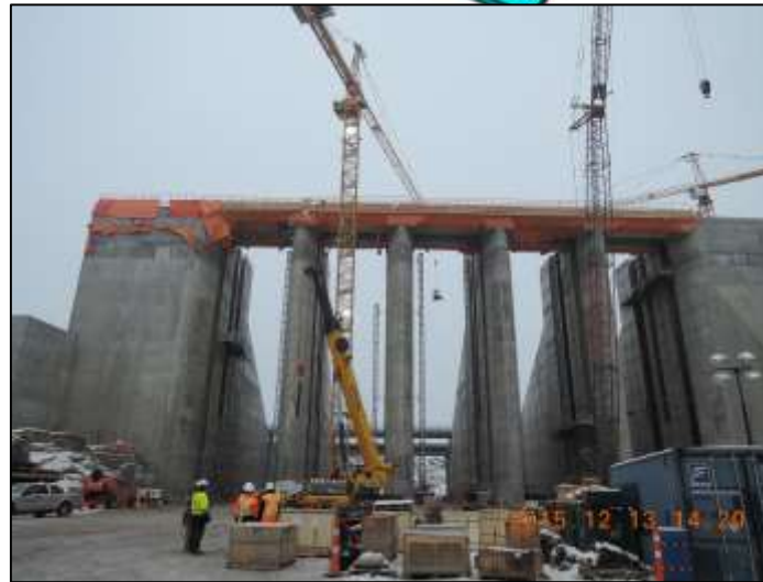
December 13 th , 2015 Civil Contractor presence continues
