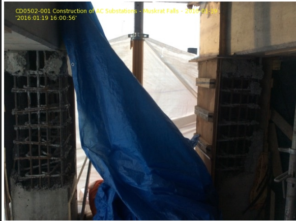
GIS Building ( Fox Construction removing formwork from the bottom of the top slab between grid lines 8 & 9 )
