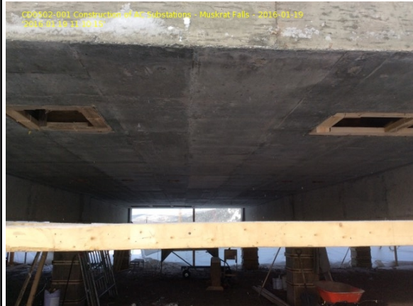
GIS Building ( Fox Construction removing formwork from the bottom of the top slab between grid lines 8 & 9 )
