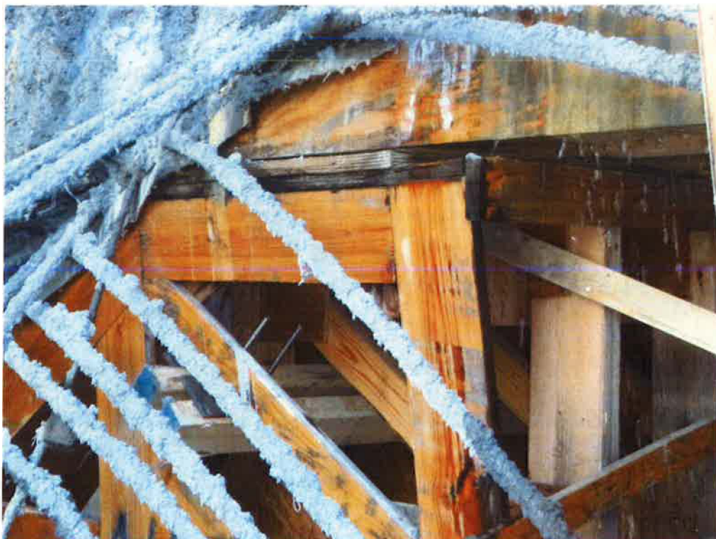
Figure 20: Timber structure of element A16
