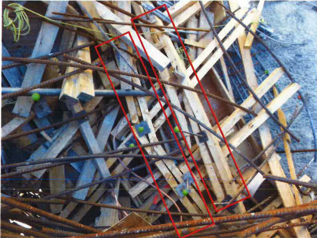
Figure 23: Whalers and ties from Built-in-place bulkhead separating D2ENB-02 and D2ENB-03
