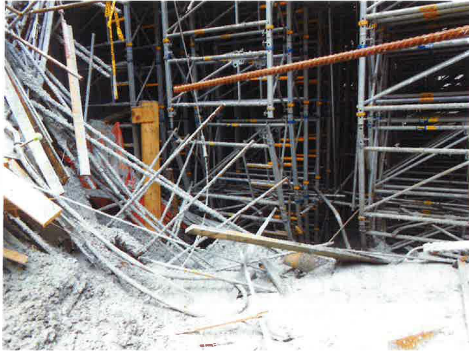
Figure 21: View of the Doka shoring towers from the Elbow
