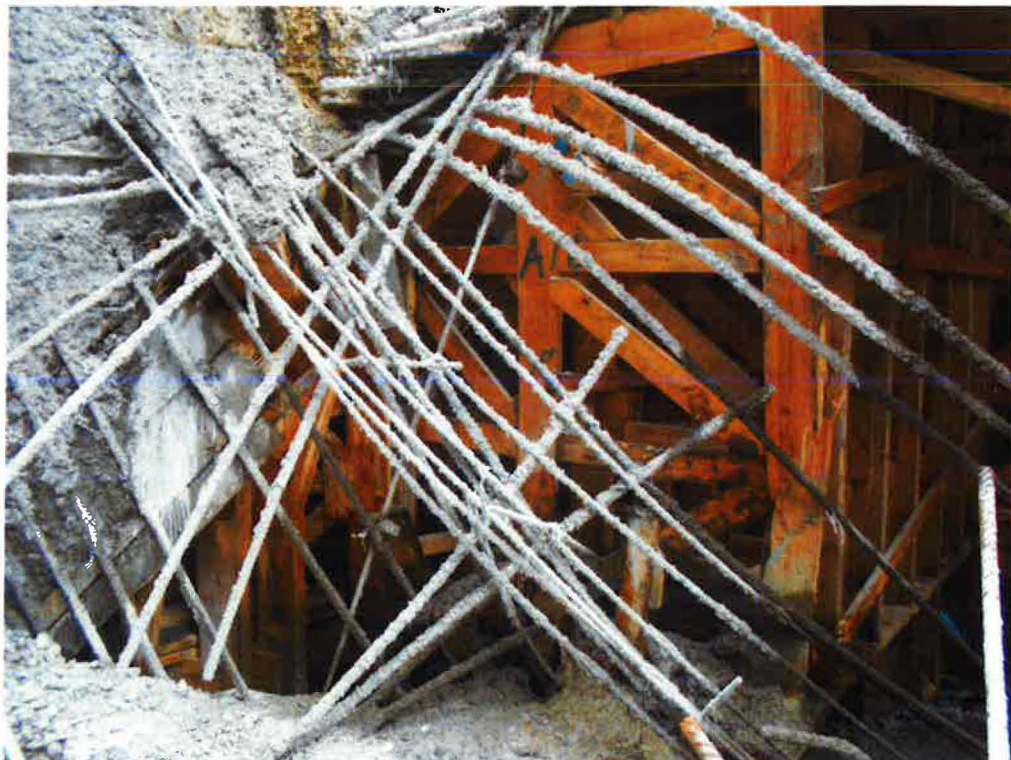
Figure 18: Timber structure of element A16
