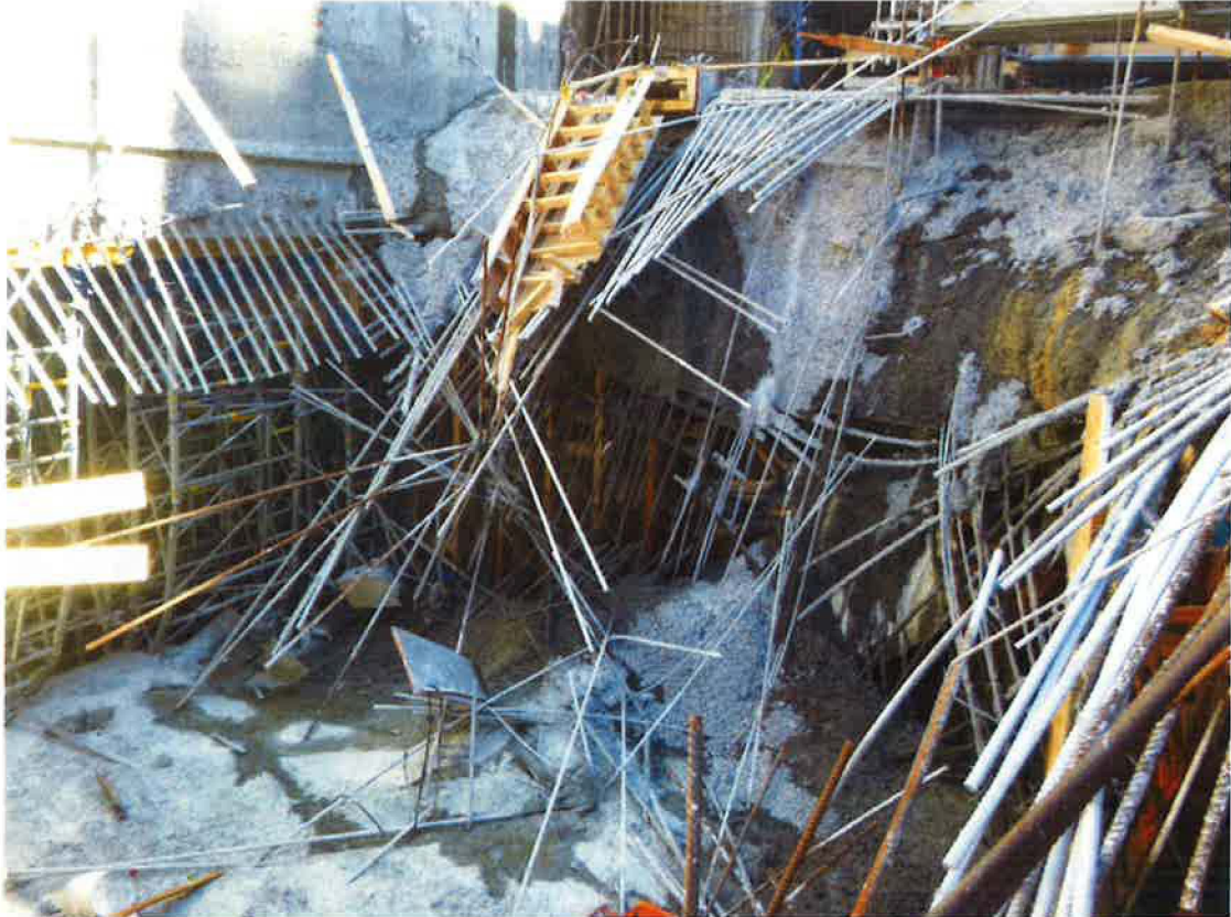
Figure 24: Suspended formwork, rebar, and concrete, looking SE
