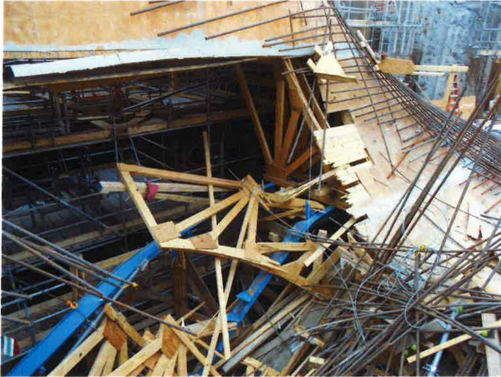
Figure 17: View of the North portion of Panel A29
