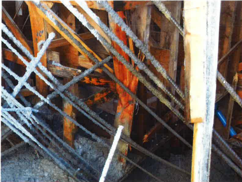
Figure 19: Timber structure of element A16
