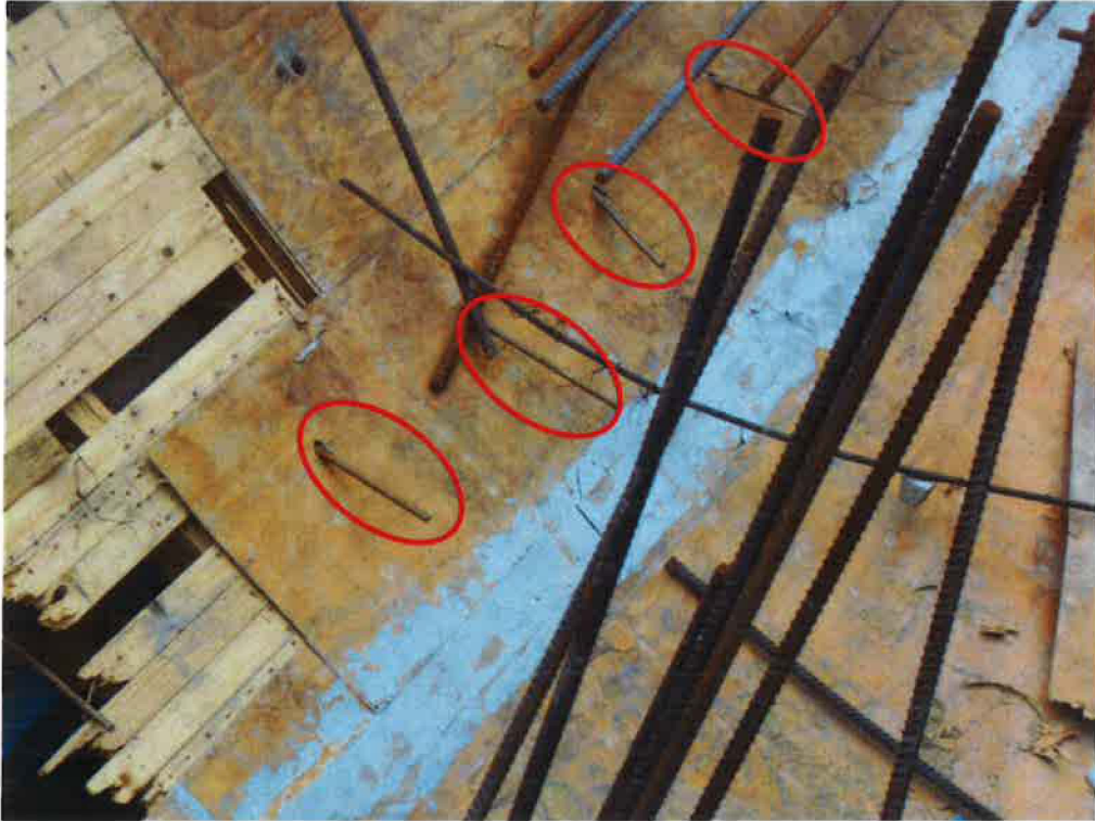
Figure 13: Ties penetrating the formwork (for upcoming pour D2ENB-03)
