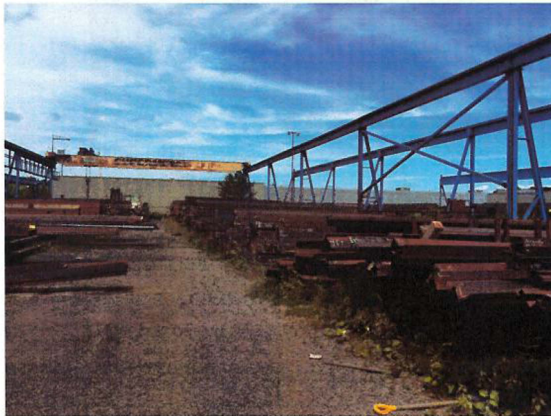
Figure 12 - Outside Steel Storage
