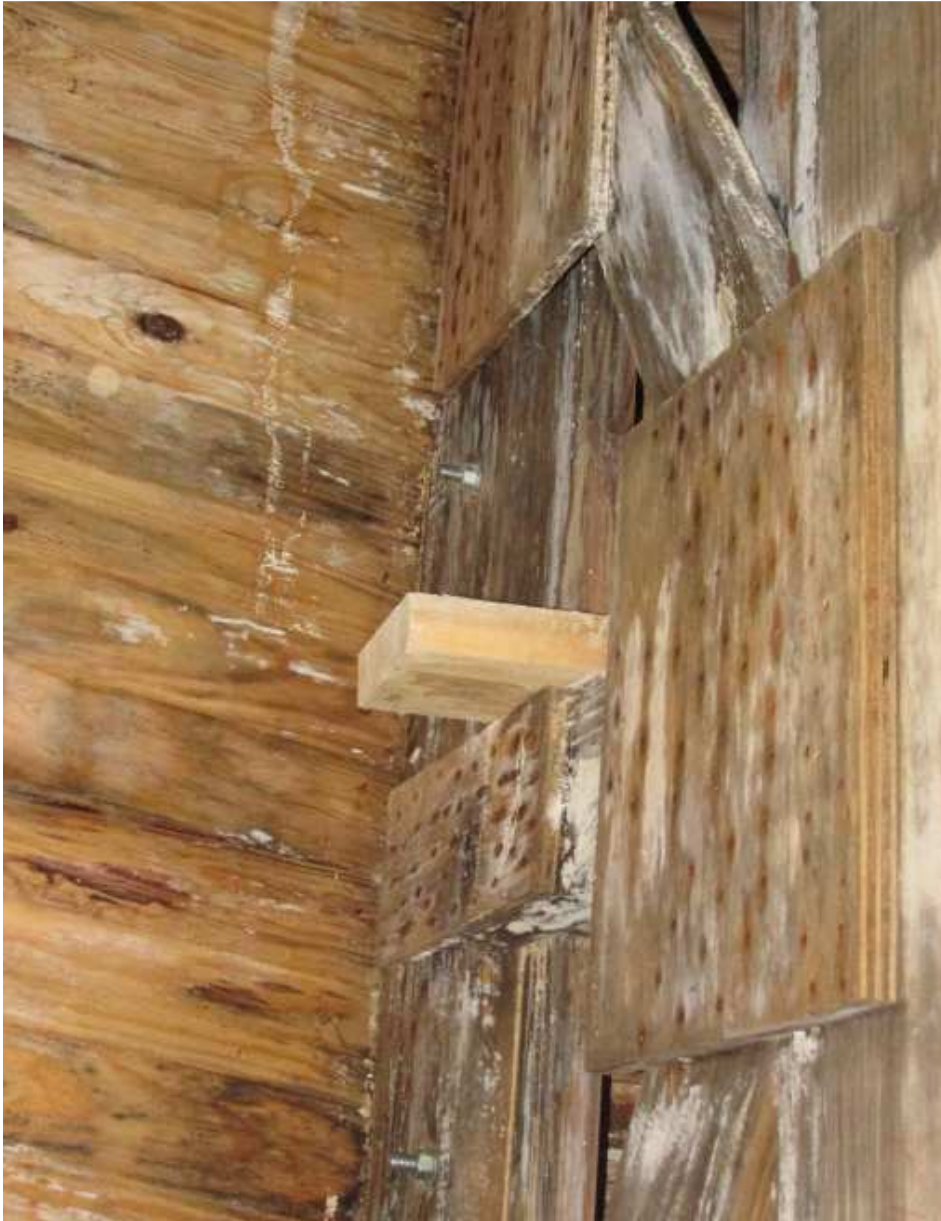
Figure 20: Weathered formwork
