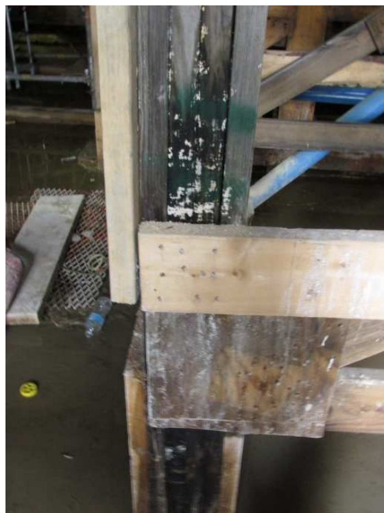
Figure 17: Shoring towers for Draft Tube 3 (green paint) found in Draft Tube 1
