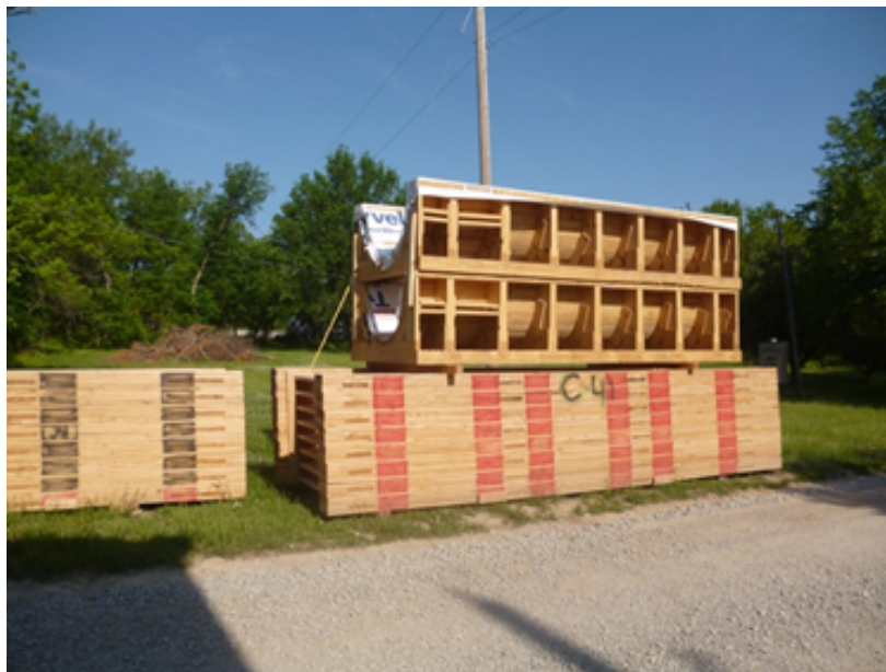
Figure 62: May 15, 2014. Formwork and falsework at CEI facility. Note fresh, unweathered wood.
