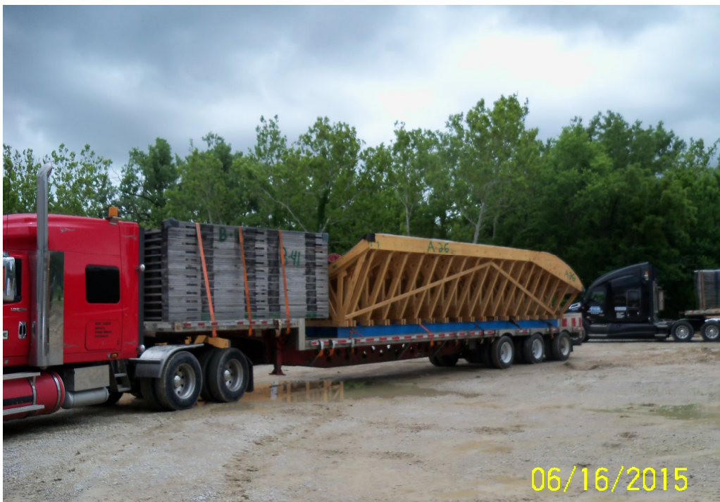
Figure 66: June 16, 2015 DT1 formwork and falsework at CEI yard in Kansas. Note weathering of tower legs relative to formwork module A26.
