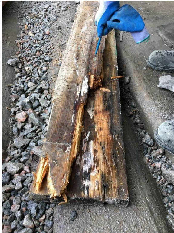
Figure 38: Bottom of Tower Leg obtained from DT2, Tower C3
