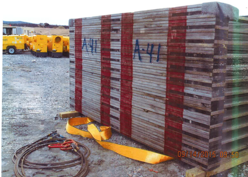
Figure 67: September 14, 2015. DT2 Falsework offloaded on site and stored at C1 laydown
