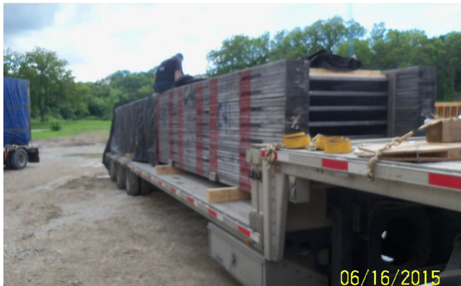
Figure 64: June 16, 2015 at CEI yard. Right hand view of falsework towers believed to have been installed in DT2.
