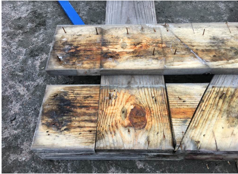
Figure 42: Disassembled Leg at Bracing from DT3
