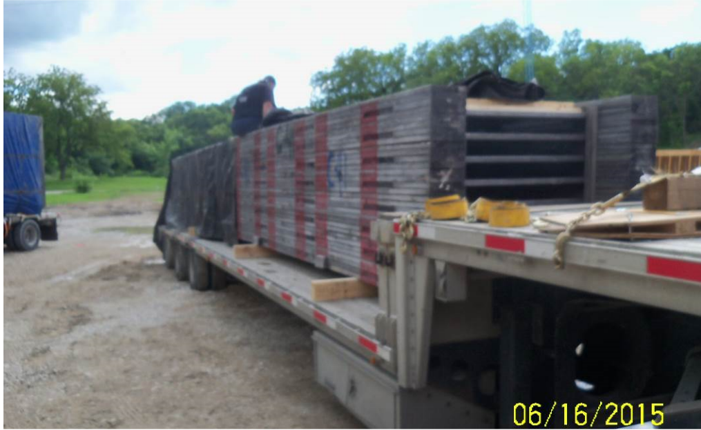
Figure 3: June 16, 2015 at CEI yard (more than one year after fabrication). Right hand view of falsework towers believed to have been installed in DT2.
