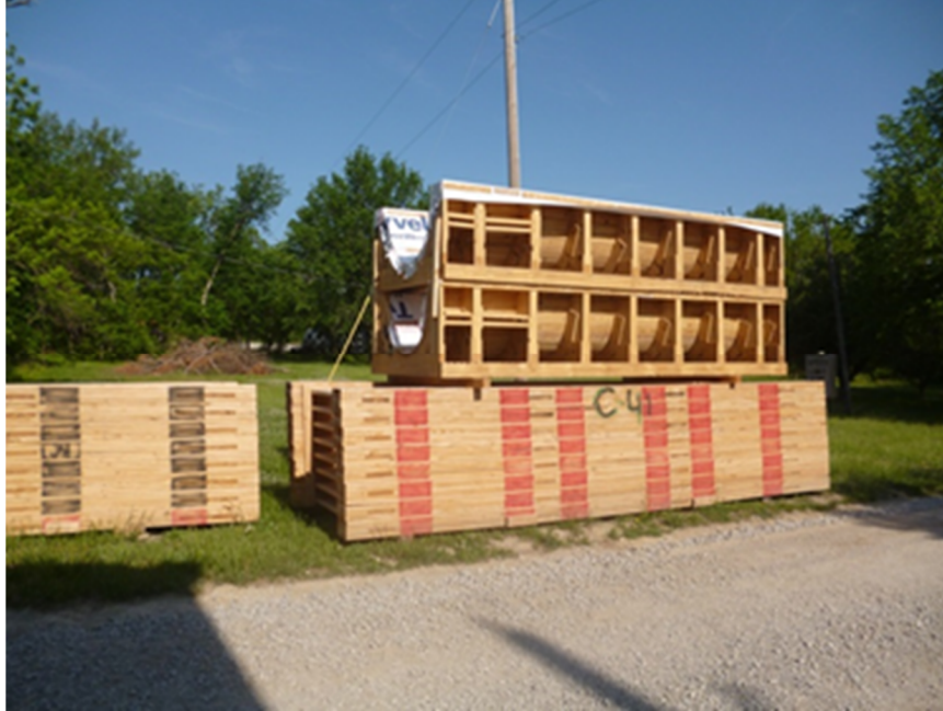
Figure 1: May 15, 2014. Formwork and falsework at CEI facility. Note fresh, unweathered wood.
