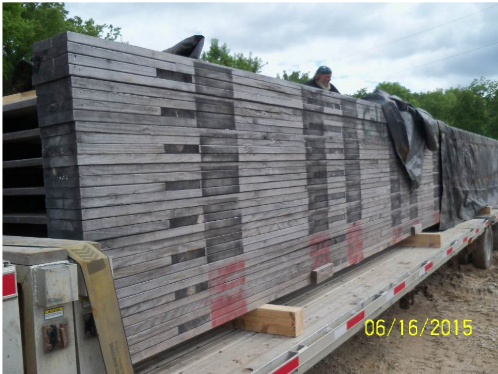
Figure 4: June 16, 2015 at CEI yard (more than one year after fabrication). Left hand view of falsework towers believed to be installed in DT2
