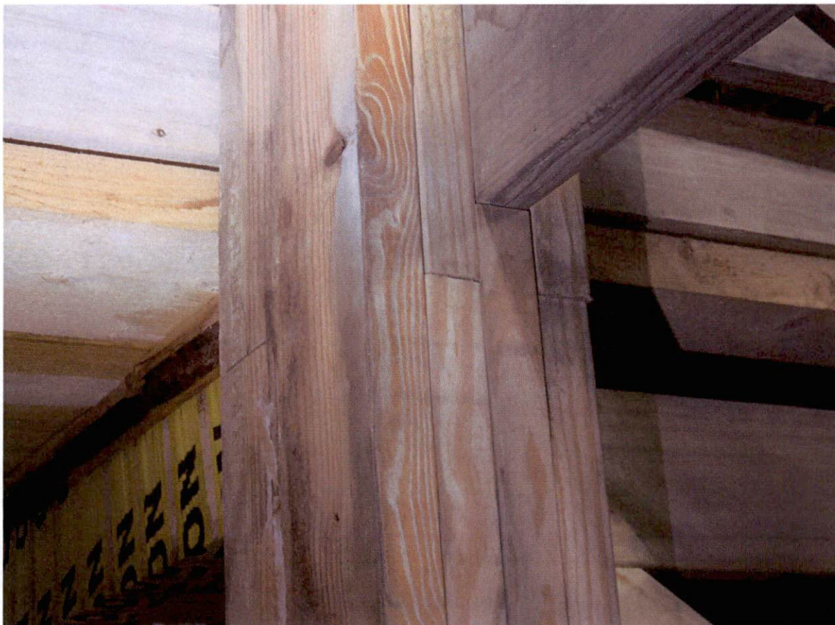
Unit 4 - Inappropriate location for built-up column joint
