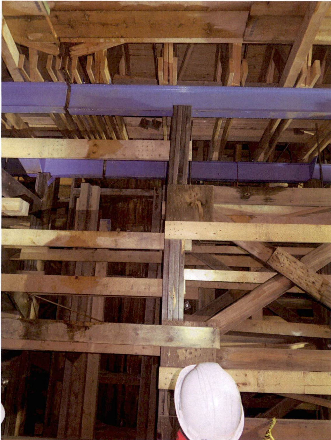
Unit 1 - Tower B3, buckling at top of post
