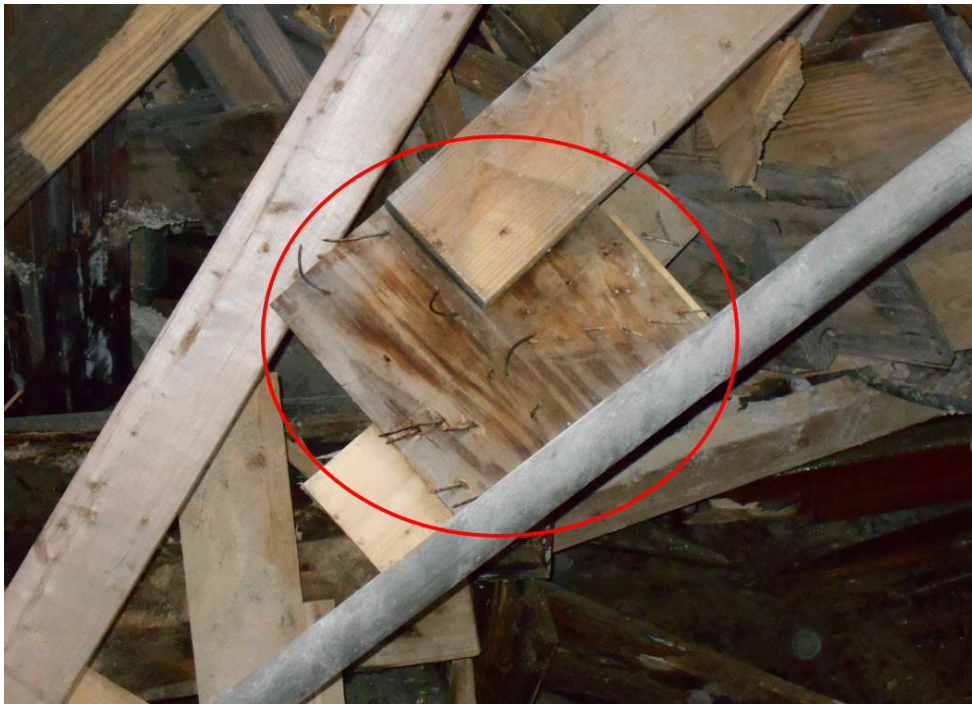
Figure 26: Splice plate pulled away from tower leg
