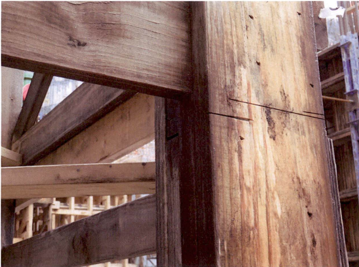
Unit 3 - Saw cut mark in lumber
