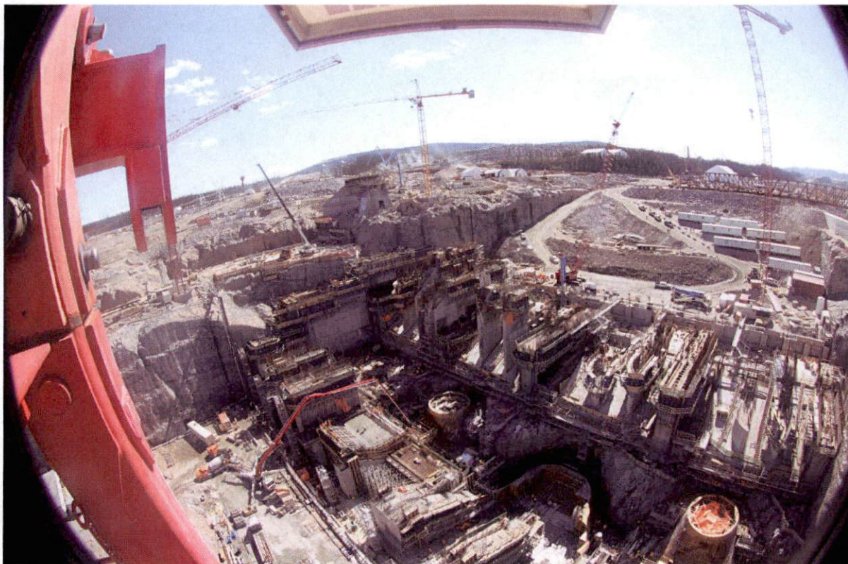
Muskrat Falls Powerhouse – Four Draft Tubes
