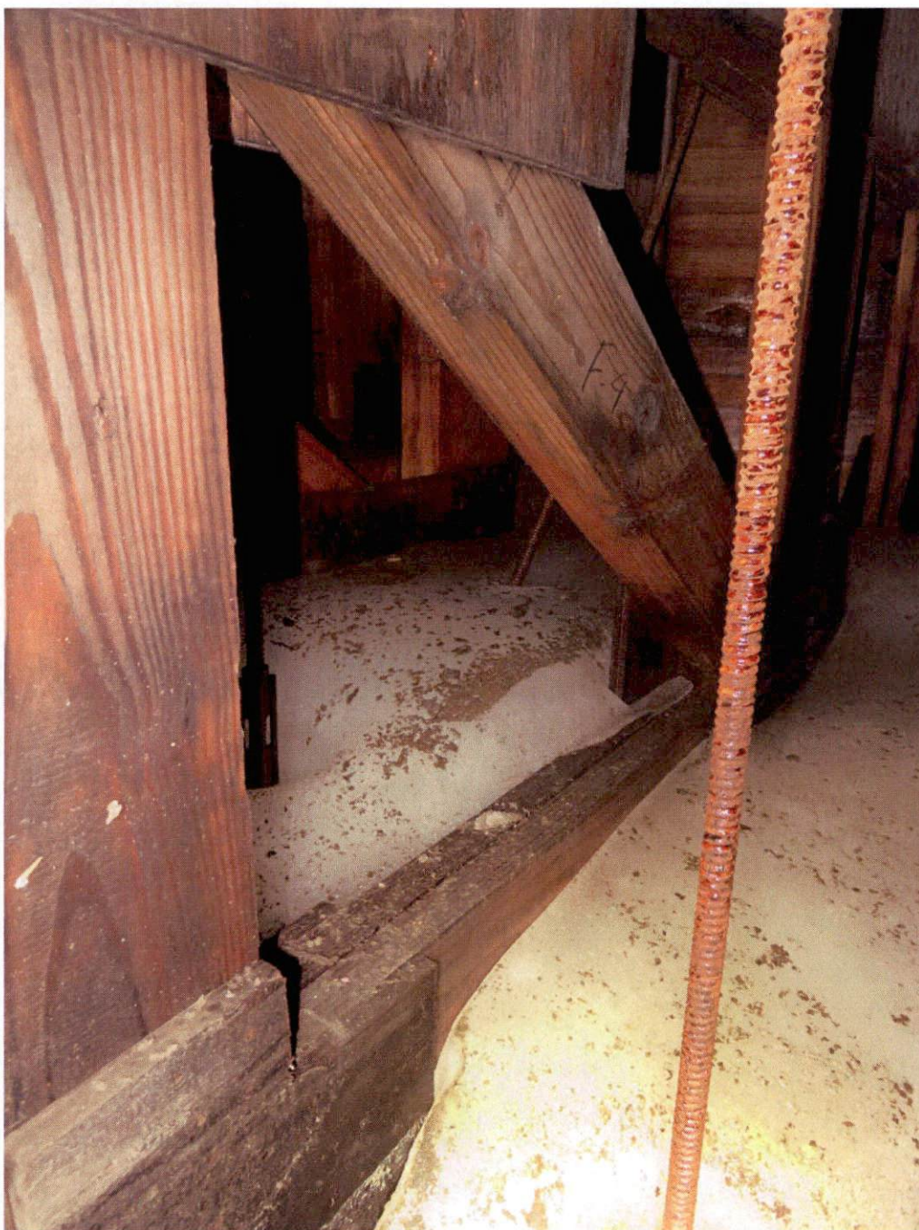
Unit 1 - Ice built up within ribs of panels A9
