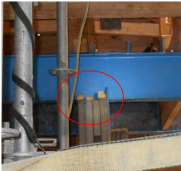
Figure 27: Inadequate shimming on top of falsework towers. No bearing plate installed
