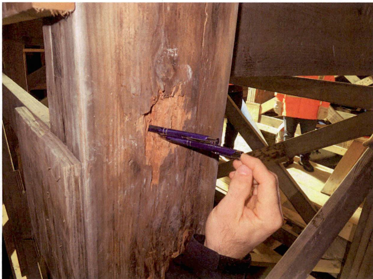
Unit 1 - Dry rot on shoring tower
