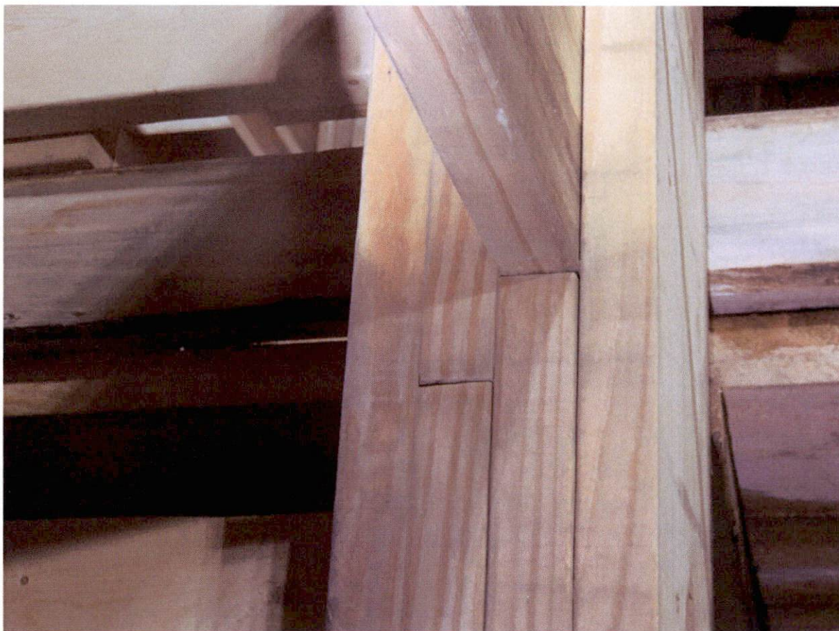
Unit 4 - Inappropriate location for built-up post joint
