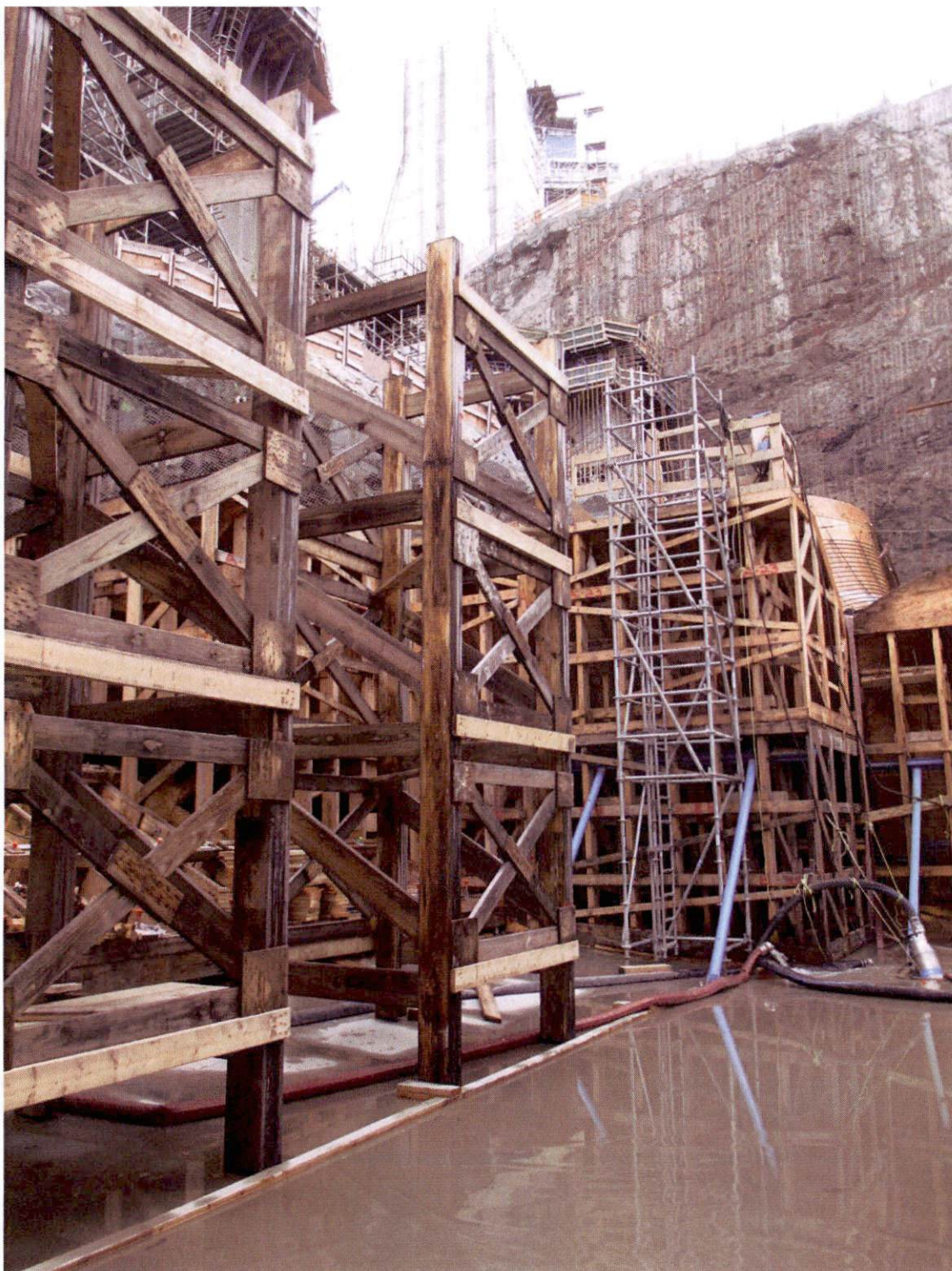
Unit 3 - Installed shoring tower weathering
