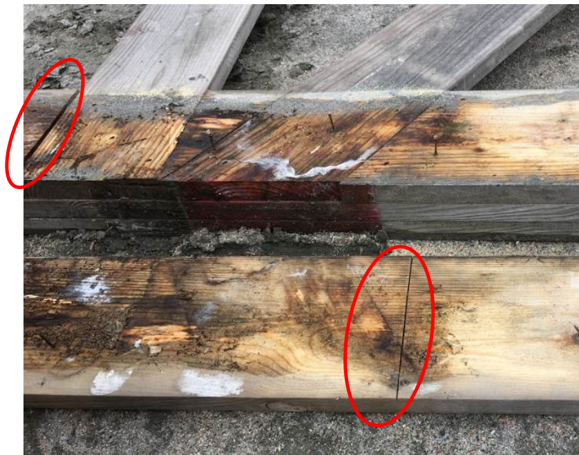
Figure 43: Gaps in Tower Leg Butt Joints (left) and saw kerfs (right) from DT3
