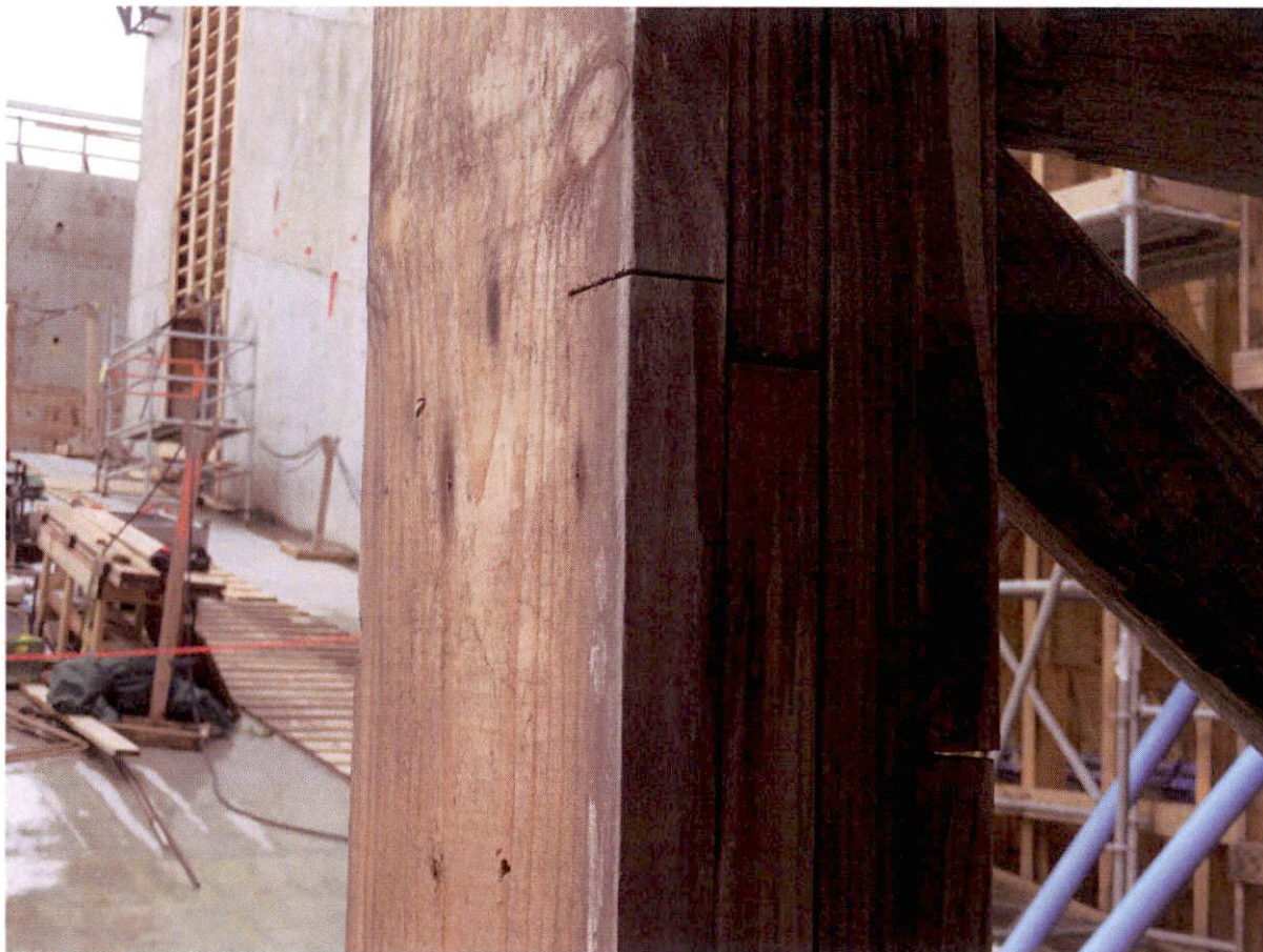
Unit 3 - Saw cut mark in lumber
