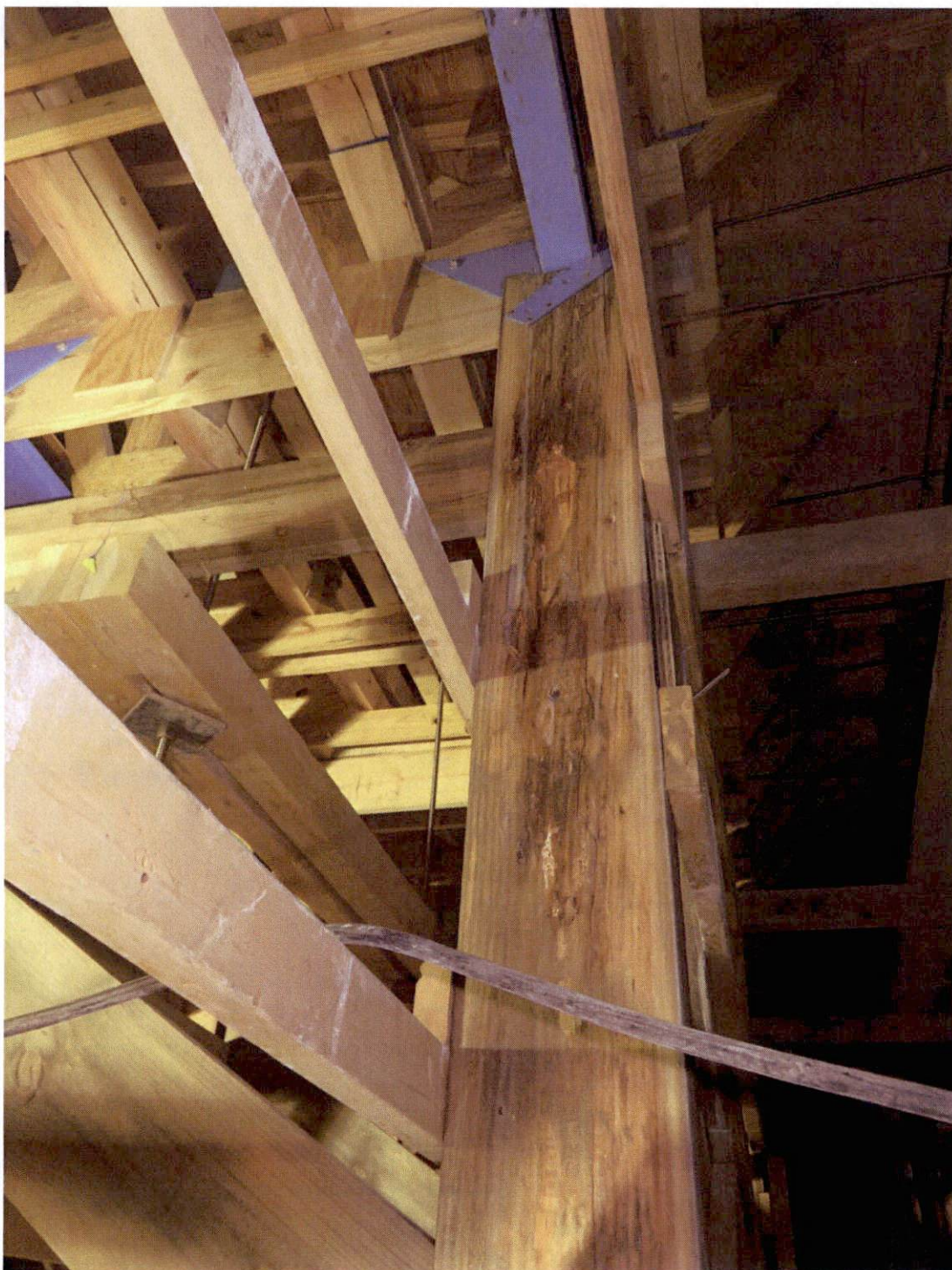
Unit 1 - Decayed wood on tower B2
