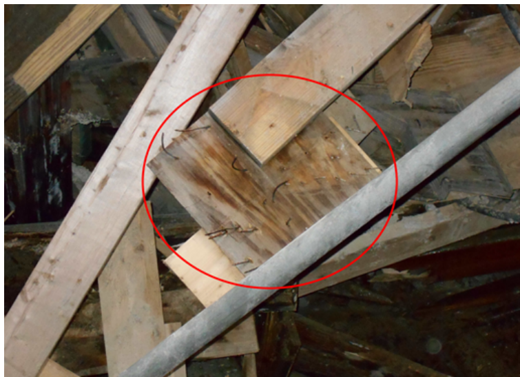
Figure 54: Inadequate nailing of splice plate in DT2
