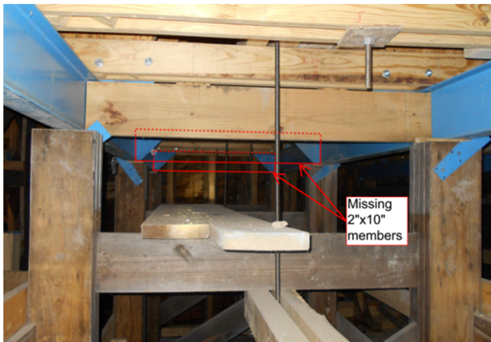
Figure 57: Missing members between beams. DT3 tower B1
