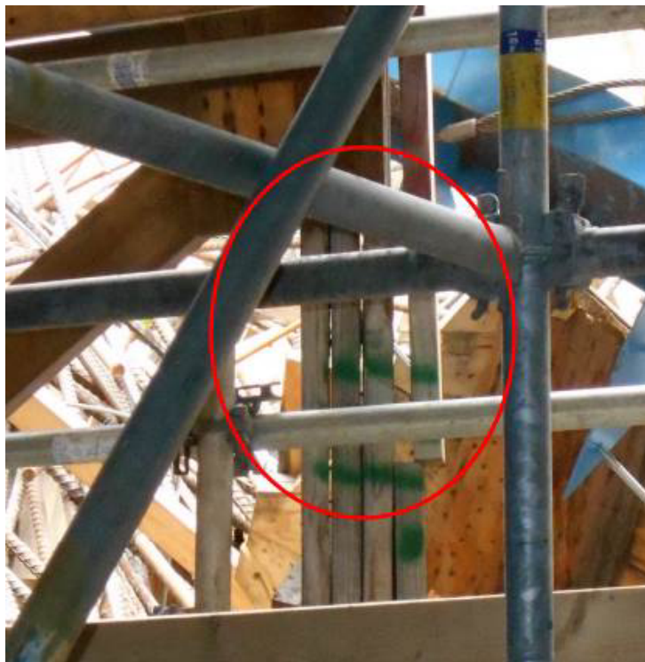
Figure 19: Built-up column members separating due inadequate joining
