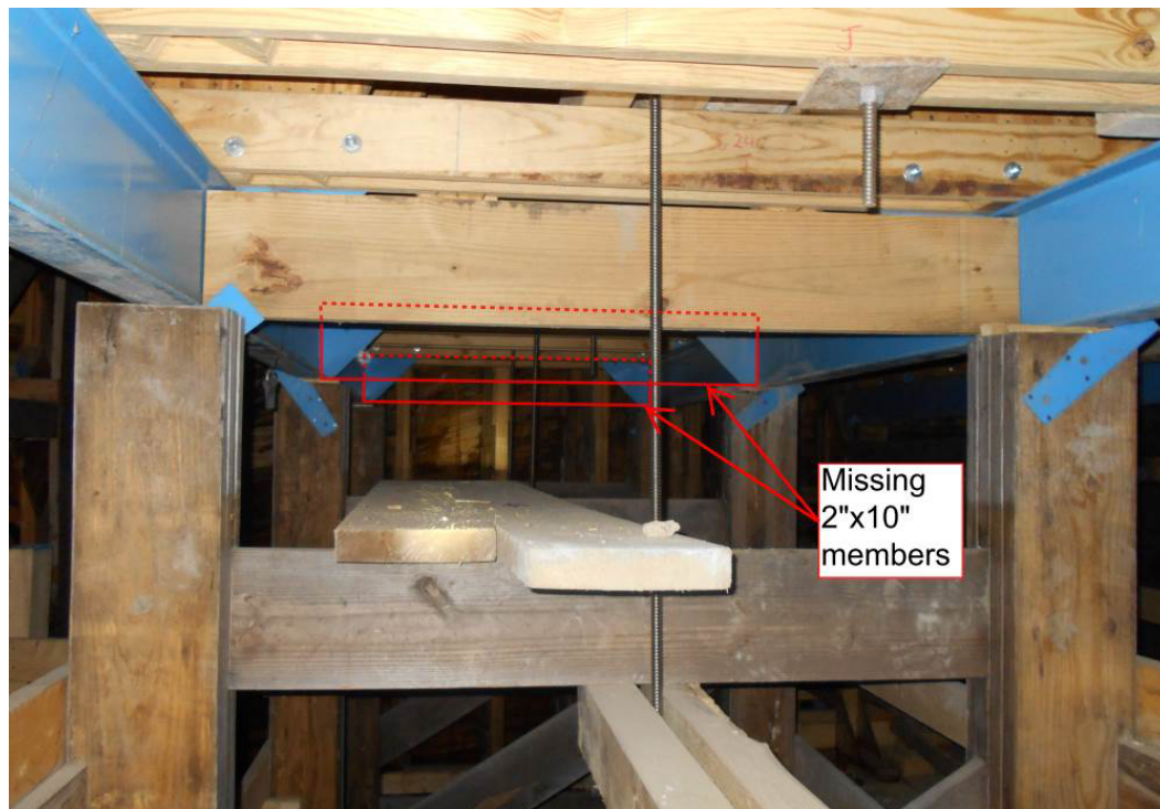
Figure 20: Missing members between steel beams above Tower B1
