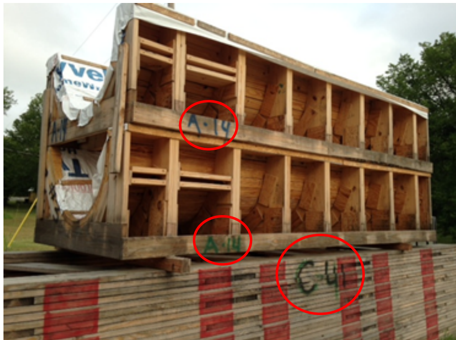
Figure 22: Formwork and falsework with multiple color markings "C41" and "A14" at CEI's facility
