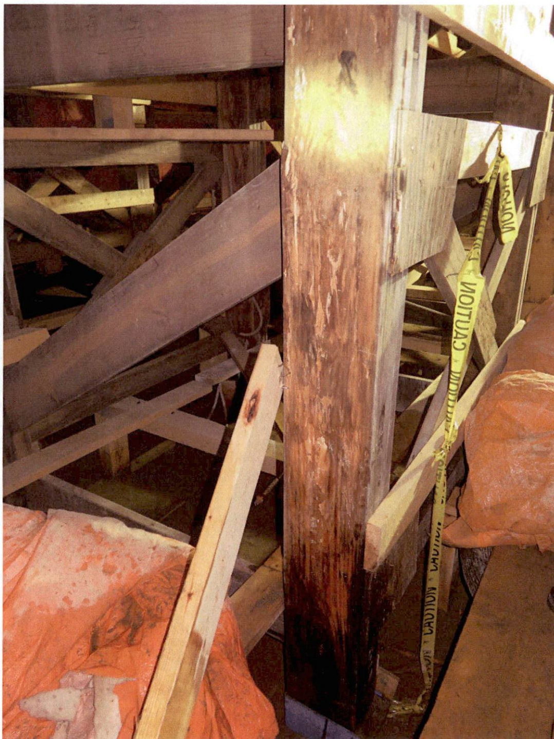
Unit 1 - Decayed wood on tower B3
