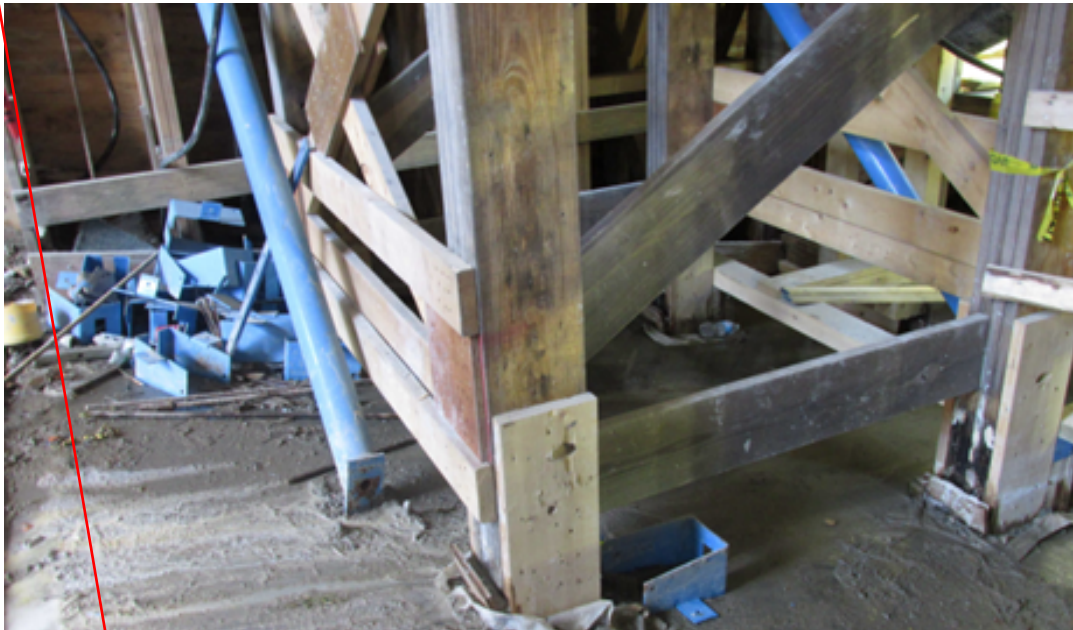
Figure 60: DT1: Uninstalled tower base anchors (blue steel clips) in foreground and piled in background. Alternate grout pad with form installed in foreground left and right.
