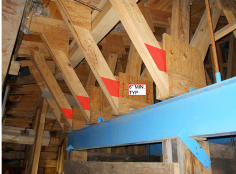
Figure 58: Inadequate splice plate size DT2
