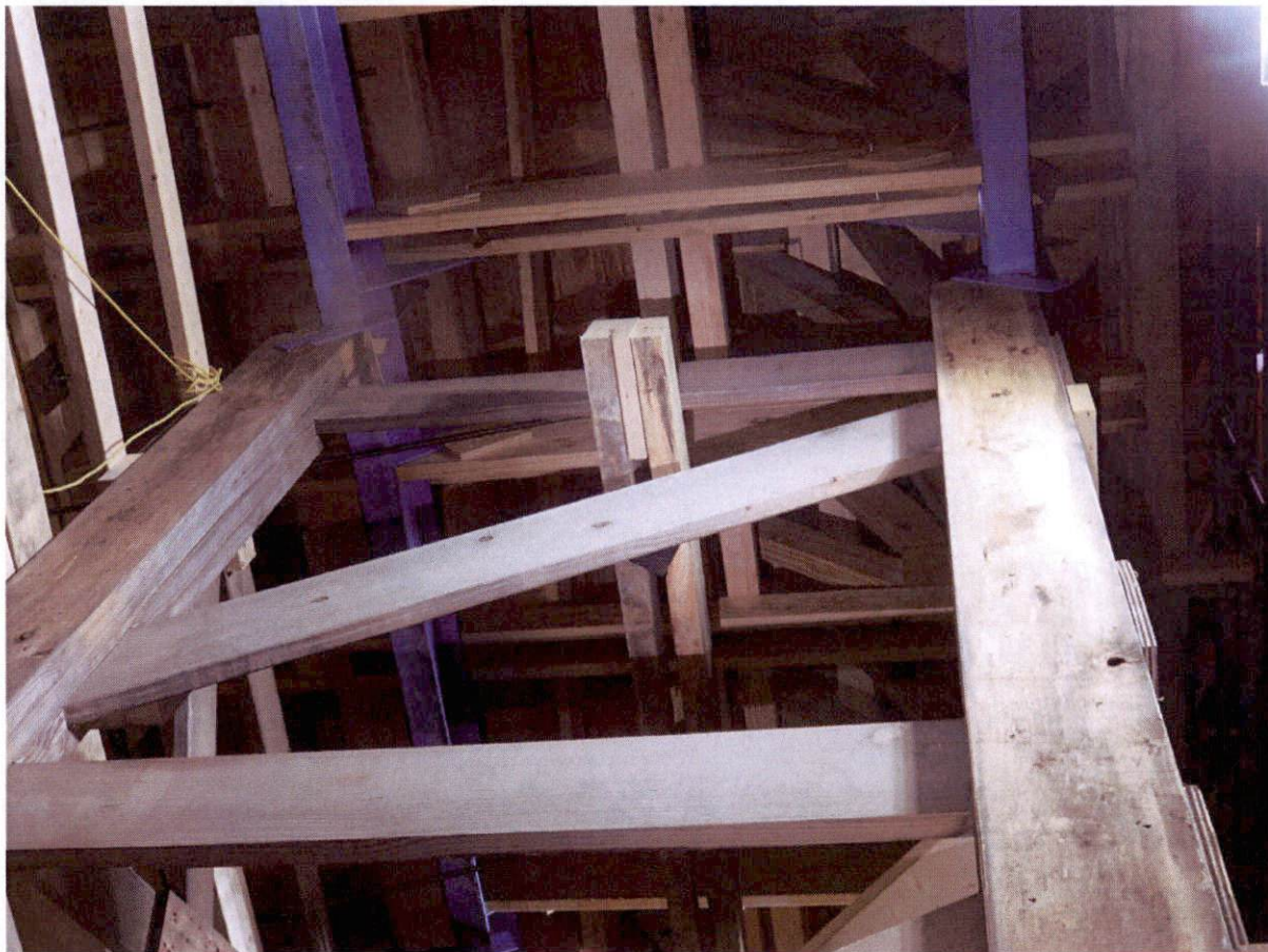
Unit 4 - Tower misaligned with steel beam
