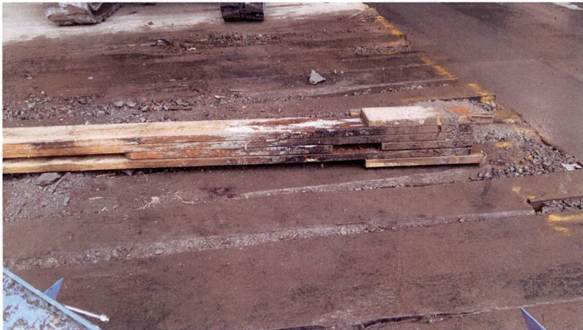
Unit 2 - Shoring Tower weathering
