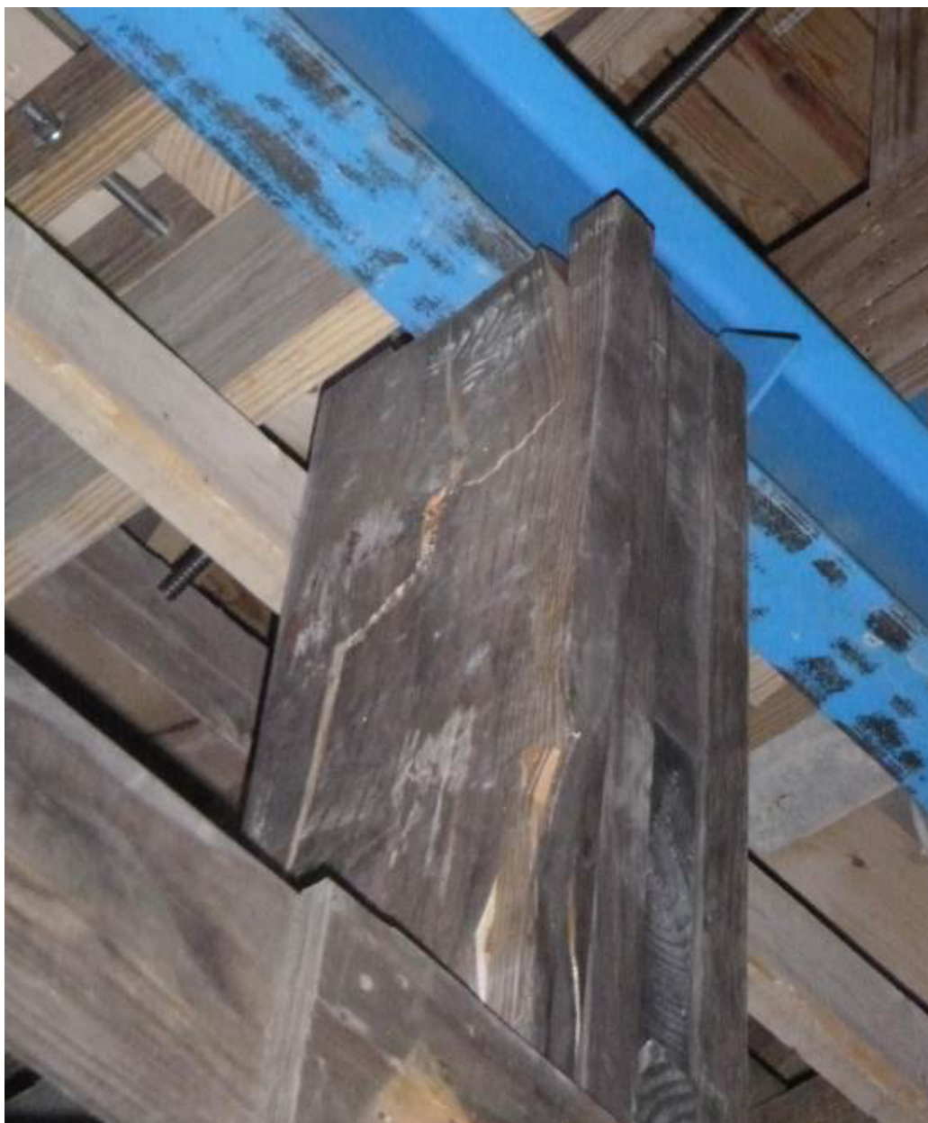
Figure 52: Local failure of tower leg at beam interface and bracing penetration in DT1
